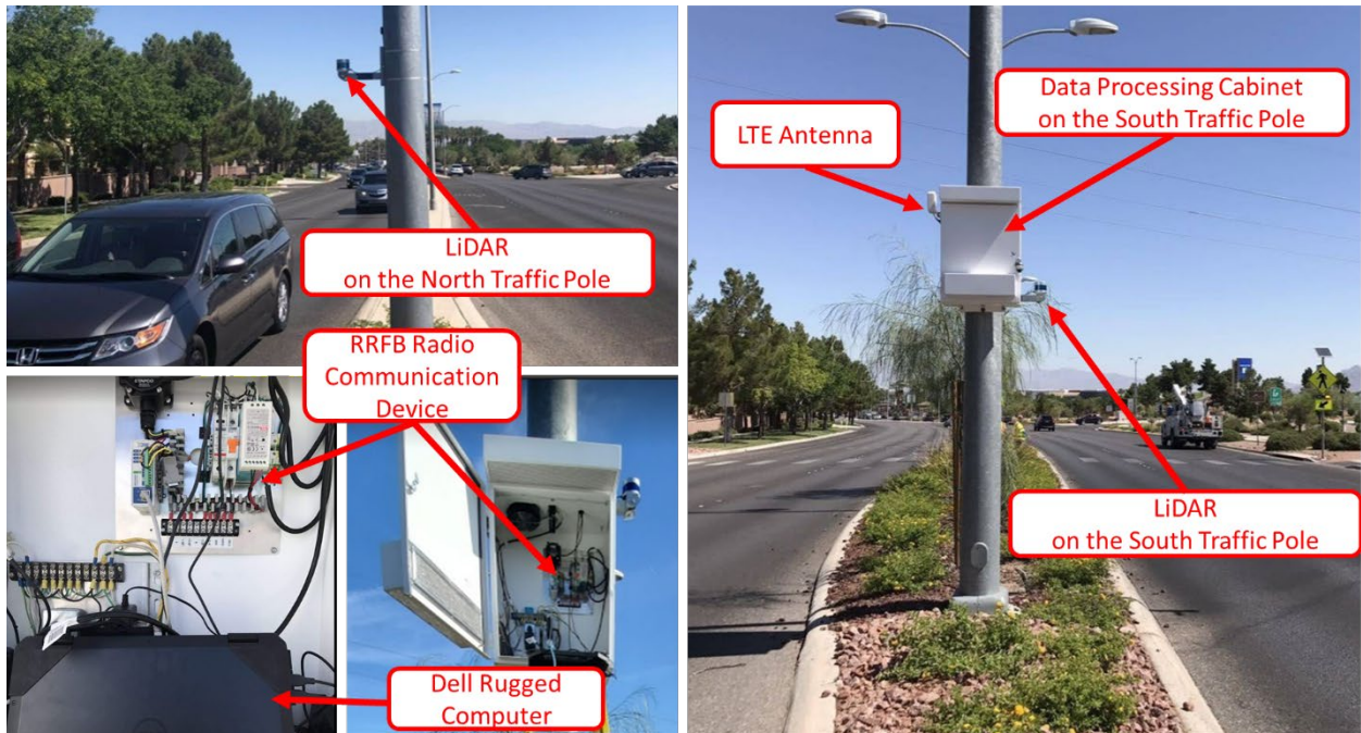
Figure 9-3 Locations of LiDAR sensors and LiDAR processing cabinet at Green Valley Pkwy and Amargosa Trail
