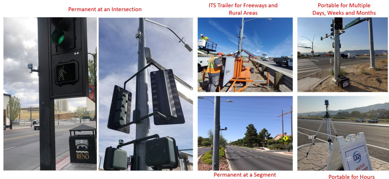
Figure 2-2 Demonstration of different roadside LiDAR sensing deployment
