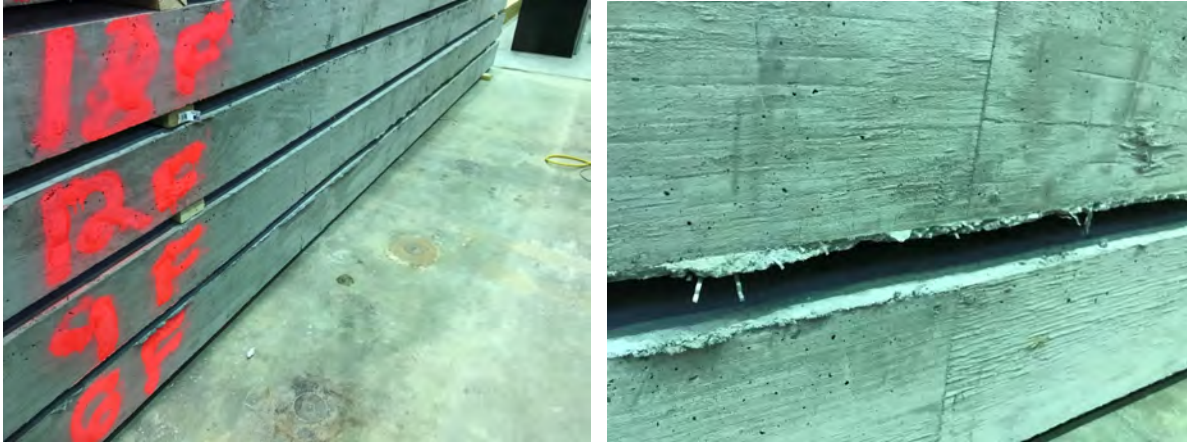
Figure 6.13 FRC slab final product
