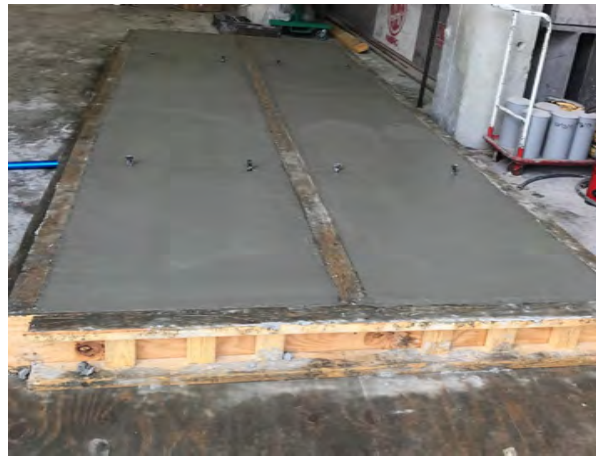
Finished slabs with inserts
