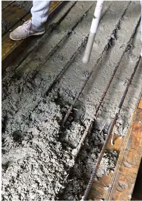
Figure 6.11 Impact of vibration on FRC workability
