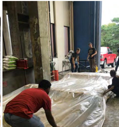
Burlap and plastic wrap for curing
