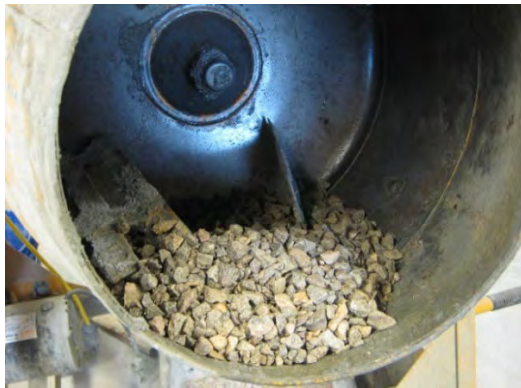
Loading coarse aggregate
