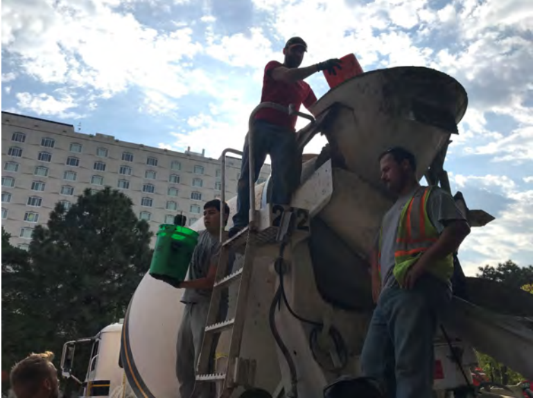
Figure 6.9 Introducing fiber into mixing truck
