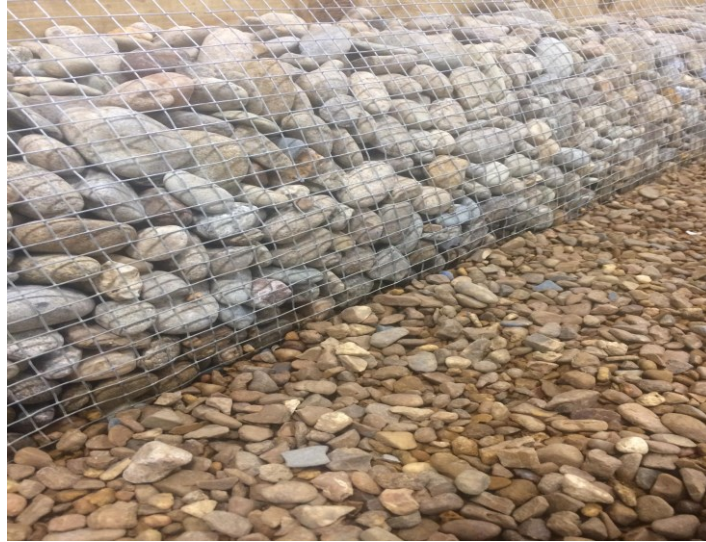
Figure 3.15. Gravel revetment with wire mesh support.
