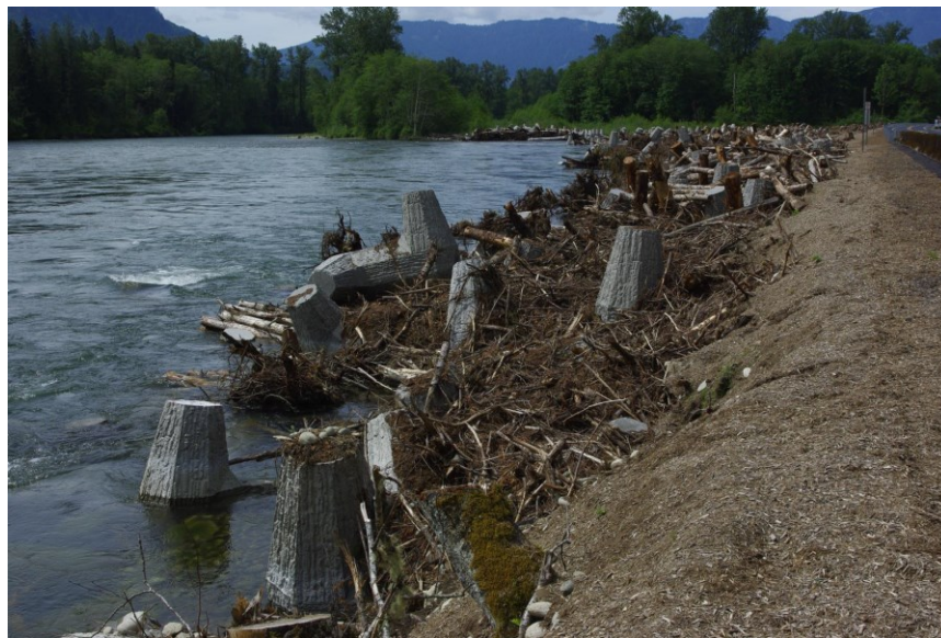
Figure 1.2. Dolotimber ELJ revetment with inclusion of logs and other LWM (WSDOT, 2011).
