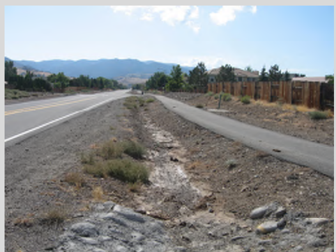
Roadside ditch along south side of Toll Road (looking west)
