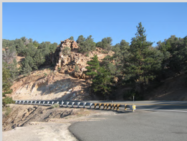
Slopes and vegetative cover along Geiger Grade Road
