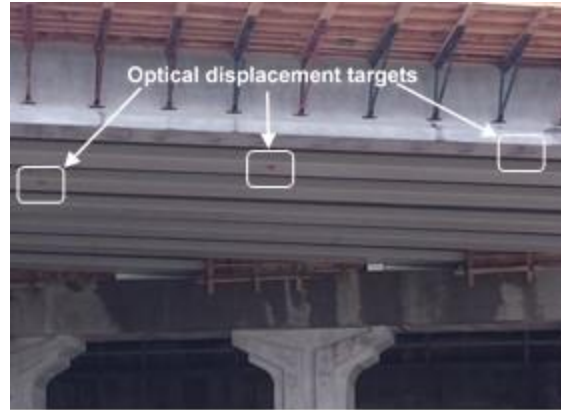
Figure 4.8. Optical displacement targets on girders of bridge central span.
