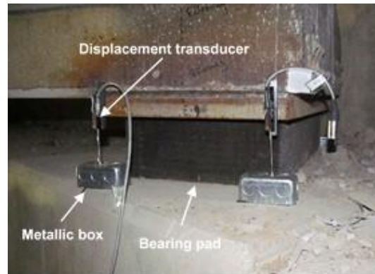
Figure 4.7. Displacement transducers installed on west abutment expansion bearing.
