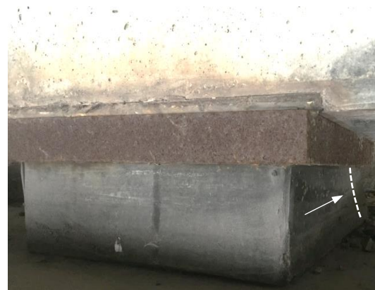
Figure 2.6. Bearing rotation at the obtuse corner. [1]
