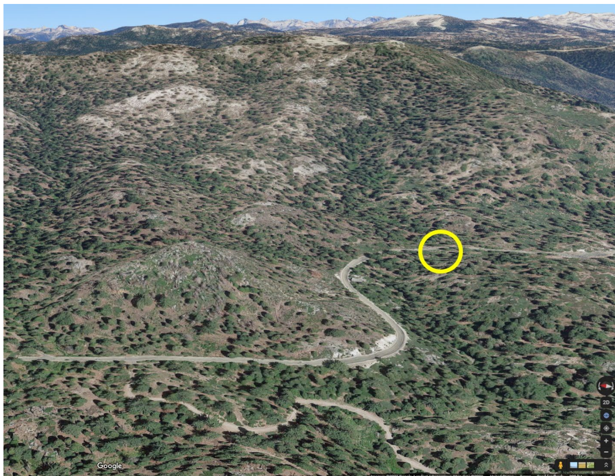
Figure 21. 3D visualization of Culvert at Wye area (looking eastward) (Google 2021).
