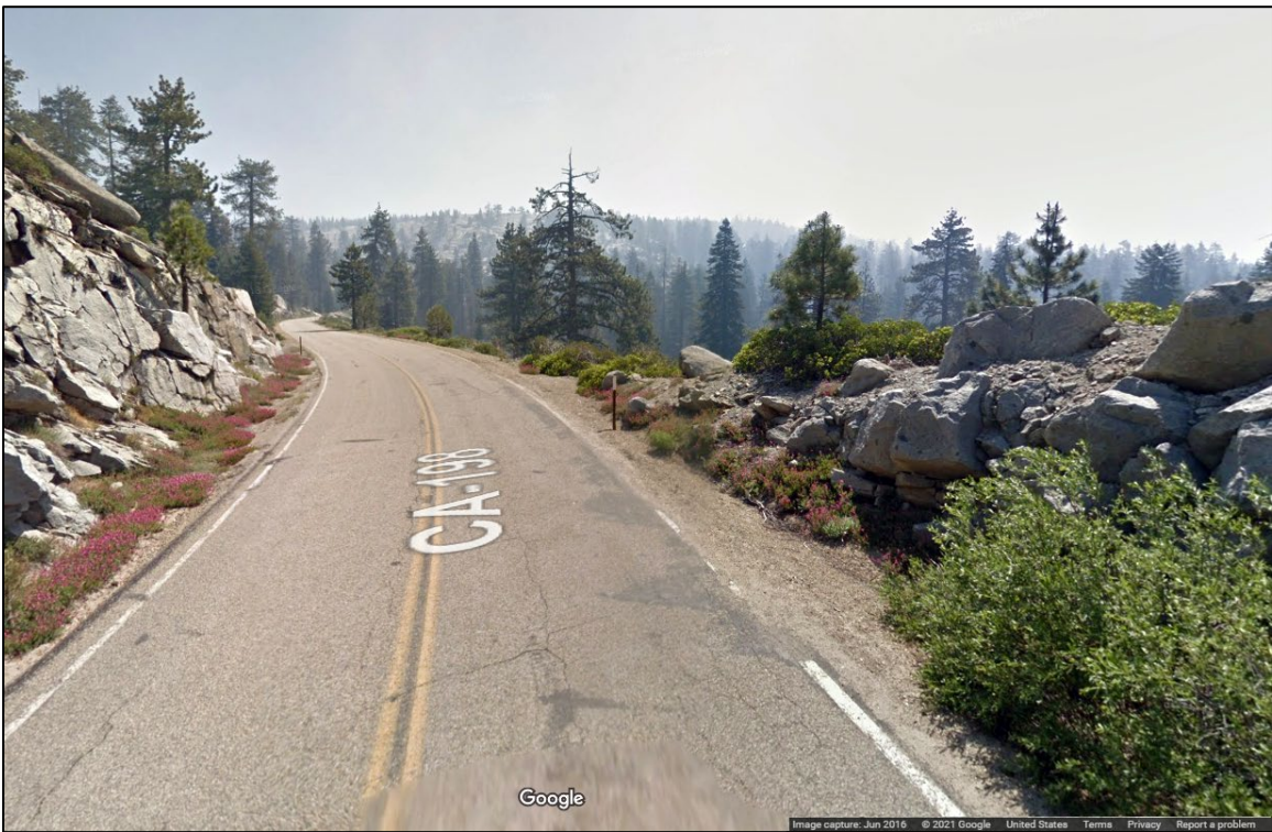
Figure 32. Looking northeast along south side curb and gutter (Google 2021).
