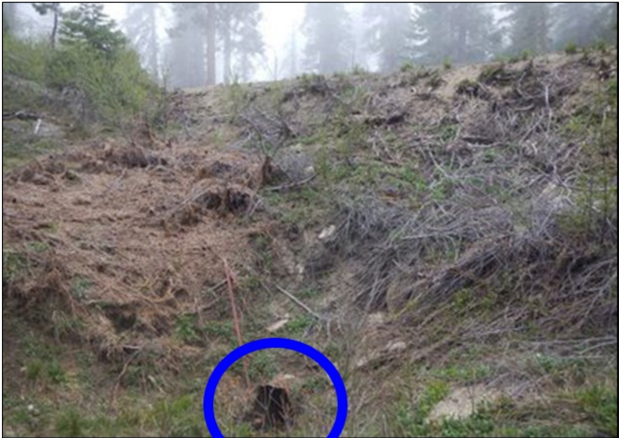
Figure 24. Outlet of Existing Culvert at the Wye.
