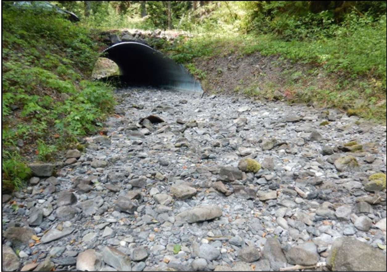
Figure 56. Looking upstream towards the Snider Creek Culvert.
