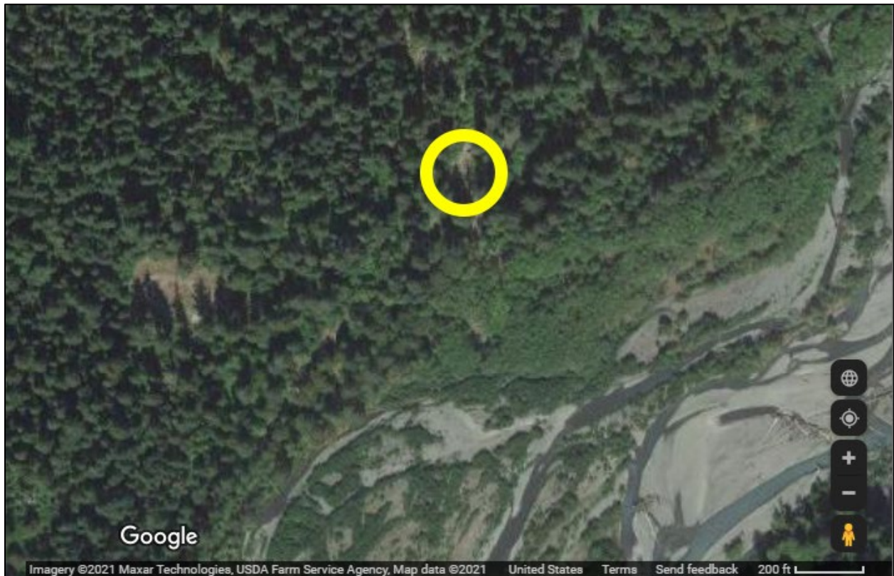
Figure 55. Aerial view of Snider Creek Culvert (Google 2021)
