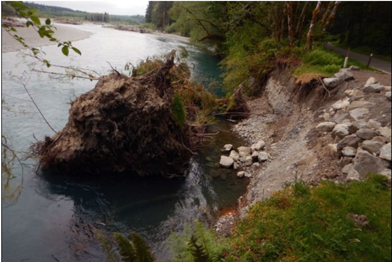
Figure 74. Looking downstream from the Hoh River stream bank (north to right).
