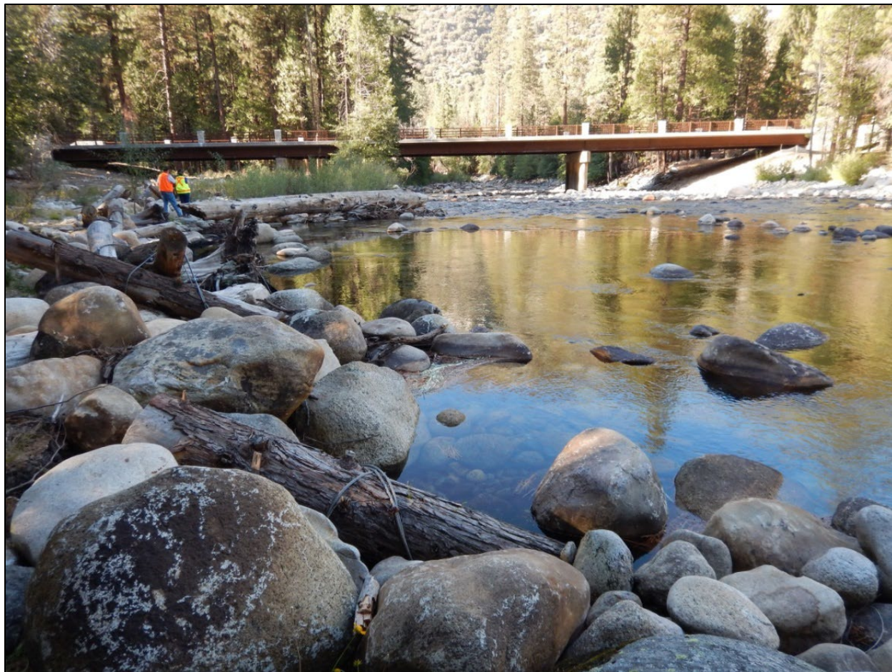
Figure 12. South Fork Kings River, Cedar Grove Bridge, view upstream of bridge.
