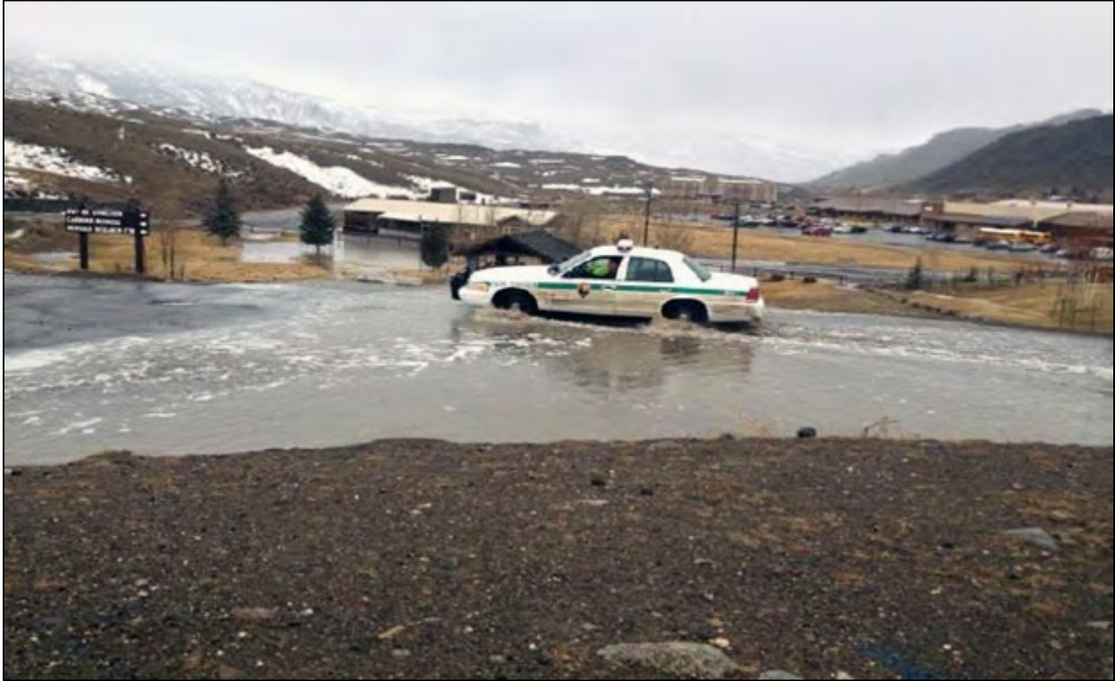
Figure 39. Runoff ponding at road profile sag west of the Arch.
