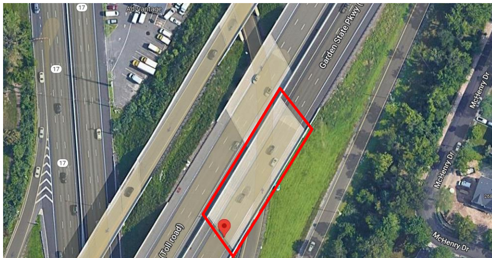
Figure 6. Structure 361632N – Aerial View.
