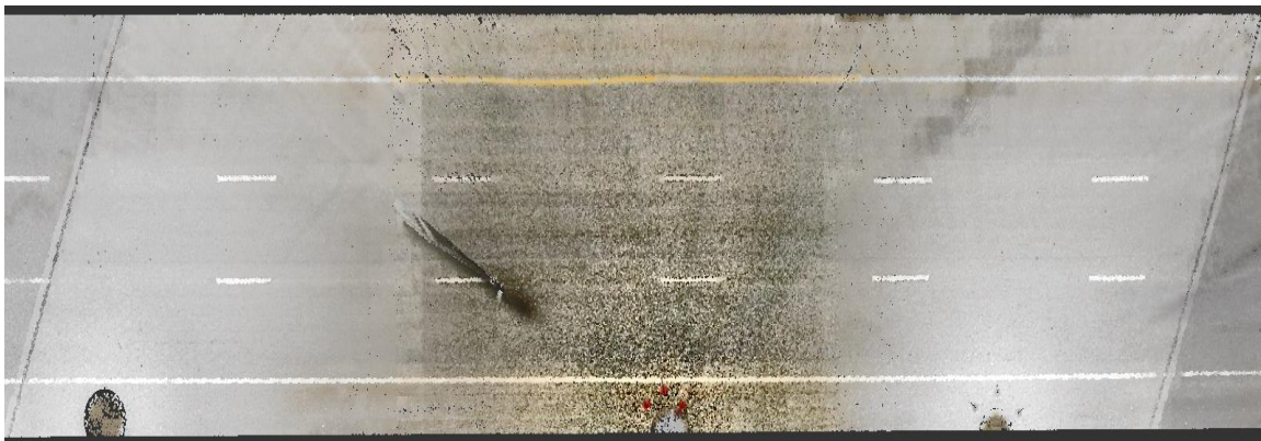
Figure 34. Structure 361632N - RGB image of the deck's top surface.
