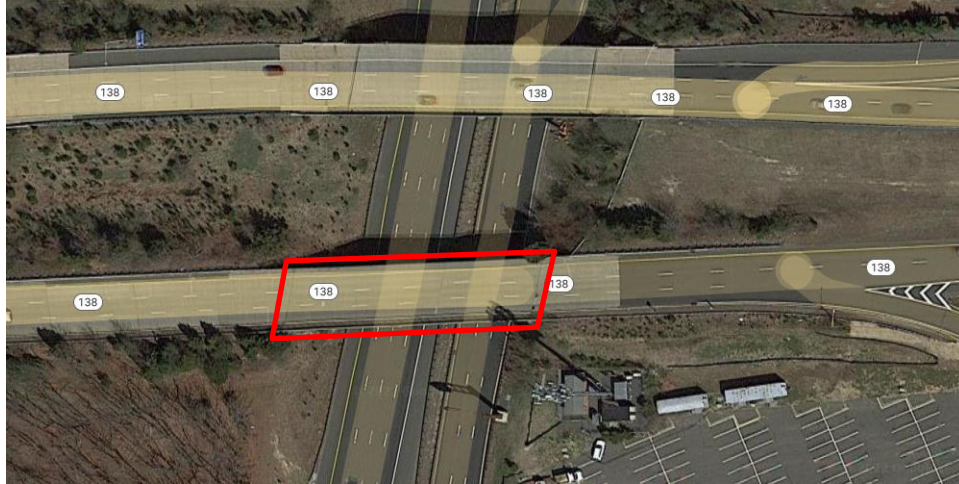
Figure 11. Structure 1317154 – Aerial View.
