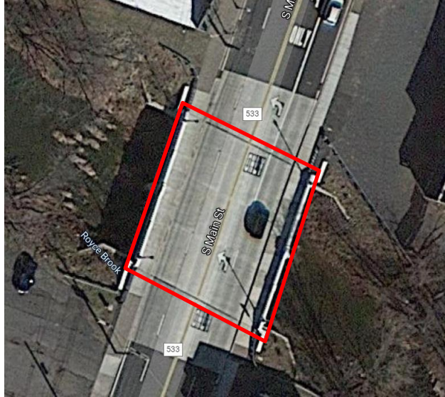
Figure7. Structure 18G0701 – Aerial View.
