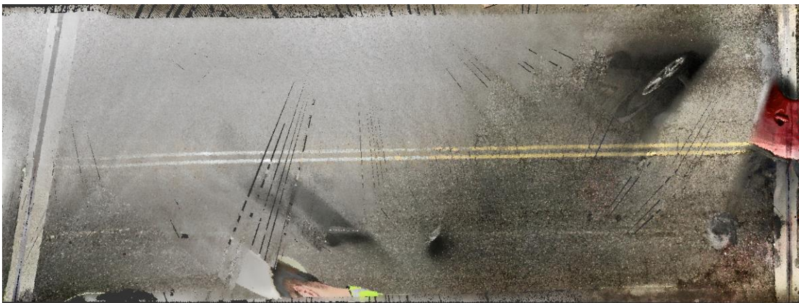
Figure 17. Structure 0954163 - RGB image of the deck's top surface.
