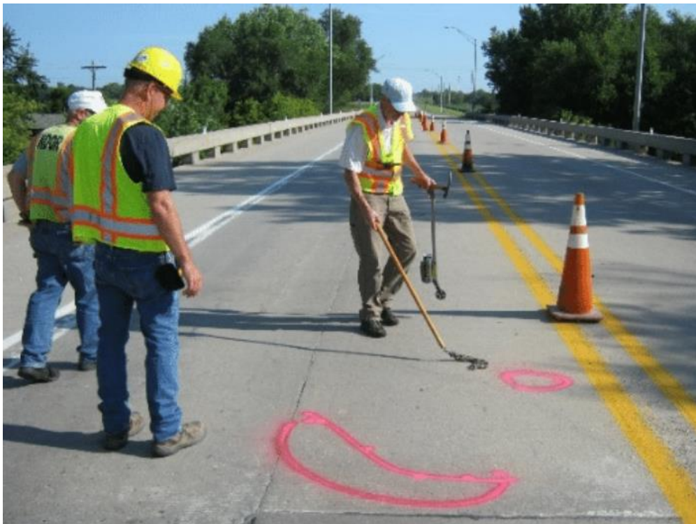
Figure 2. Chain Dragging Test (Source: www.researchgate.net ).
