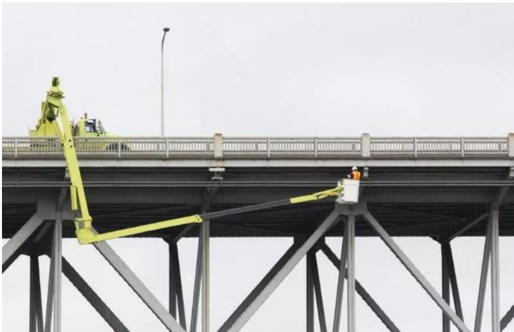
Figure 3. Visual Inspection on a Bridge using a Snoops Truck.
