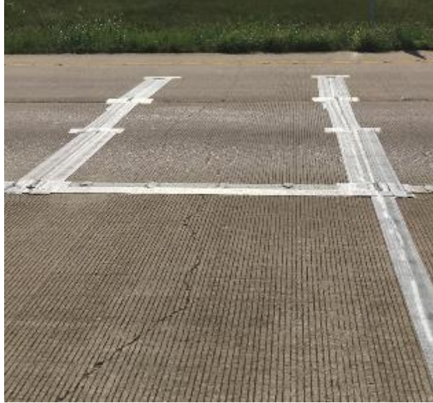
Figure 26. Portable WIM Installation on SH 130 in Travis County.
