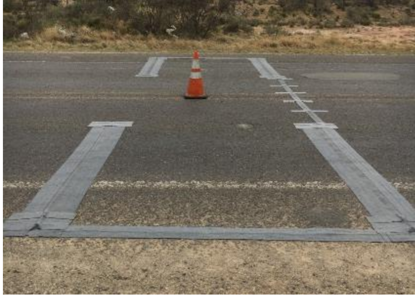
Figure 30. Portable WIM Installation on RM 652 in Culbertson County.
