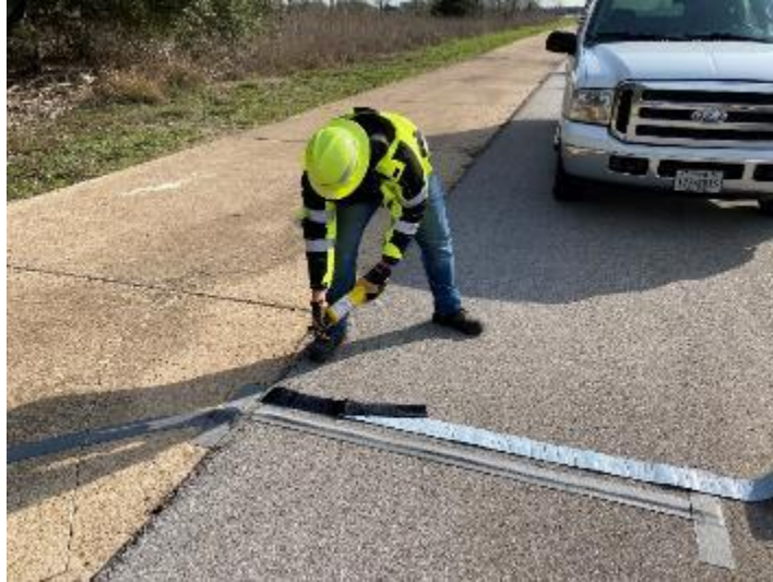
Figure 38. Heating up the Mastic Tapes
