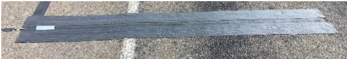
Figure 15. 6-Inch Road Tape Installed on the Road.
