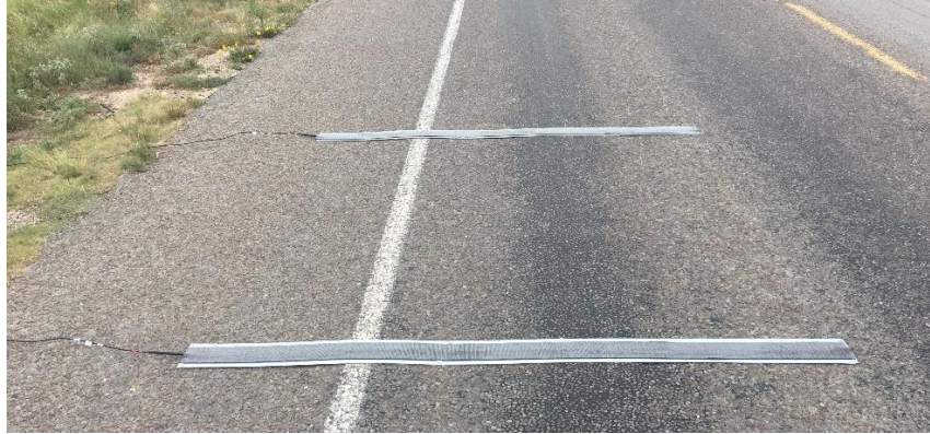
Figure 5. 8-ft Metal Plates Installed on the Road.
