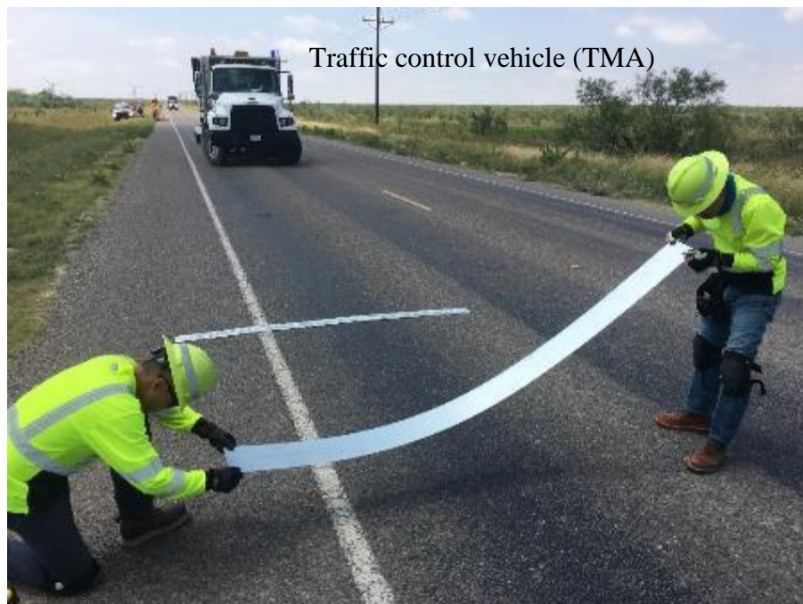
Figure 35. Placing the Metal Plates on the Marked Area.
