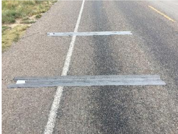
Figure 41. 4-Inch Road Tape Applied on the Pavement.
