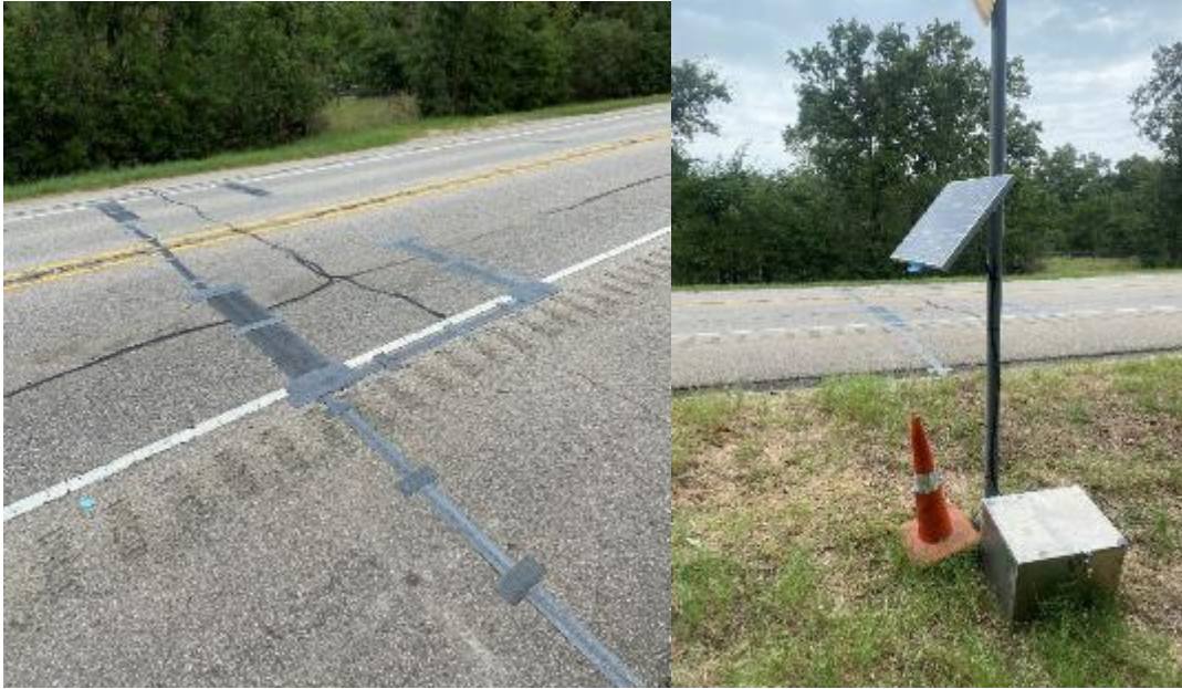
Figure 87. Portable WIM Installation on US 190, Bryan District.
