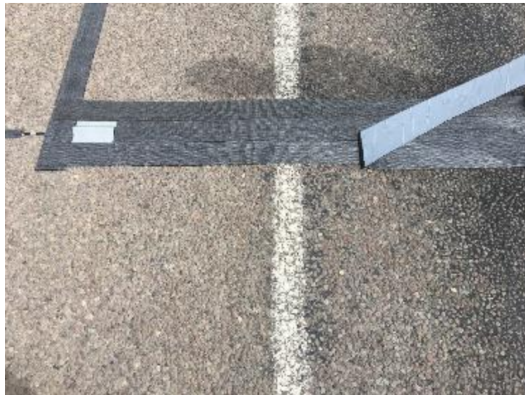
Figure 42. Applying 6-Inch Road Tape.
