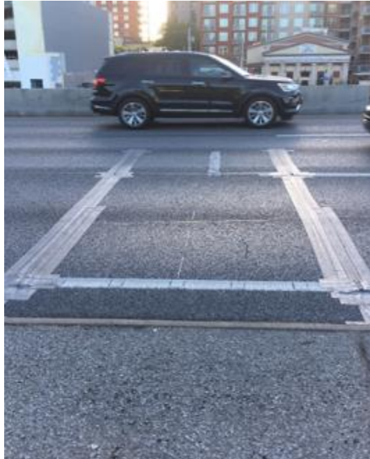
Figure 28. Portable WIM Installation on IH 35 in Travis County.
