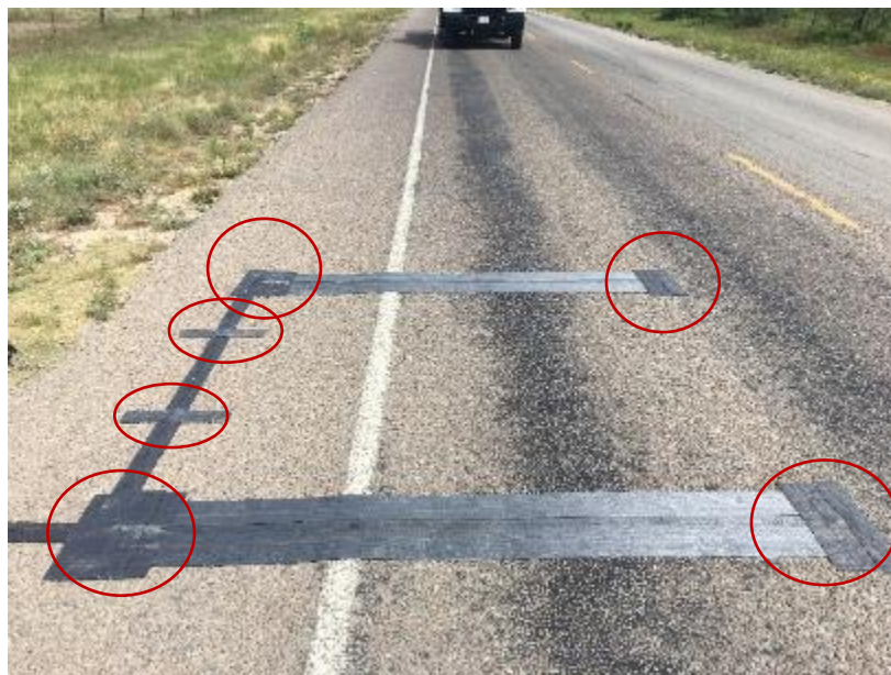
Figure 44. Horizontal Road Tapes (about 20-Inch Long).
