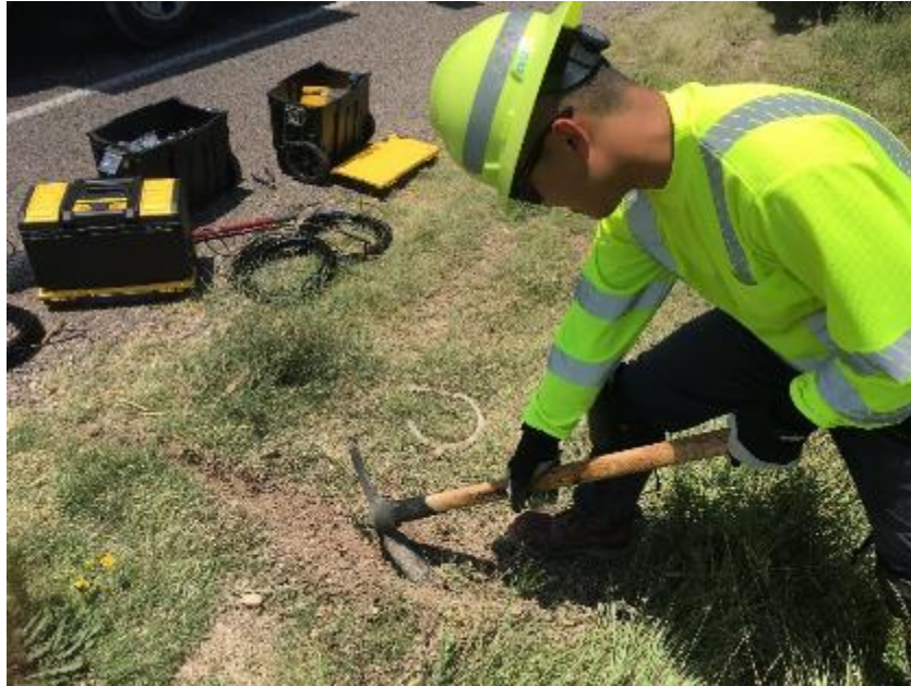
Figure 46. Digging a Trench.
