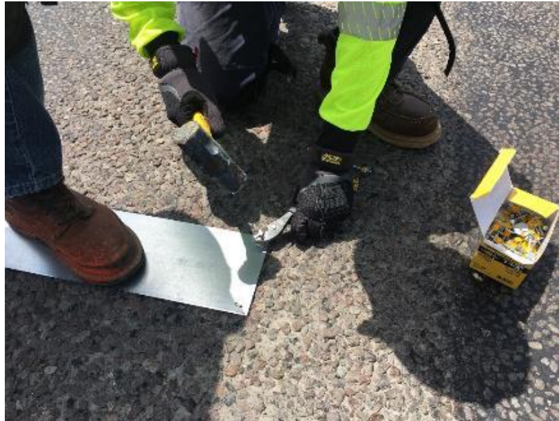
Figure 36. Nailing the Metal Plates.
