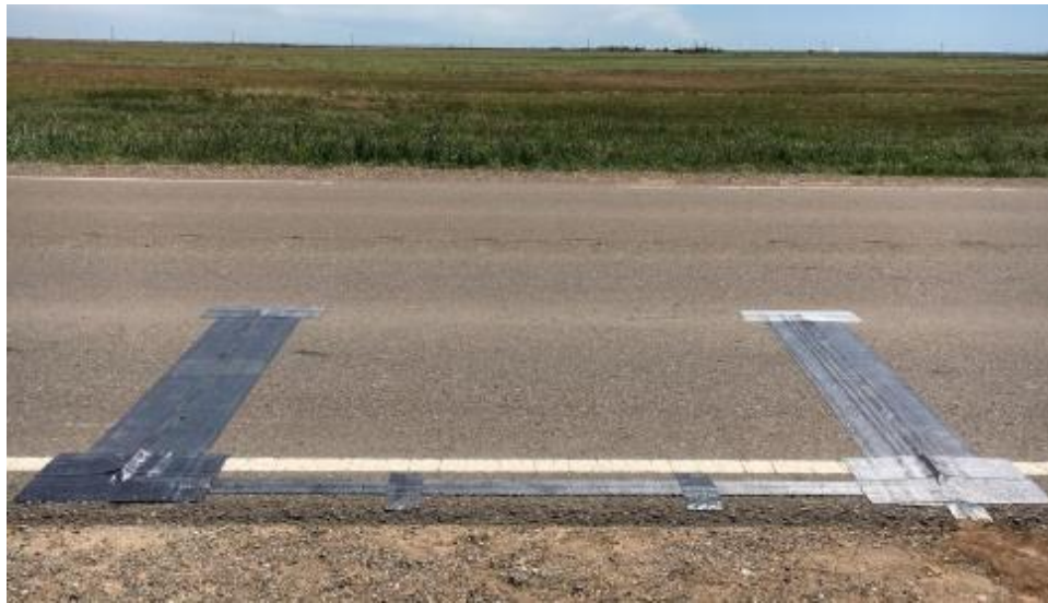
Figure 22. Portable WIM Installation on FM 281 in Moore County.
