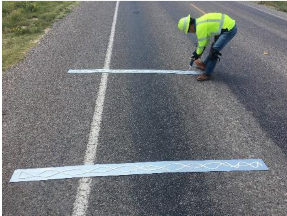
Figure 34. Applying Silicon Adhesive Using Caulk Gun.
