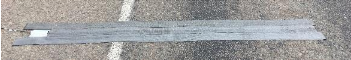
Figure 14. 4-Inch Road Tape Installed on the Road.
