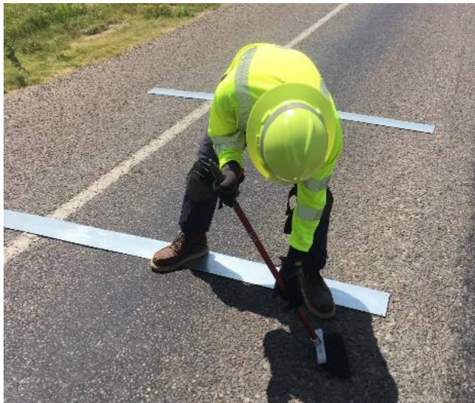
Figure 33. Cleaning the Marked Area.
