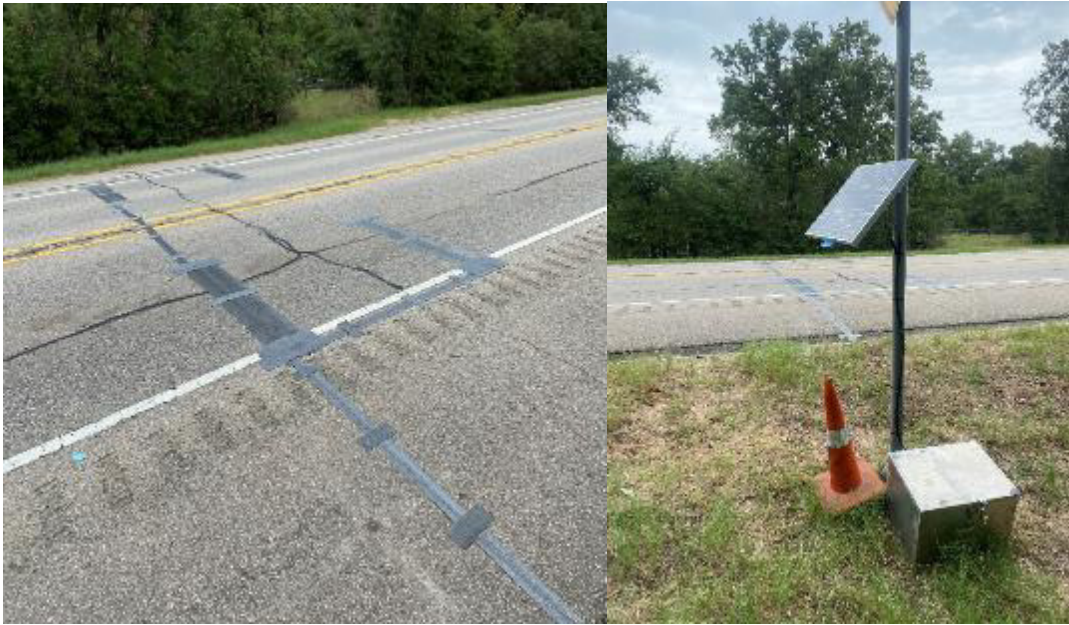
Figure 30. Portable WIM Installation on US 190, Bryan District.
