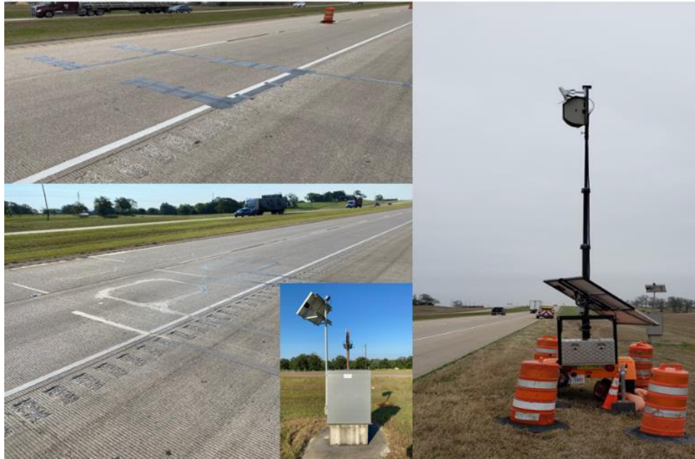
Figure 44. Portable WIM Demo-Monitoring Testing Station in SH 6 (SB), Bryan District.
