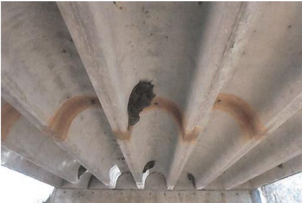
(b) Underside view
