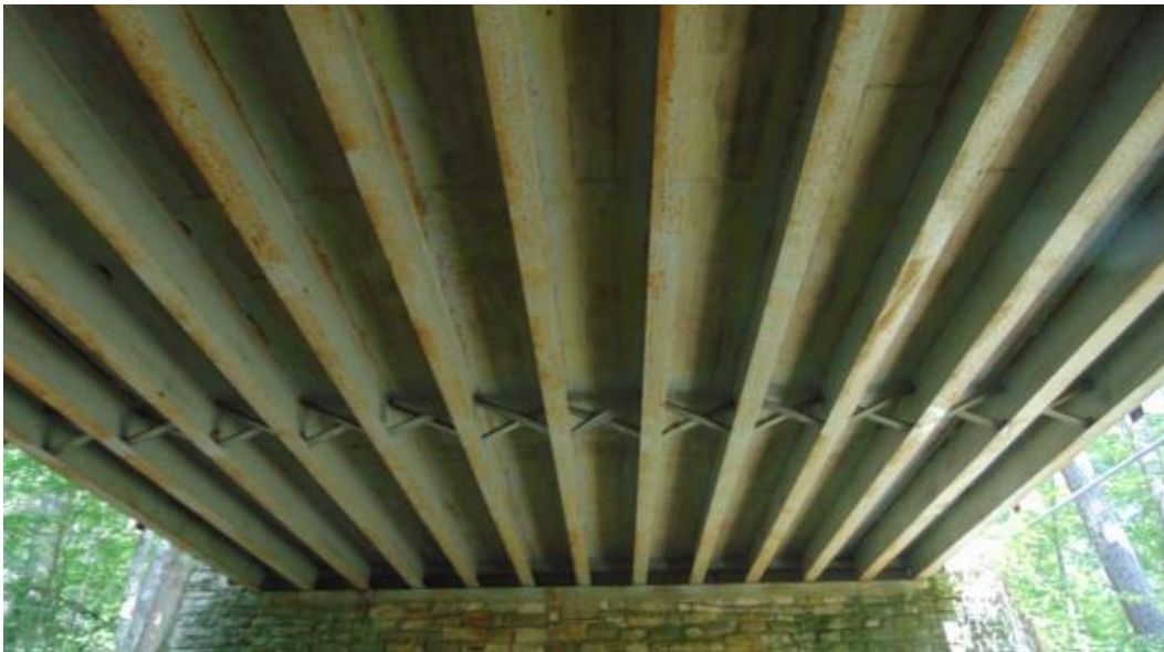
(b) Underside view
