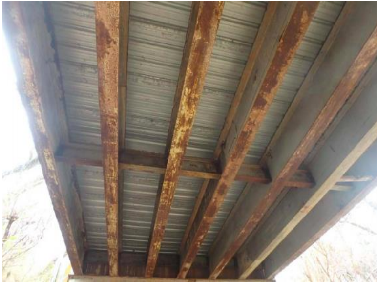
(b) Underside view
