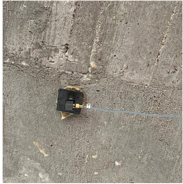
(b) Installed Accelerometer
