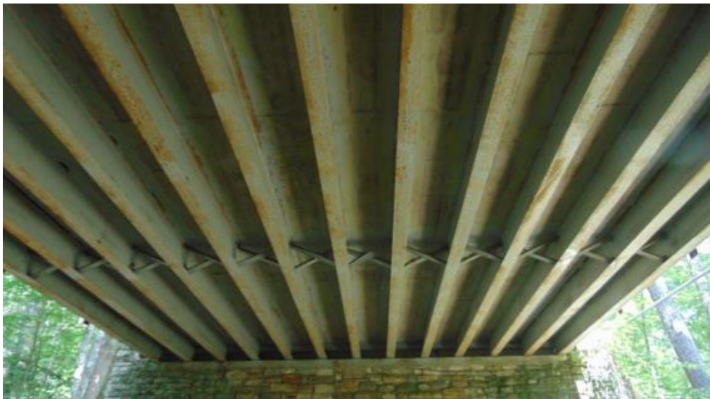
(b) Underside view
