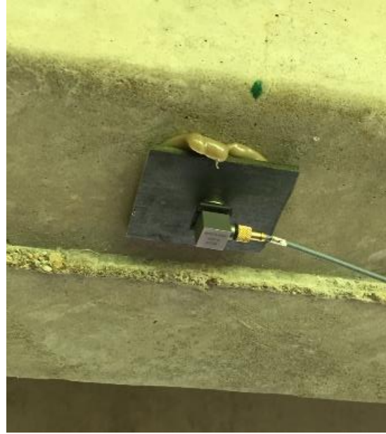
(b) Installed Accelerometer
