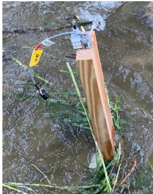
(c) Example of an Installed String Potentiometer
