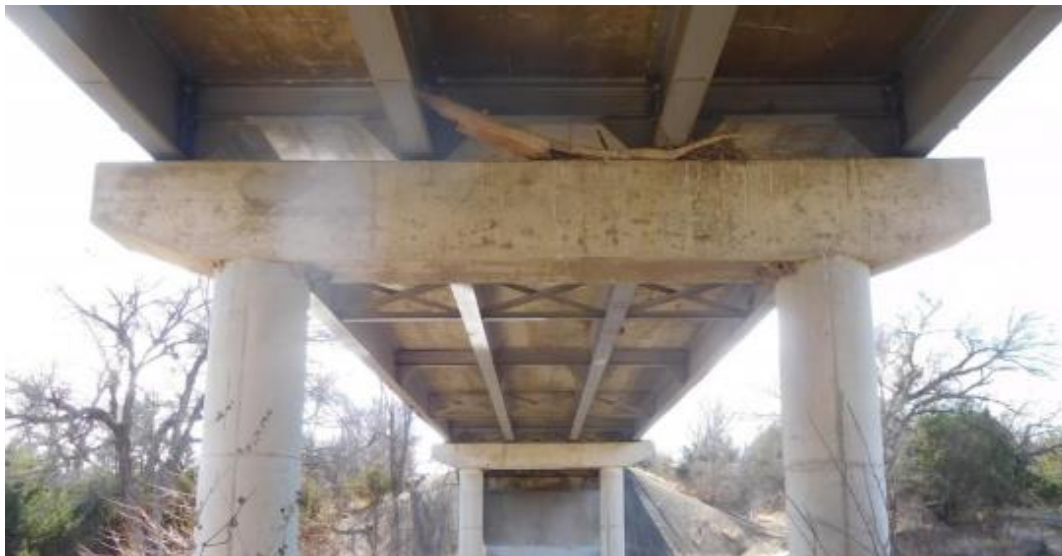
(b) Underside view
