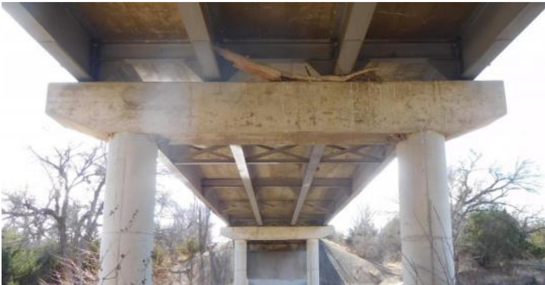
(b) Underside view
