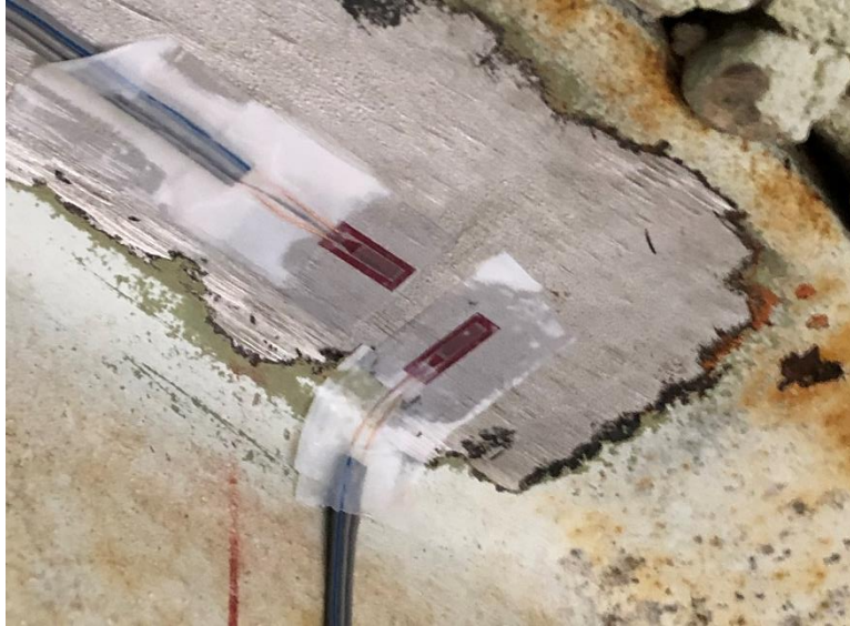
Figure 6.9. Close-Up of Strain Gauge Installation
