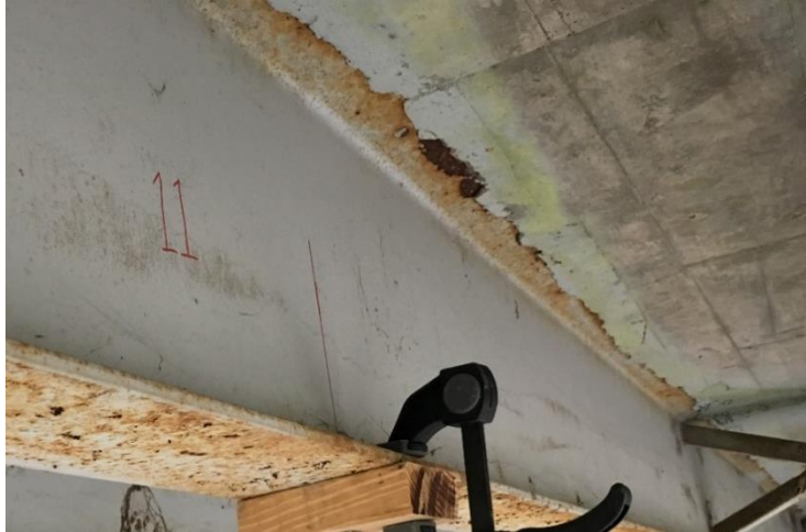
Figure 6.3. Observation of Girder Flange Embedment with No Signs of Cracking
