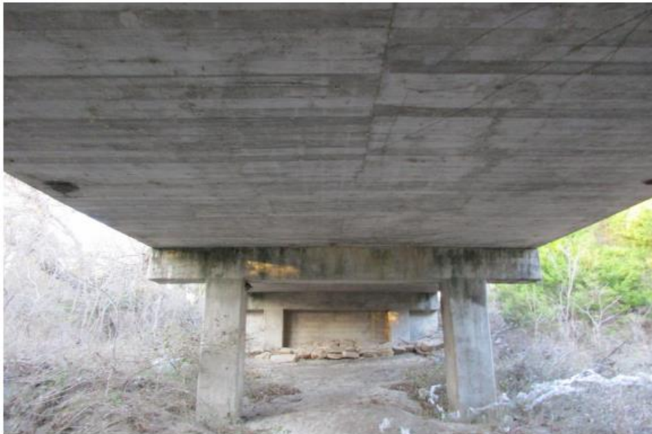
(b) Underside View
