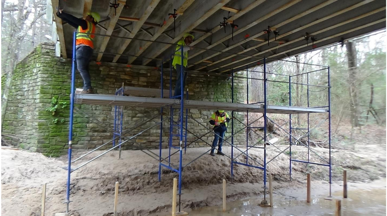
(a) Instrumentation of Bridge SM-5
