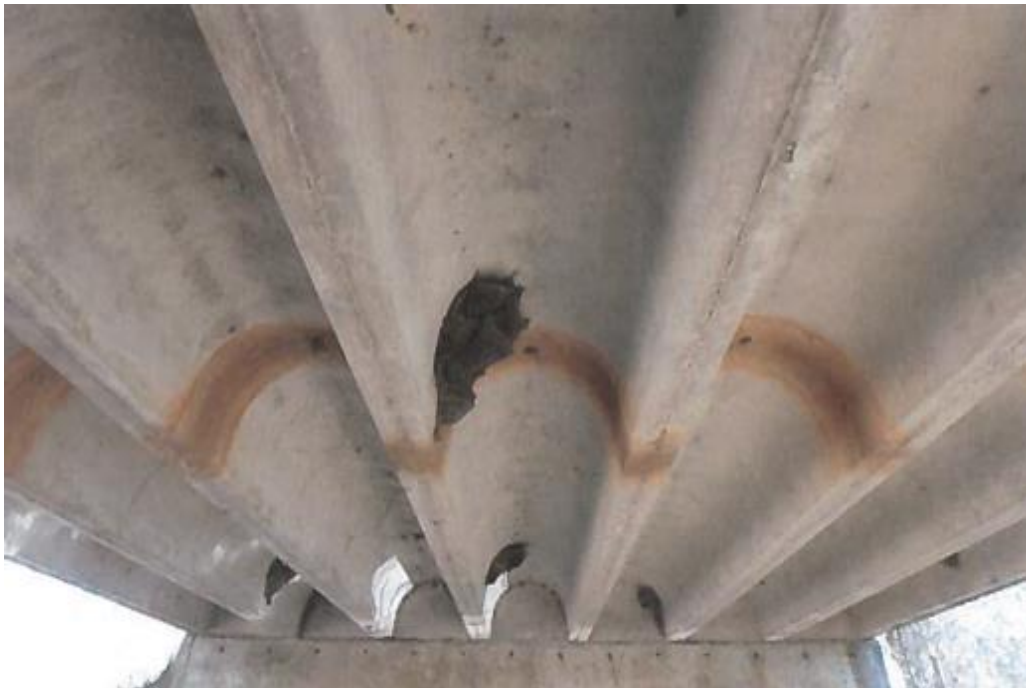
(b) Underside view
