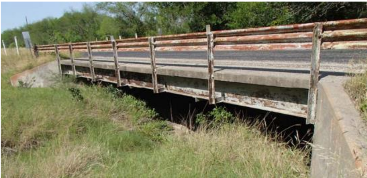
Figure B.1. Bridge SM-1 (TxDOT 2018c)
