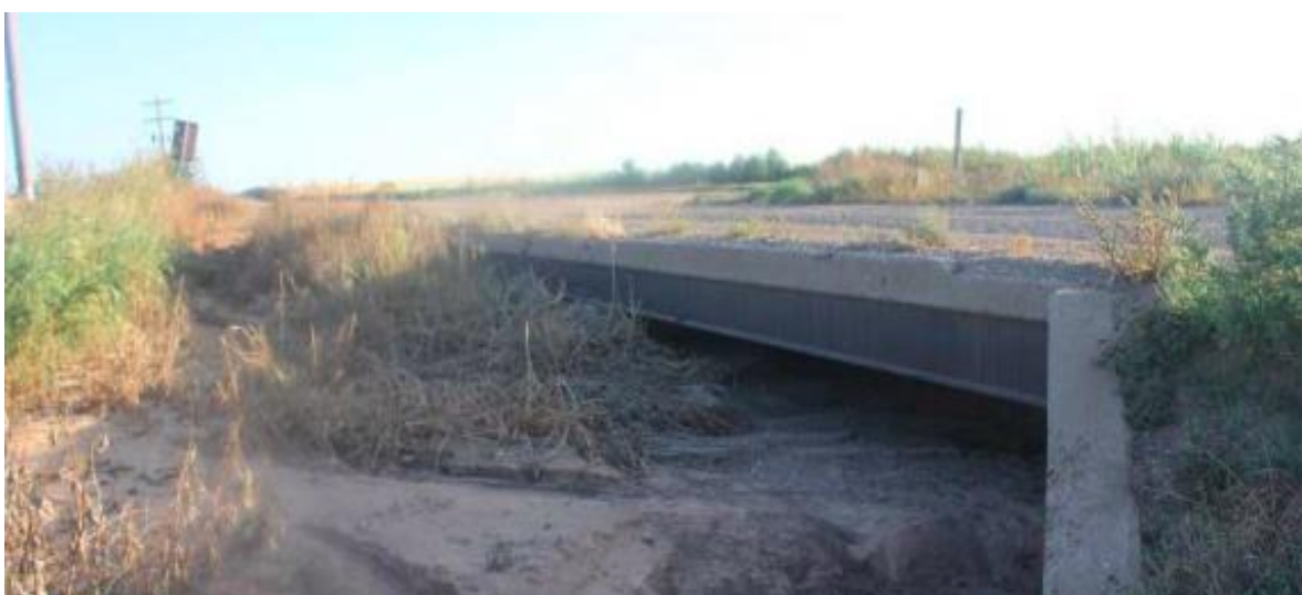
Figure B.11. Bridge SM-6 (TxDOT 2018c)
