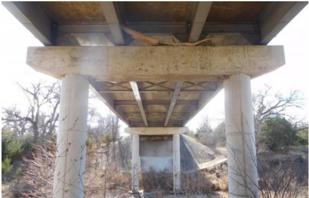
(c) Underside Superstructure View
