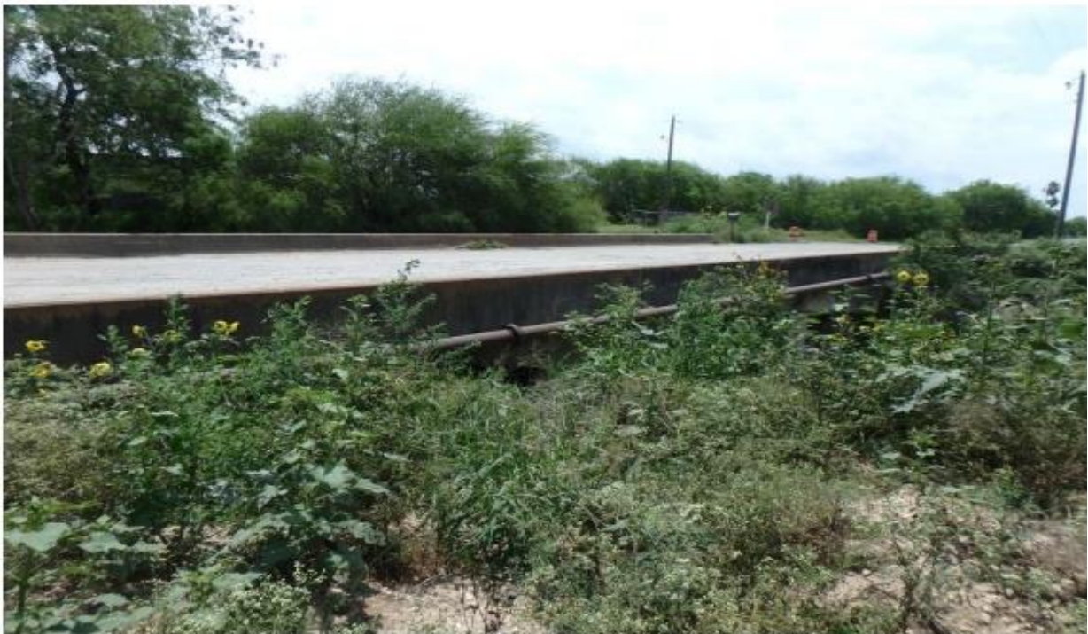
Figure C.41. Bridge CS-21 (TxDOT 2018c)
