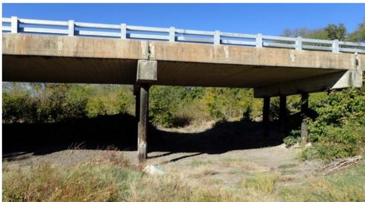
Figure C.15. Bridge CS-8 (TxDOT 2018c)
