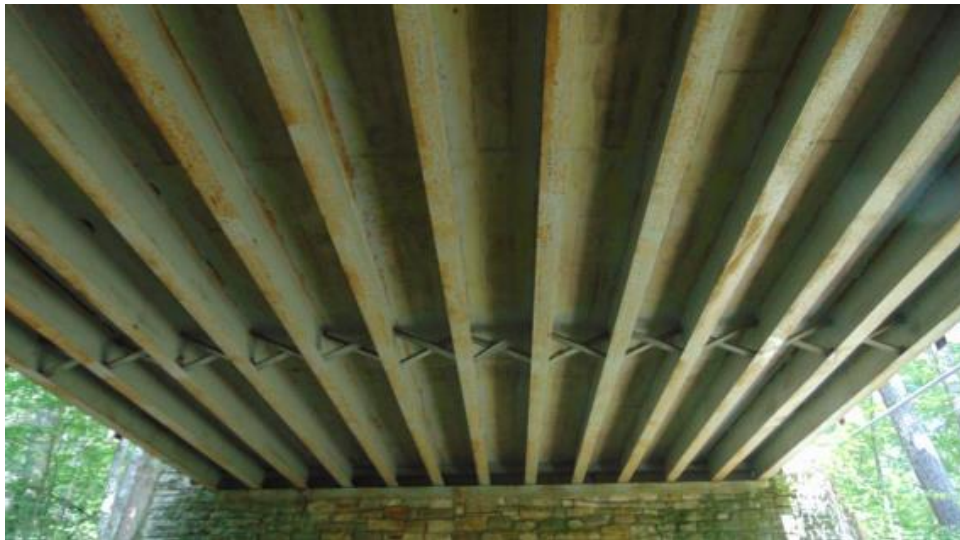
(c) Underside Superstructure View
