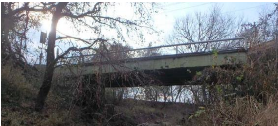
Figure B.41. Bridge SM-21 (TxDOT 2018c)
