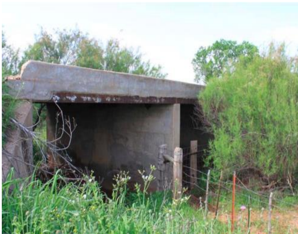
Figure B.71. Bridge SC-11 (TxDOT 2018c)
