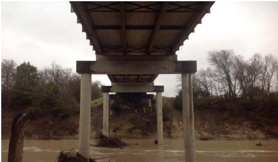
(c) Underside Superstructure View
