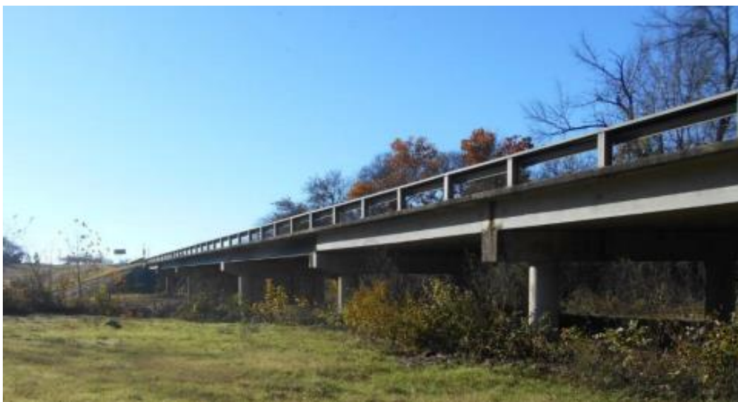
Figure B.75. Bridge SC-13 (TxDOT 2018c)
