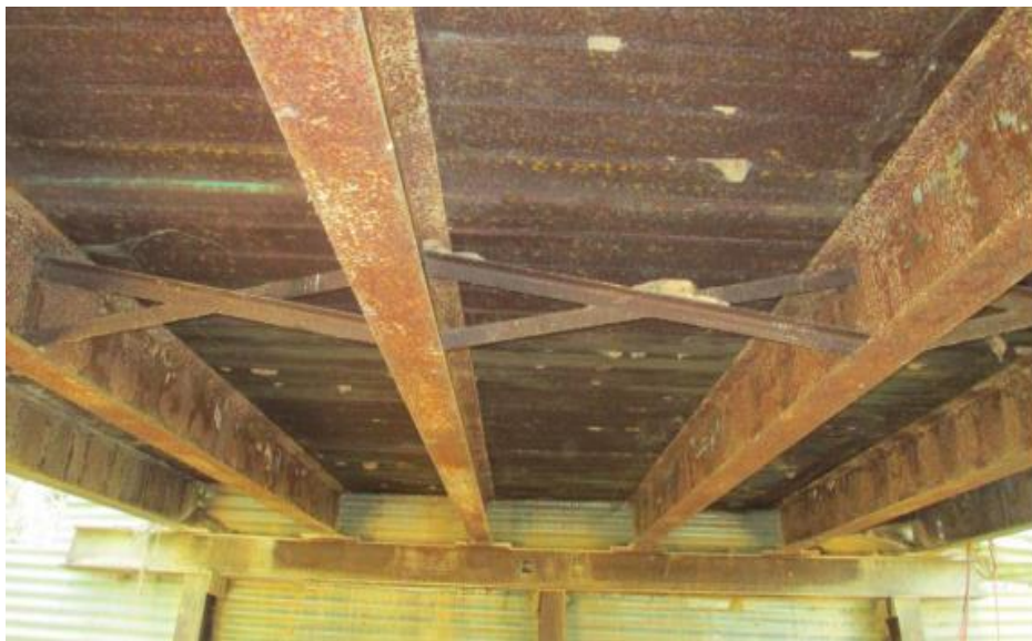
(c) Underside Superstructure View
