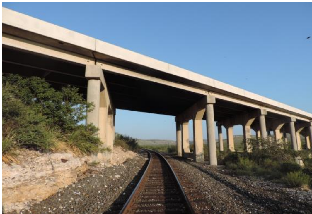
Figure B.21. Bridge SM-11 (TxDOT 2018c)
