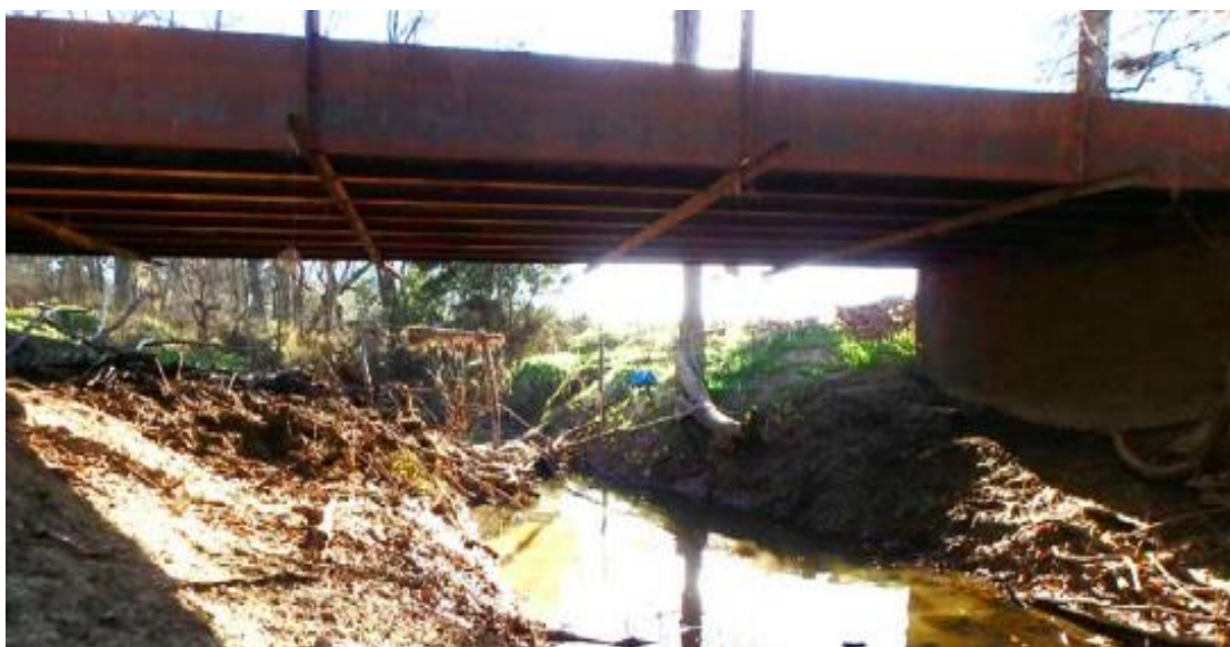
Figure B.27. Bridge SM-14 (TxDOT 2018c)
