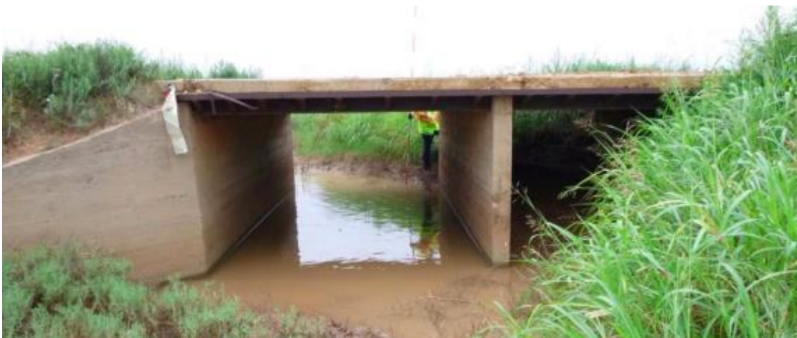
Figure B.67. Bridge SC-9 (TxDOT 2018c)
