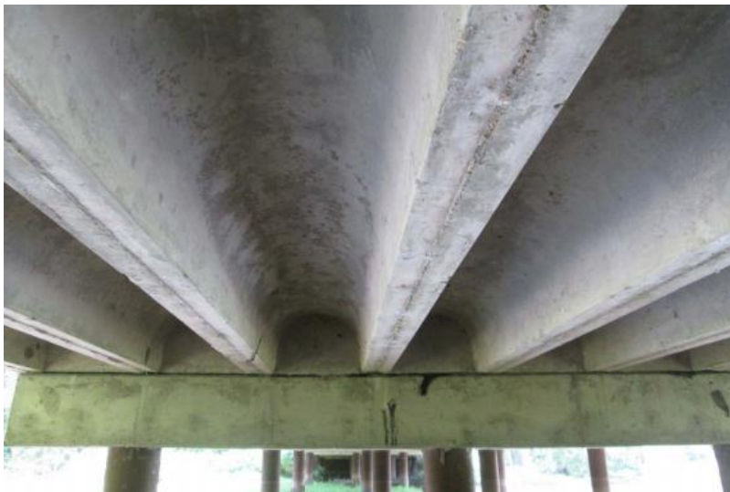
(c) Underside Superstructure View
