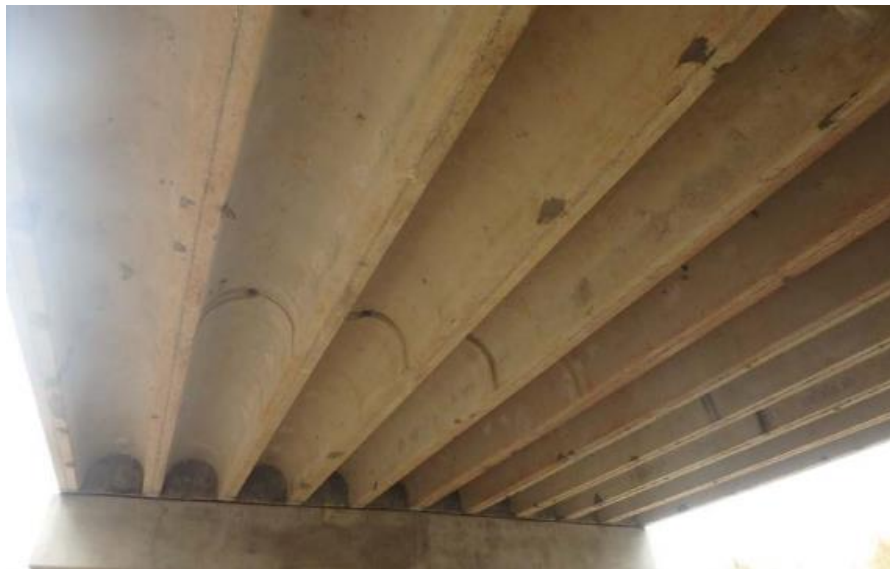
(c) Underside Superstructure View
