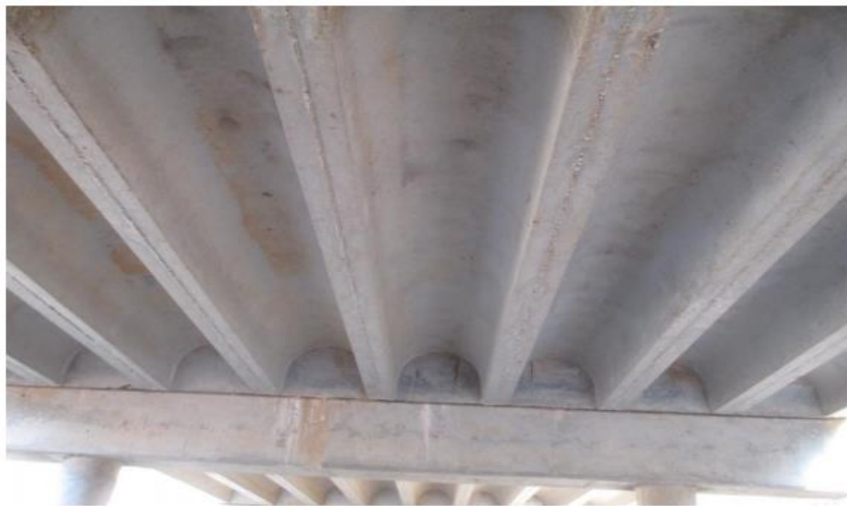
(c) Underside Superstructure View
