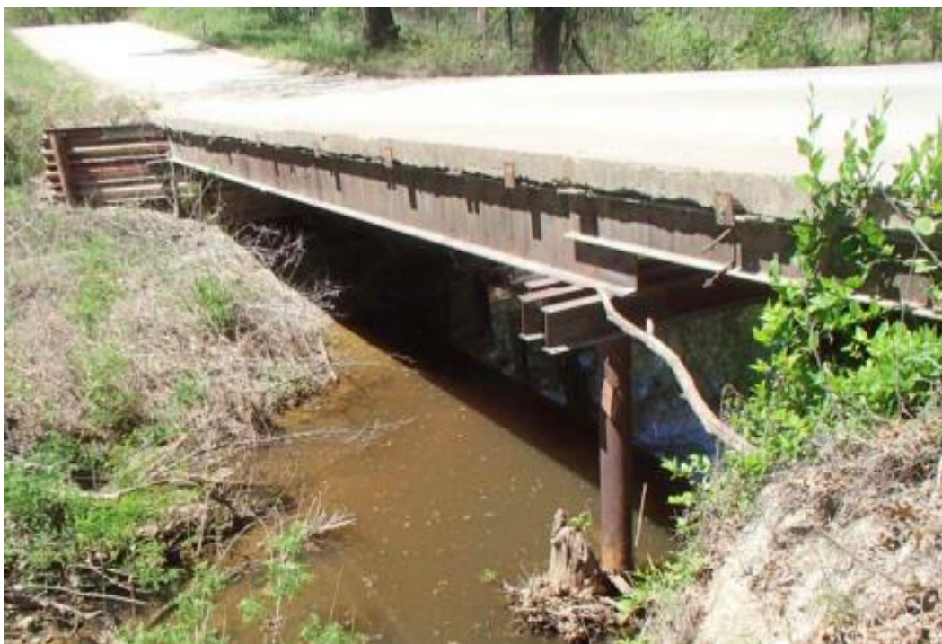
Figure B.77. Bridge SC-14 (TxDOT 2018c)
