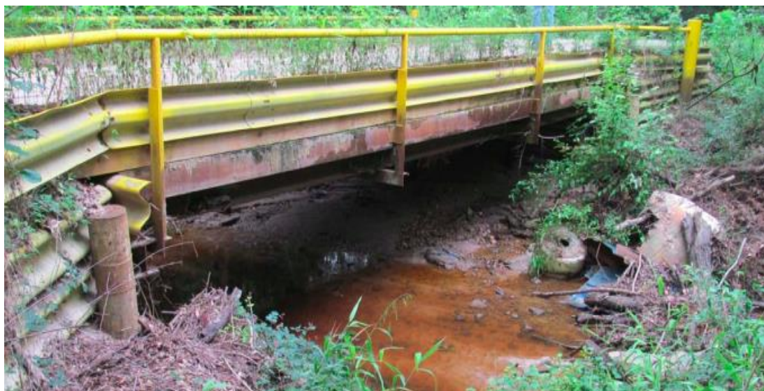
Figure B.47. Bridge SM-24 (TxDOT 2018c)
