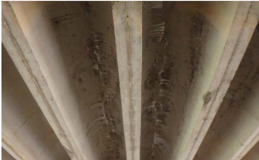
(c) Underside Superstructure View
