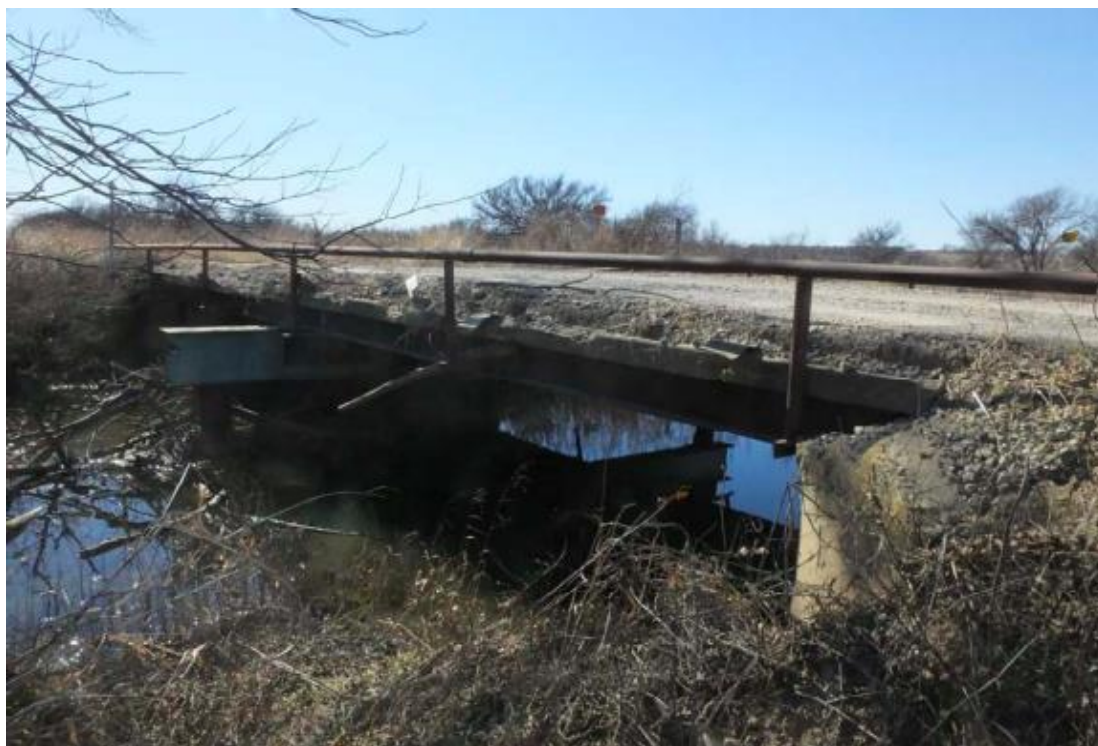
Figure B.57. Bridge SC-4 (TxDOT 2018c)
