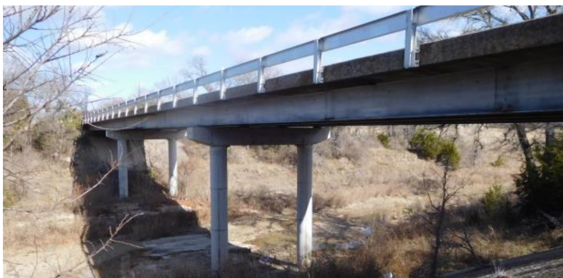
Figure 7.3. Bridge SC-12 (TxDOT 2018c)
