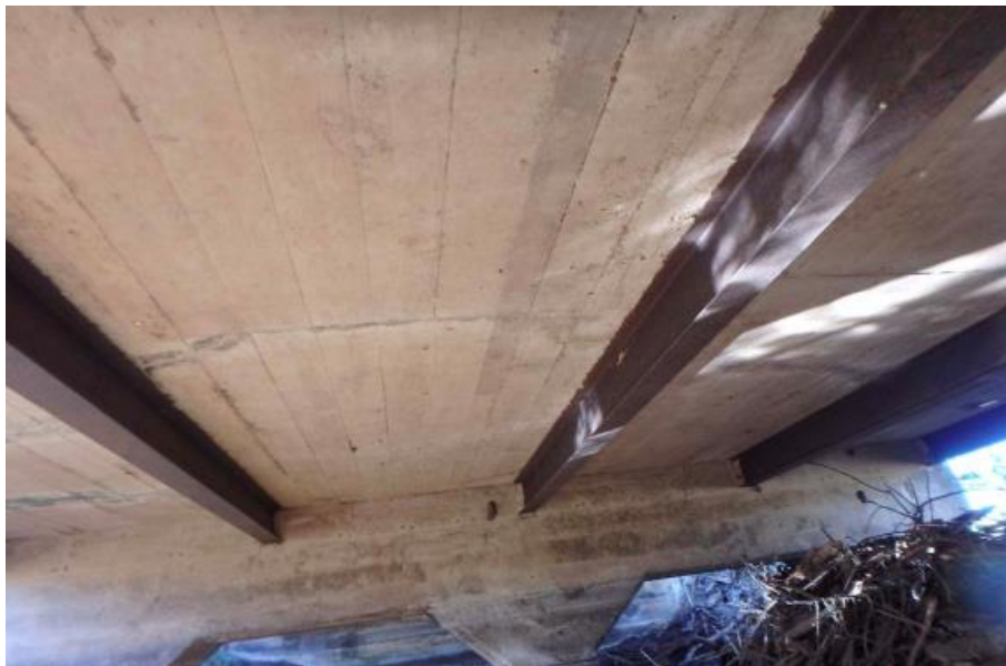
(c) Underside Superstructure View
