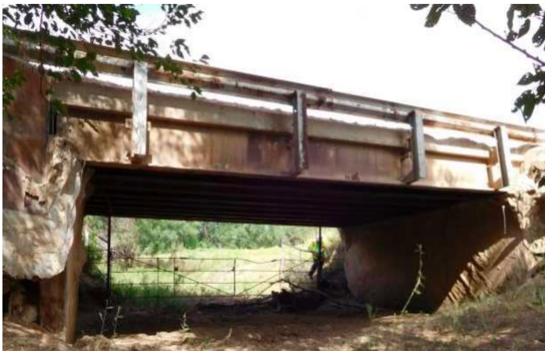
Figure B.49. Bridge SM-25 (TxDOT 2018c)
