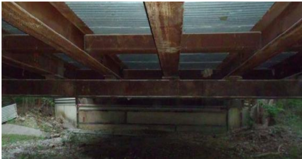
(c) Underside Superstructure View
