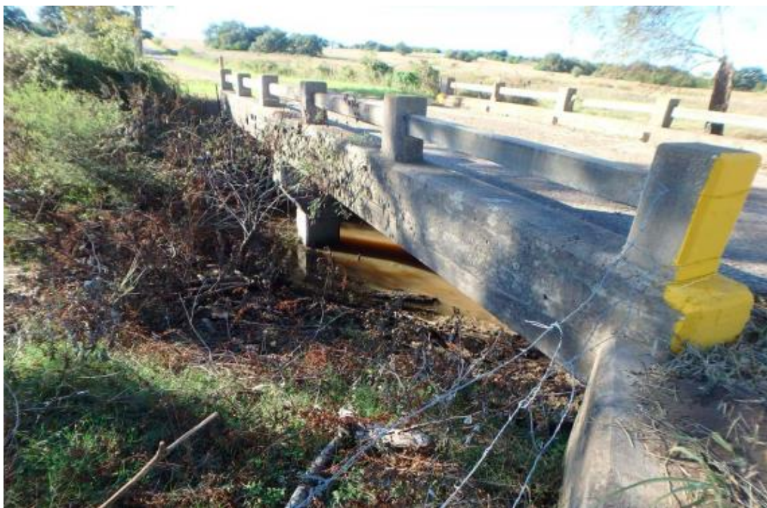
Figure B.59. Bridge SC-5 (TxDOT 2018c)
