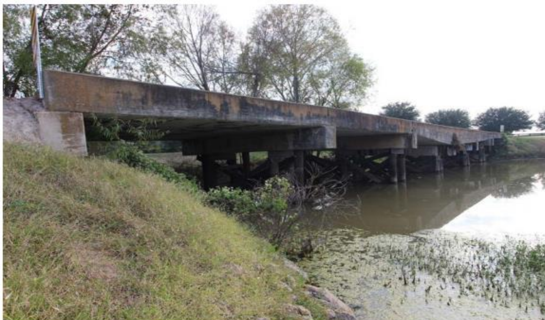
Figure C.13. Bridge CS-7 (TxDOT 2018c)
