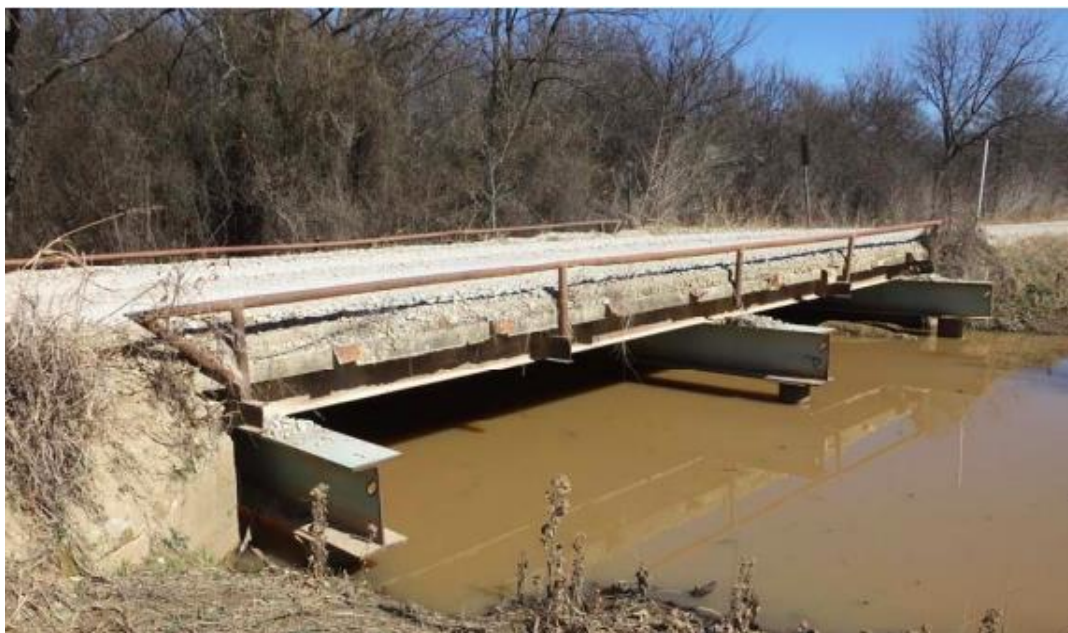
Figure B.55. Bridge SC-3 (TxDOT 2018c)
