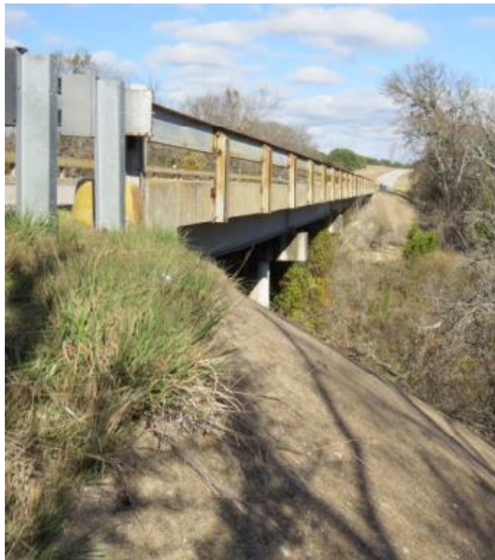
Figure B.29. Bridge SM-15 (TxDOT 2018c)
