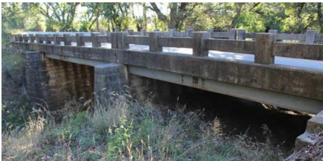
Figure B.13. Bridge SM-7 (TxDOT 2018c)
