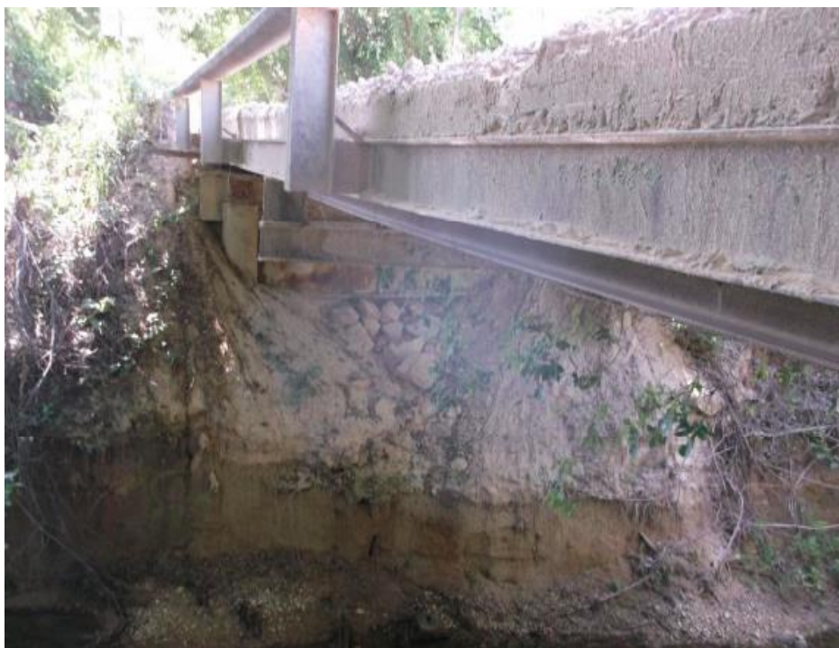
Figure B.35. Bridge SM-18 (TxDOT 2018c)
