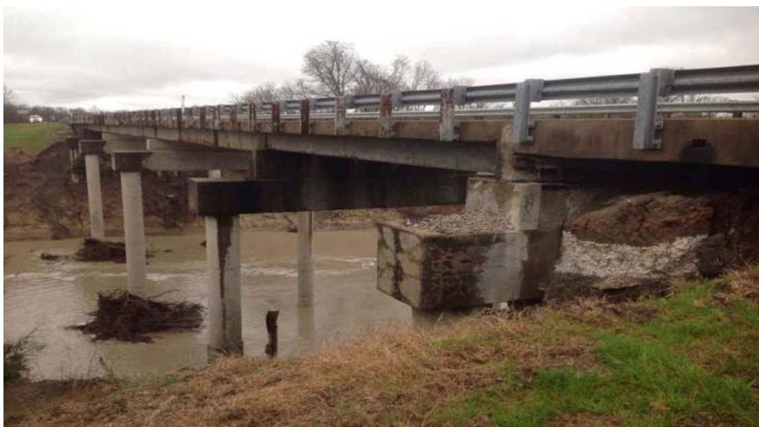
Figure B.65. Bridge SC-8 (TxDOT 2018c)
