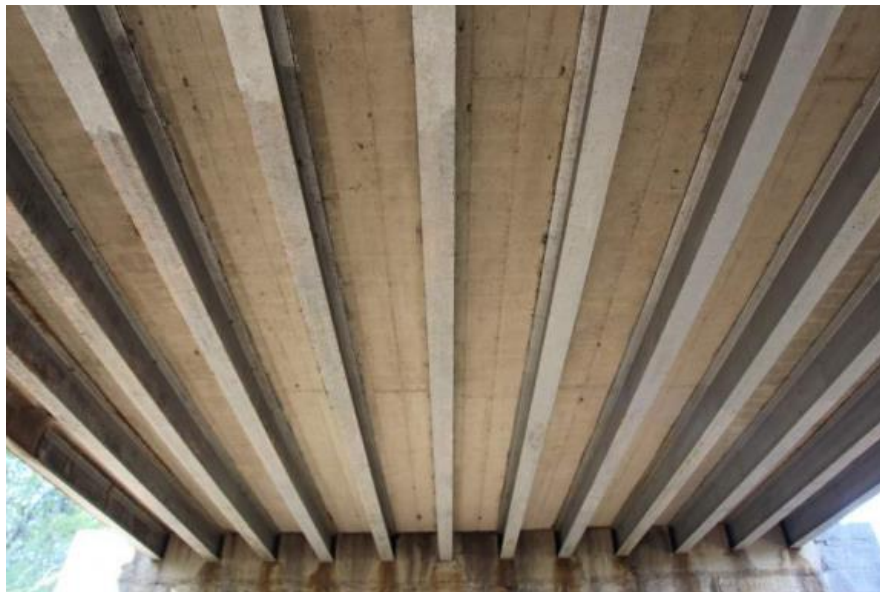
(c) Underside Superstructure View
