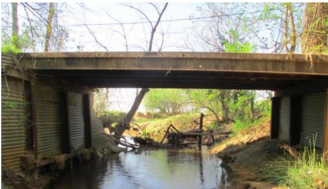
Figure B.37. Bridge SM-19 (TxDOT 2018c)
