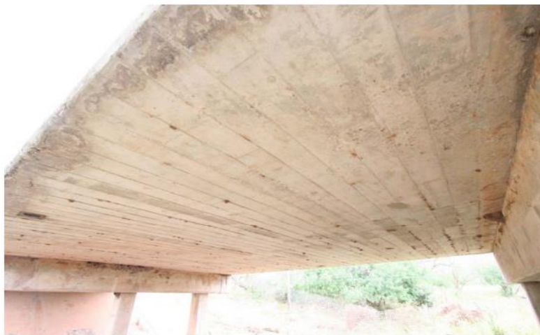
(c) Underside Superstructure View
