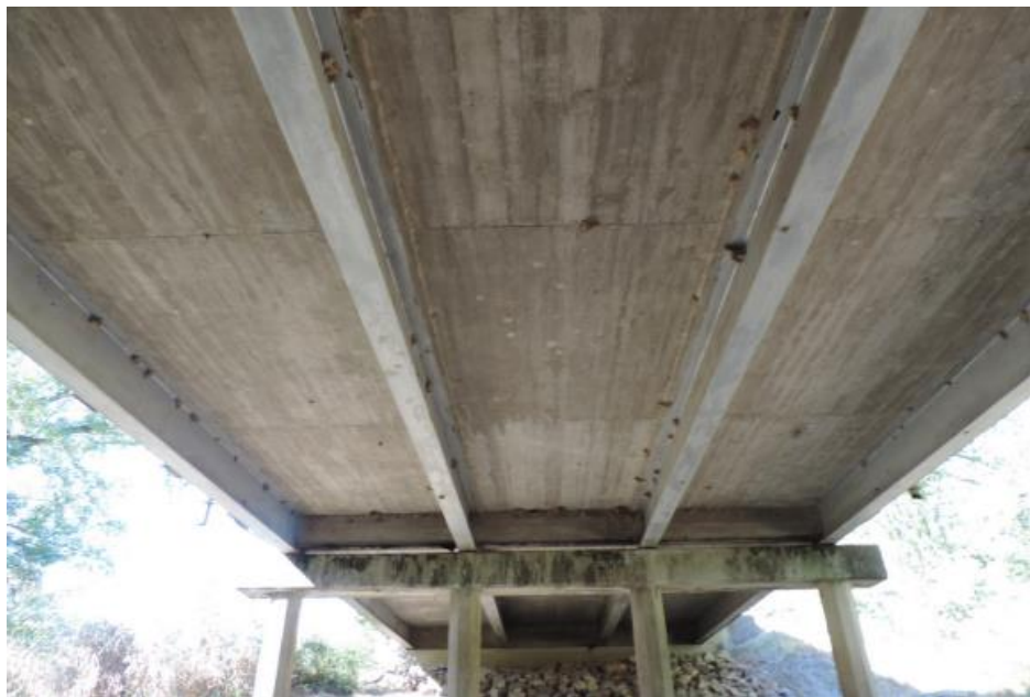
(c) Underside Superstructure View
