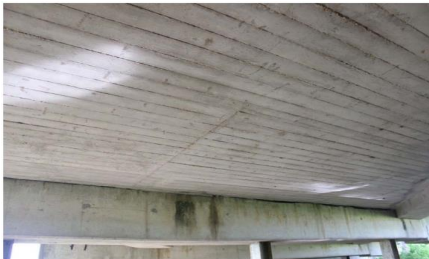
(c) Underside Superstructure View
