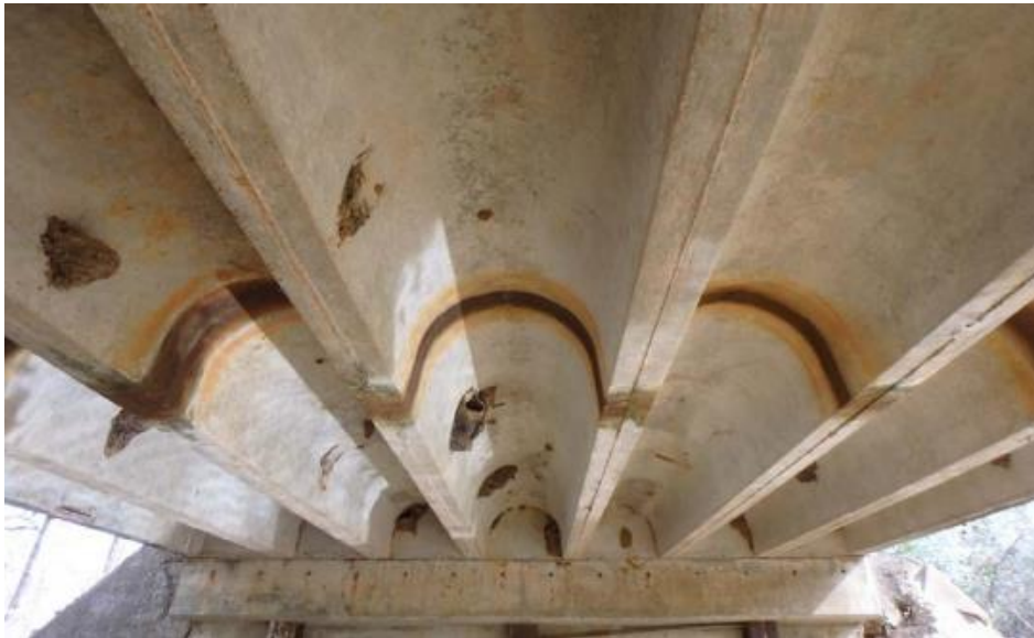
(c) Underside Superstructure View
