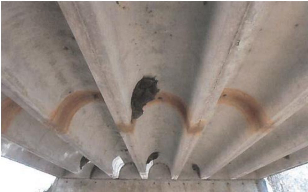
(c) Underside Superstructure View
