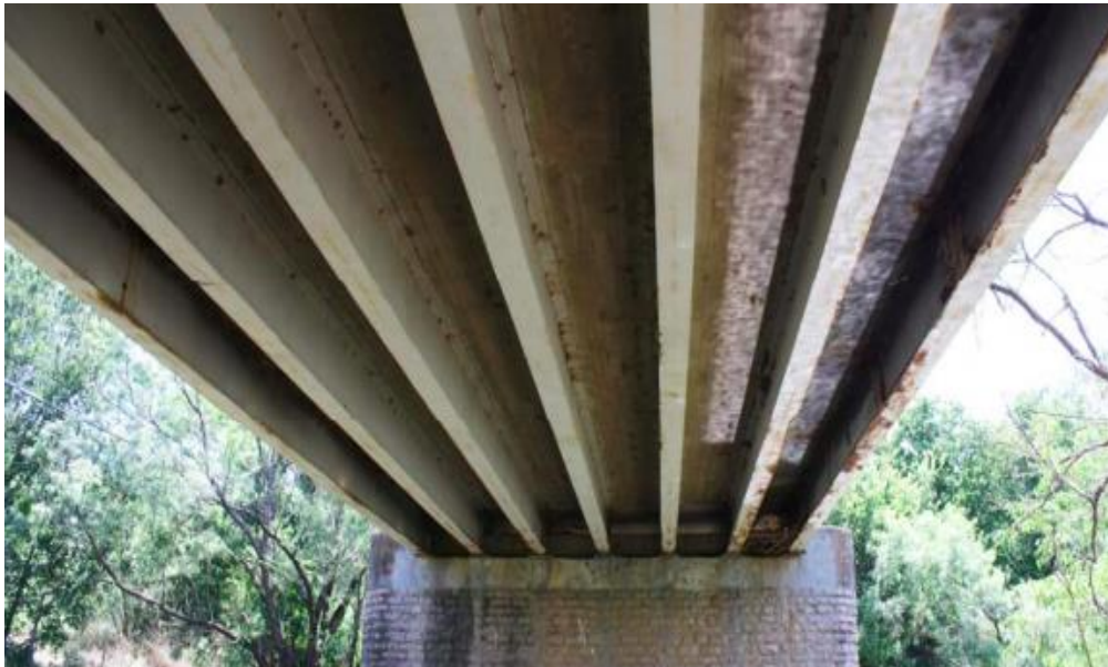
(c) Underside Superstructure View
