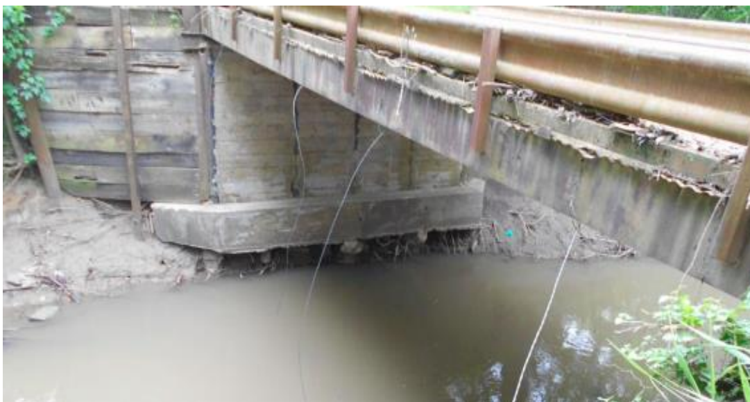
Figure B.33. Bridge SM-17 (TxDOT 2018c)
