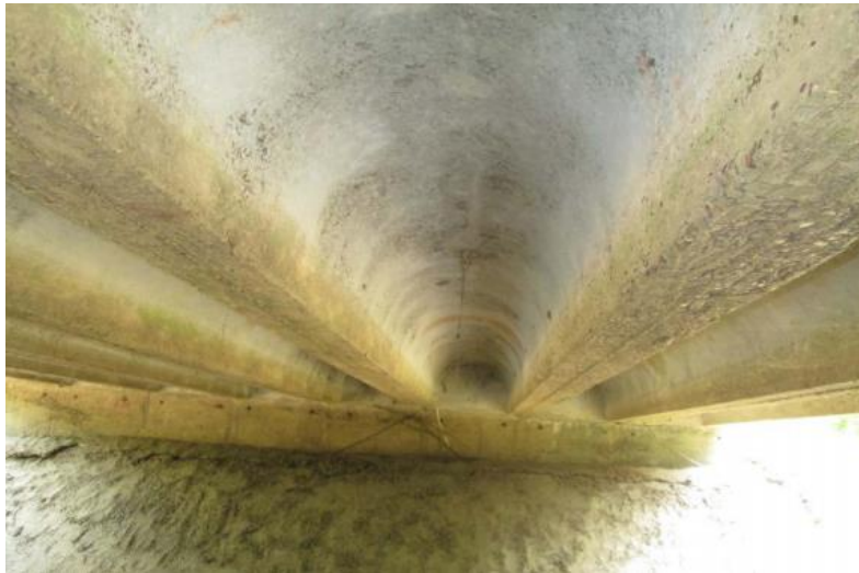
(c) Underside Superstructure View
