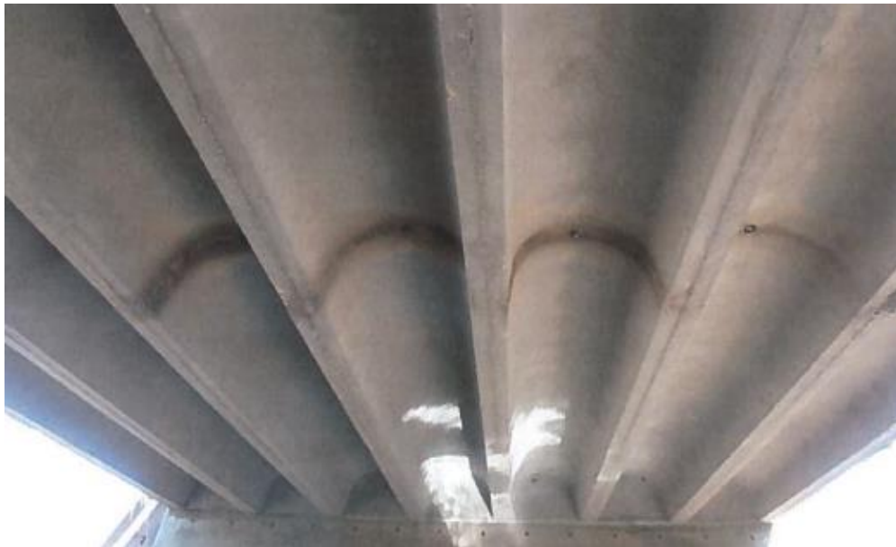
(c) Underside Superstructure View
