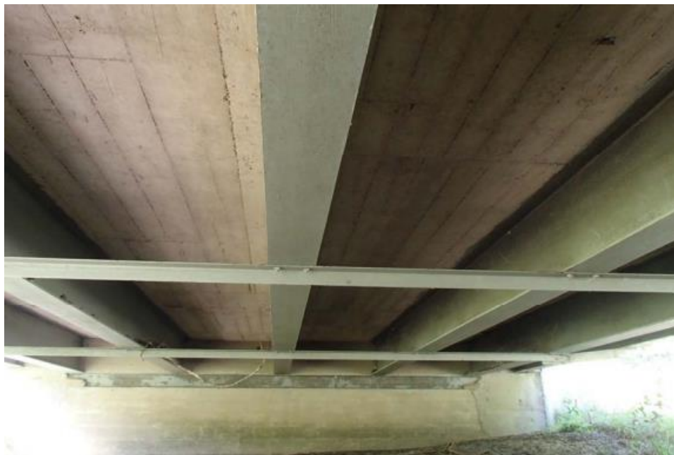
(c) Underside Superstructure View
