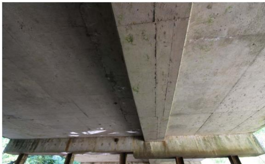
(c) Underside Superstructure View
