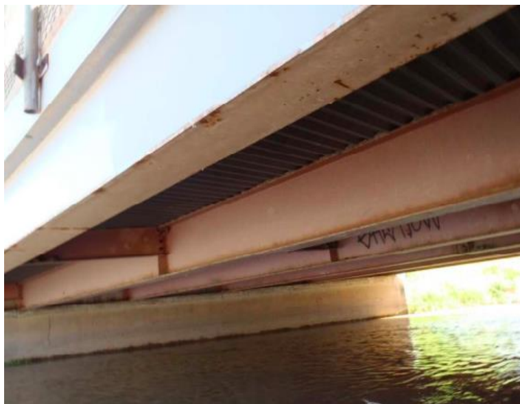
(c) Underside Superstructure View
