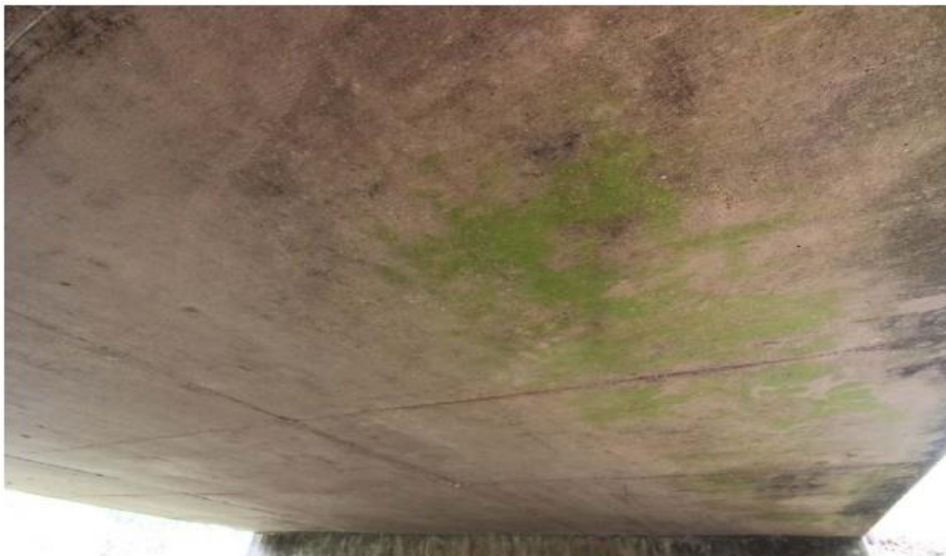
(c) Underside Superstructure View
