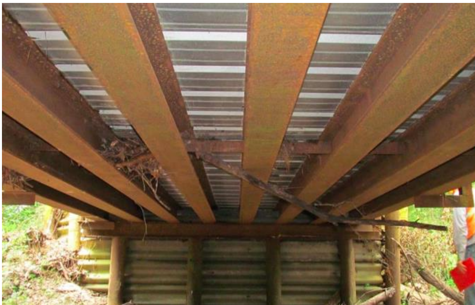
(c) Underside Superstructure View
