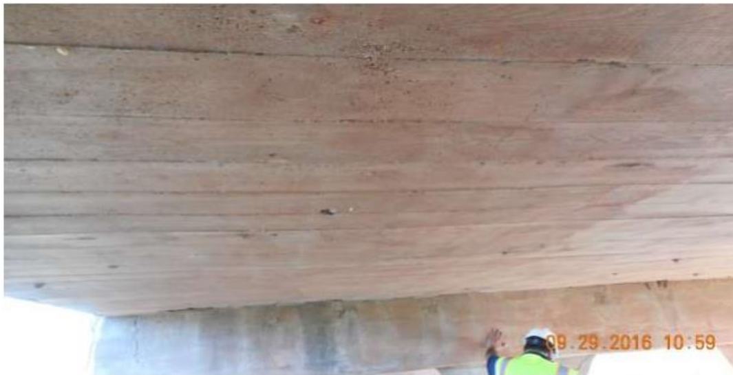
(c) Underside Superstructure View
