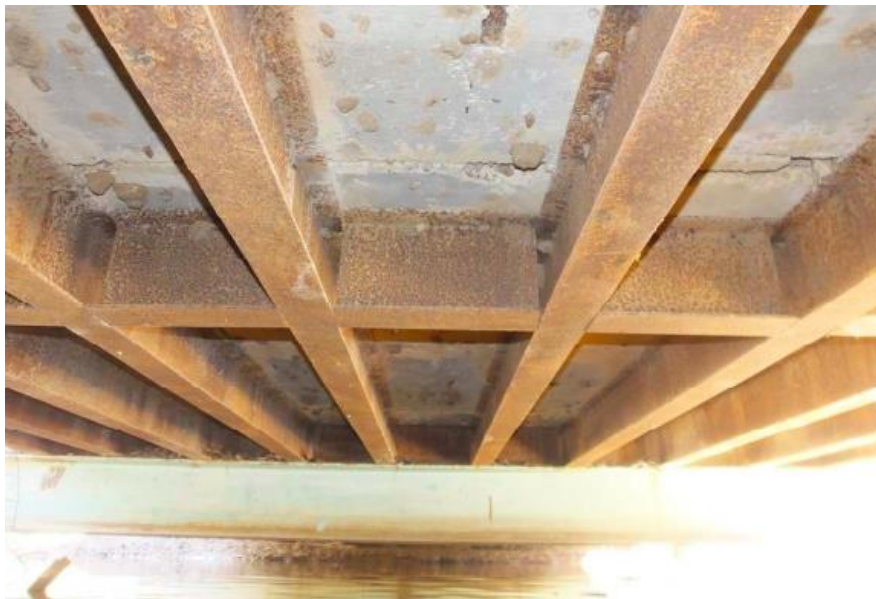
(c) Underside Superstructure View
