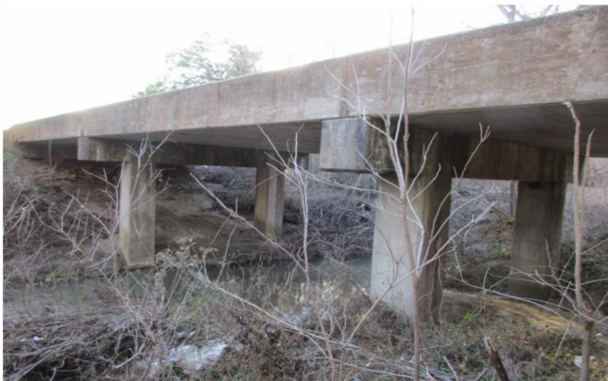
Figure C.17. Bridge CS-9 (TxDOT 2018c)
