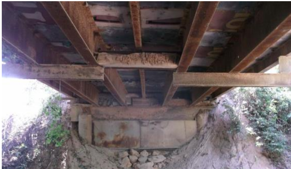
(c) Underside Superstructure View
