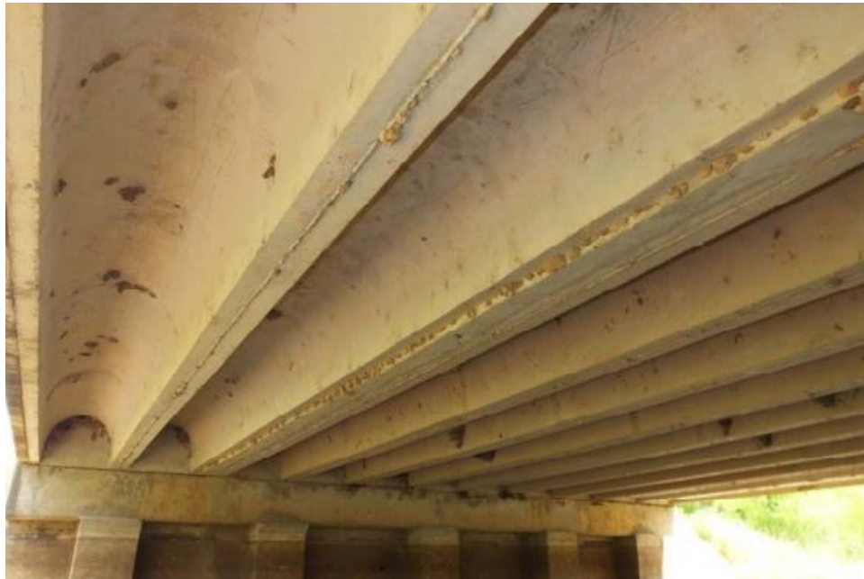
(b) Underside Superstructure View
