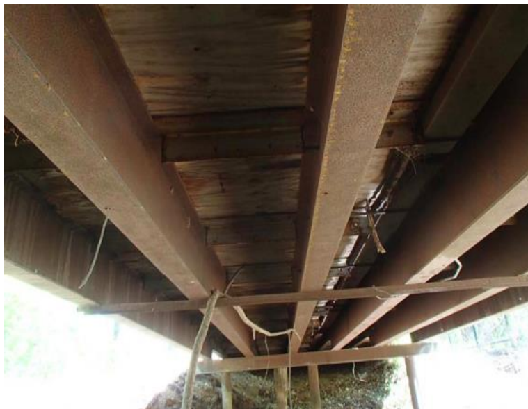
(c) Underside Superstructure View
