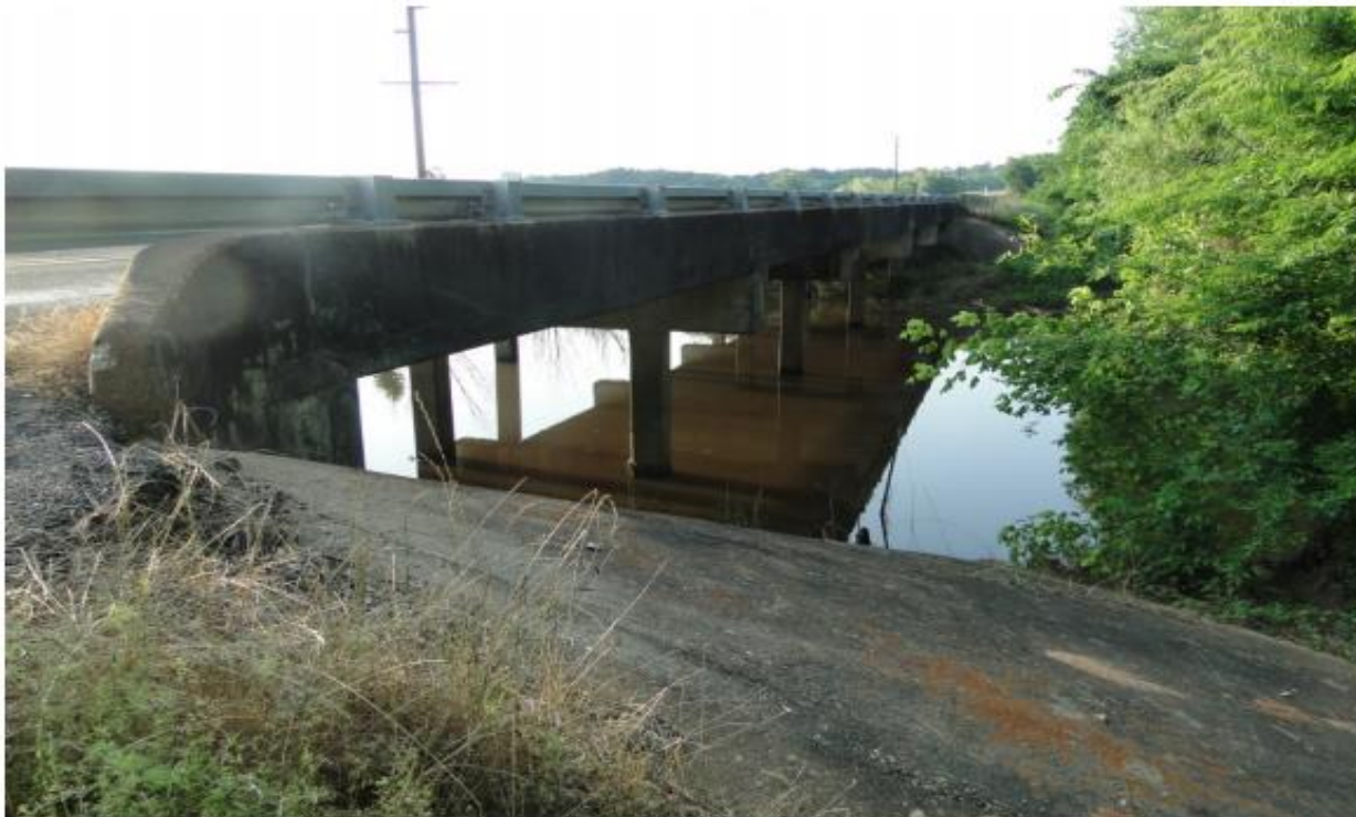
Figure C.29. Bridge CS-15 (TxDOT 2018c)
