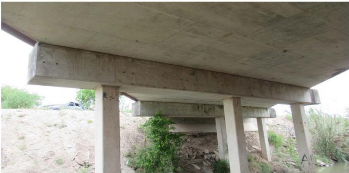
(c) Underside Superstructure View
