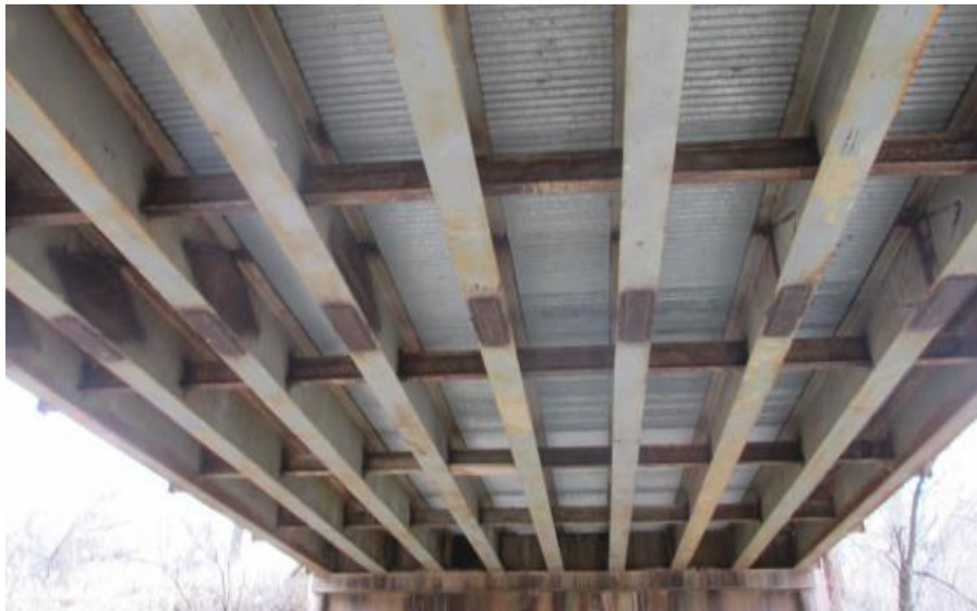
(c) Underside Superstructure View
