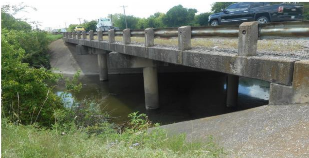
Figure C.21. Bridge CS-11 (TxDOT 2018c)
