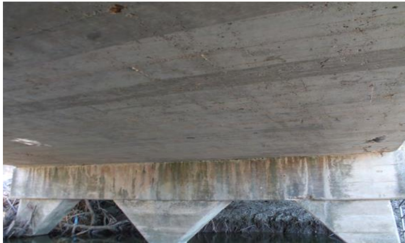
(c) Underside Superstructure View
