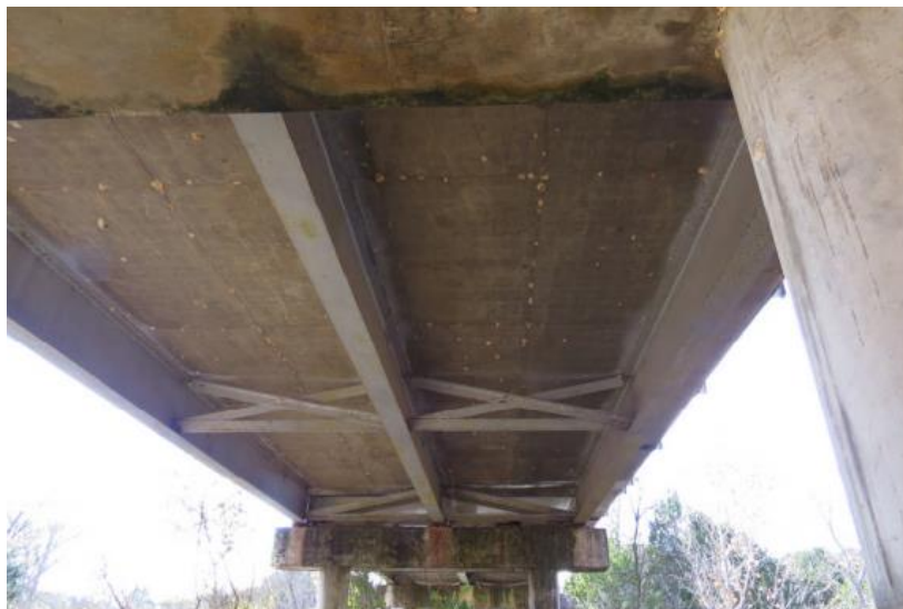
(c) Underside Superstructure View
