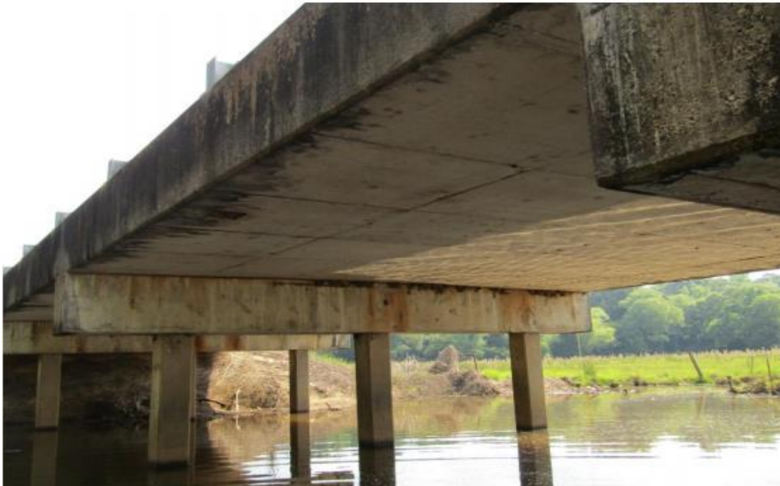
(c) Underside Superstructure View
