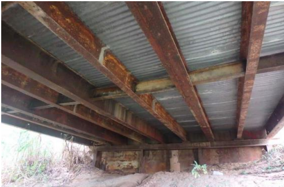
(c) Underside Superstructure View
