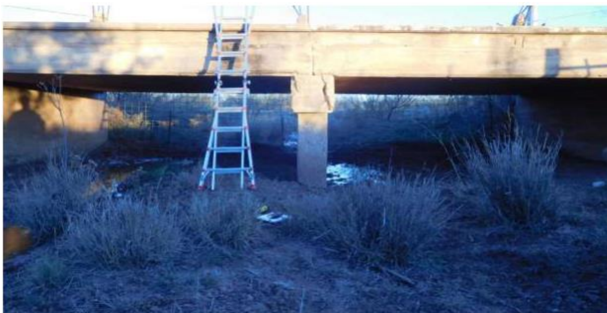
Figure C.3. Bridge CS-2 (TxDOT 2018c)
