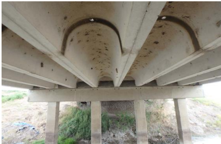
(c) Underside Superstructure View
