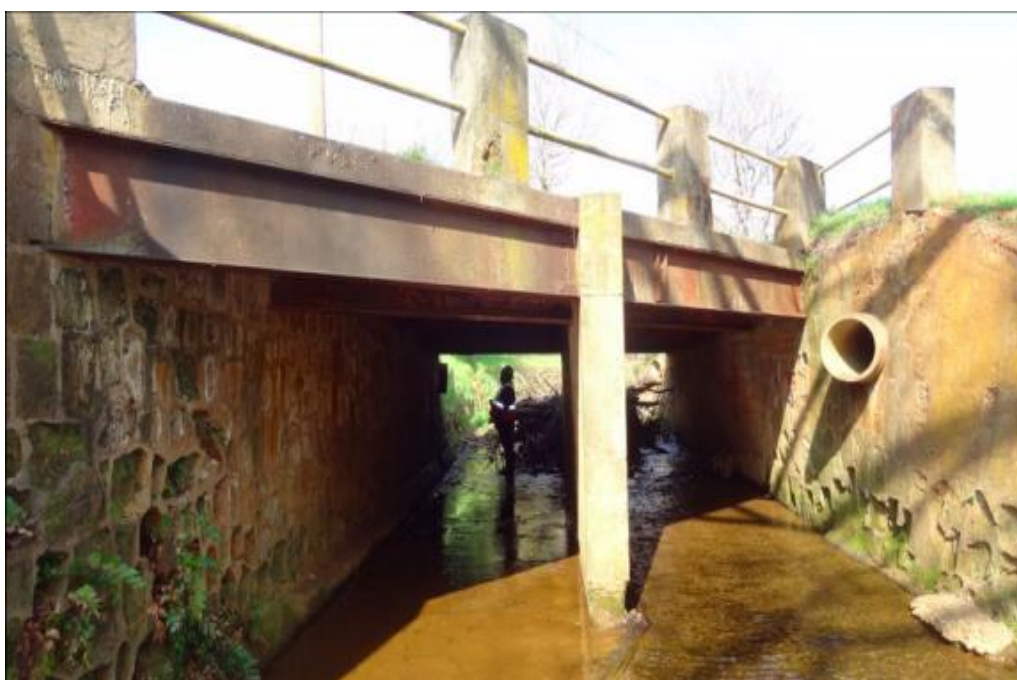
Figure B.25. Bridge SM-13 (TxDOT 2018c)
