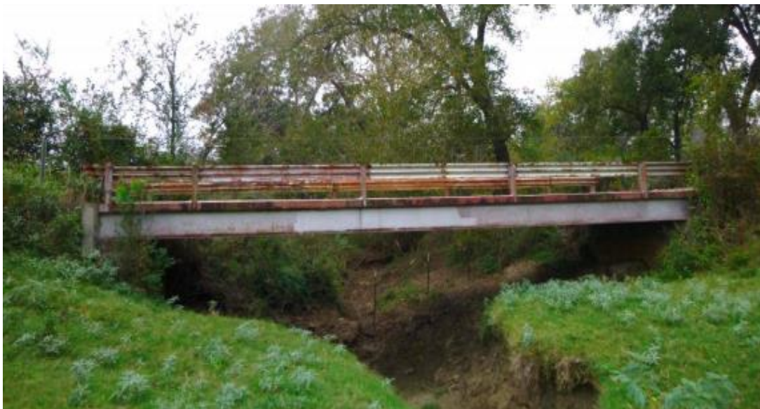
Figure B.45. Bridge SM-23 (TxDOT 2018c)
