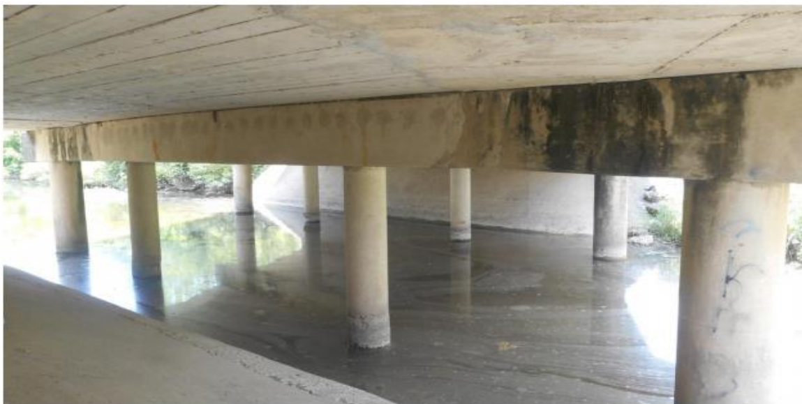
(c) Underside Superstructure View
