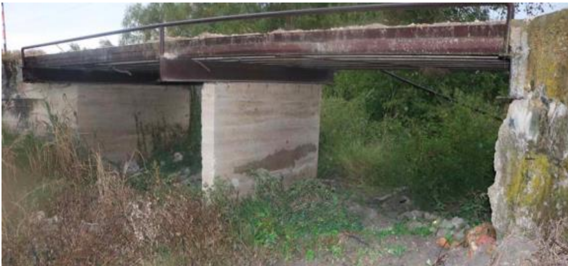
Figure B.51. Bridge SC-1 (TxDOT 2018c)
