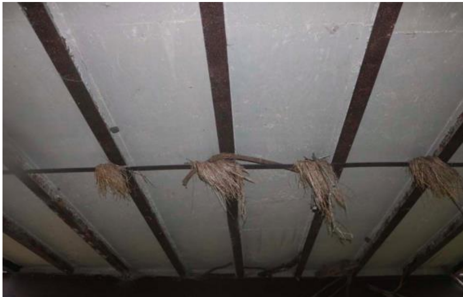
(c) Underside Superstructure View
