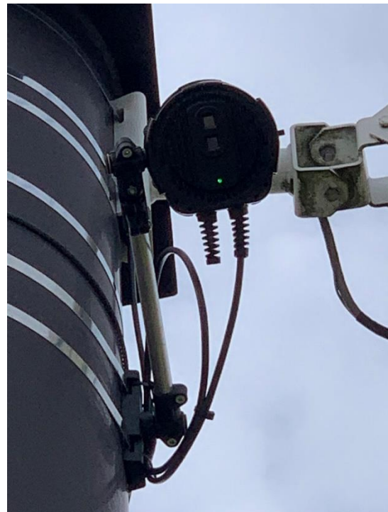
Figure 7. Location of FLIR Sensors on Traffic Pole.
