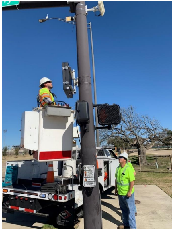
Figure 11. City of College Station Personnel Installing Equipment.
