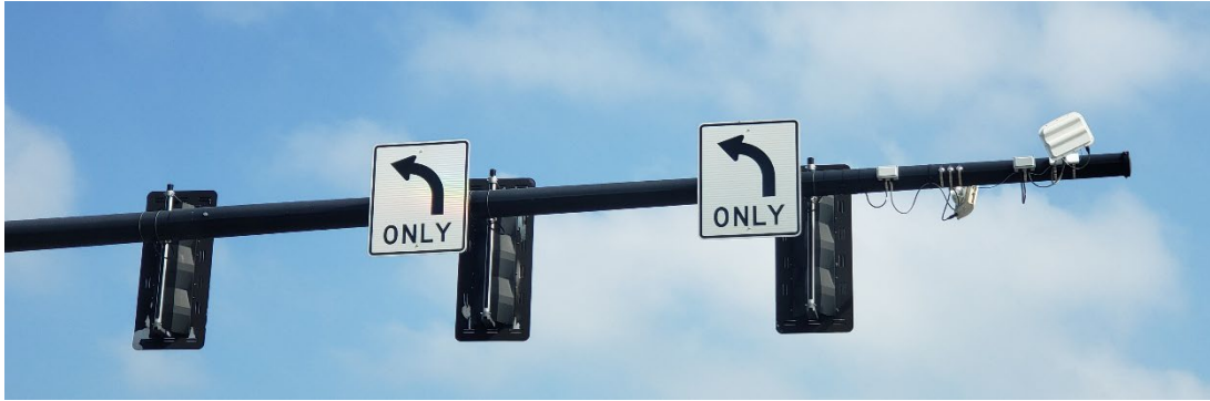
Figure 3: Example of Partial Aerodynamic Shielding on a Mast Arm
