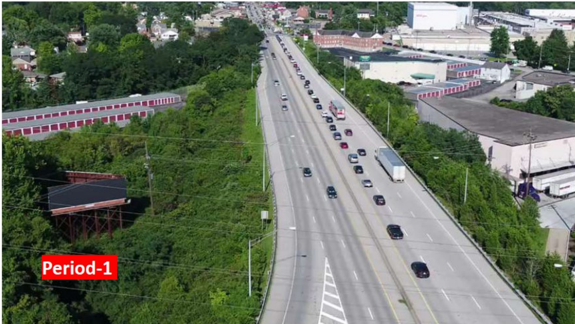
Figure 32: UAV image of built-up queues along US50 in Fairfax, OH area
