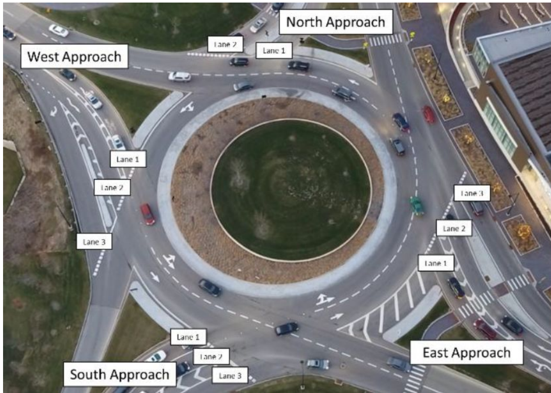
Figure 36: Multilane roundabout in Dublin, OH
