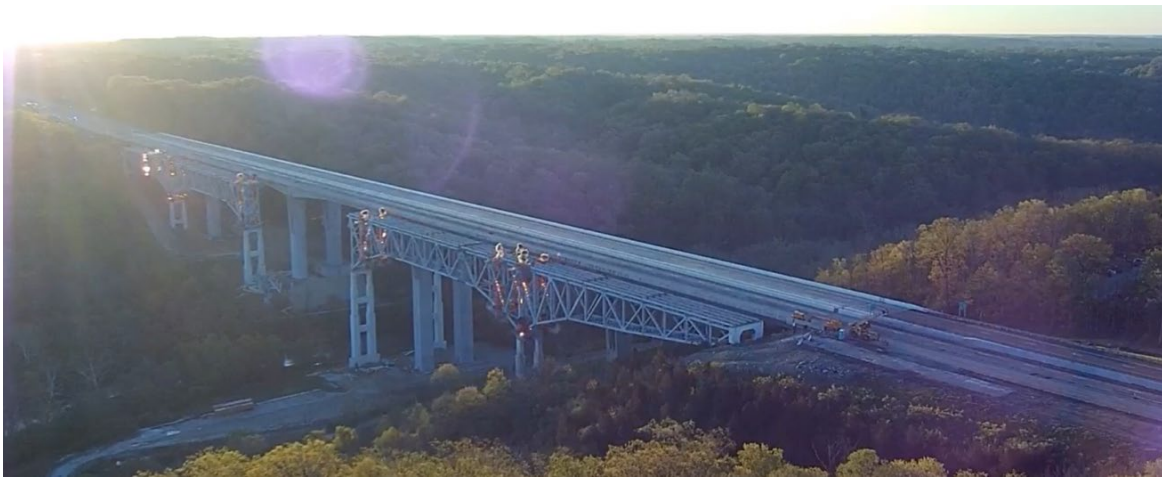
Figure 10: Demolition of Jerimiah Morrow Bridge
