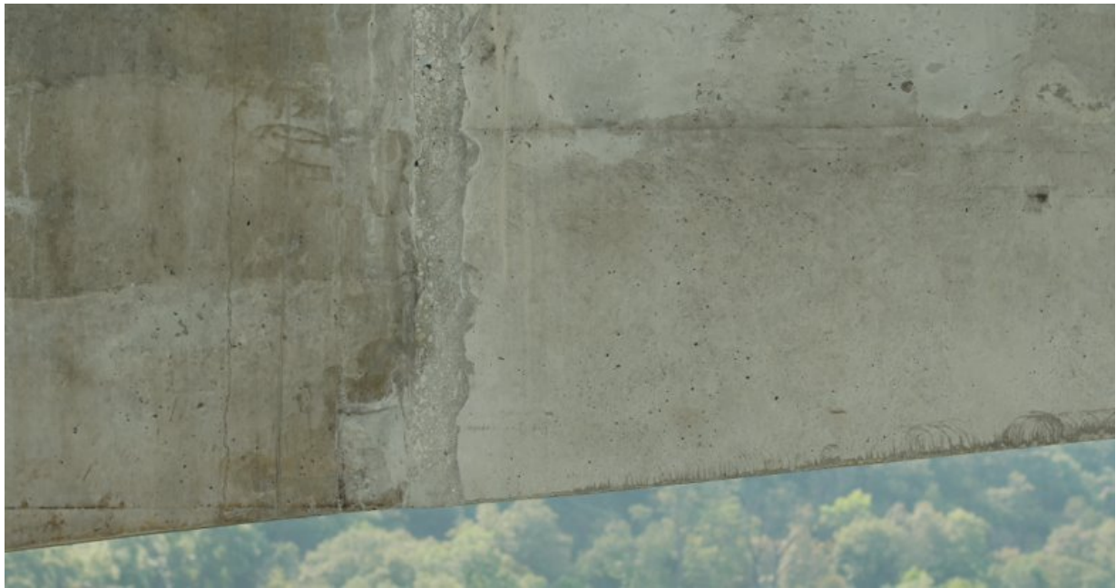
Figure 105: Example Image from Bridge Inspection
