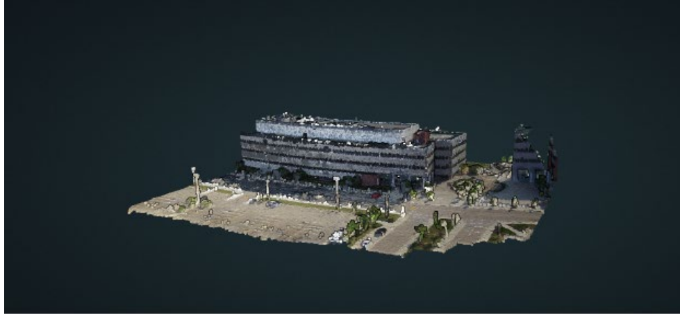
Figure 158: 3D point cloud of ODOT Headquarters, Columbus, OH
