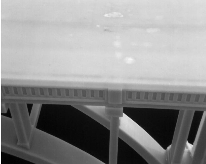
Figure 108: Thermal Delamination Example
