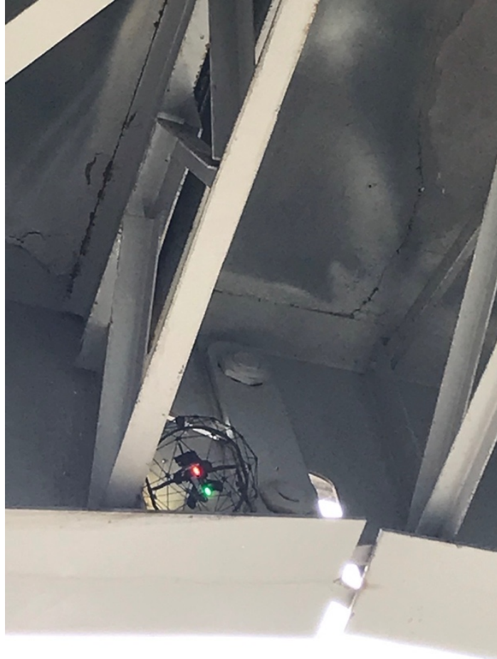
Figure 106: Flyability Elios Inspection of Expansion Joint
