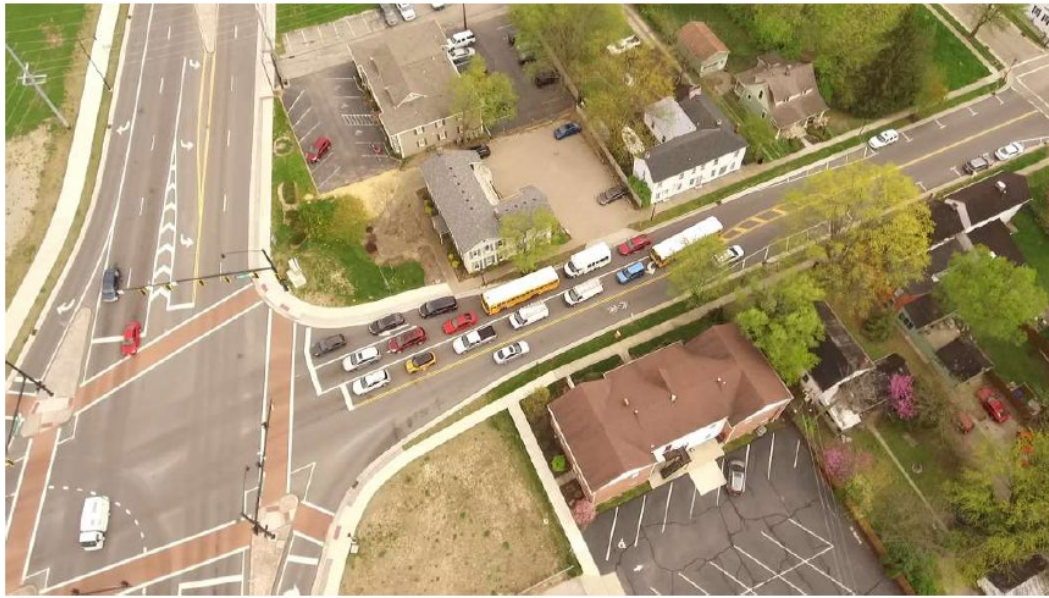
Figure 46: Site picture obtained by UAV at intersection of SR-714 and SR-73, northern terminus
