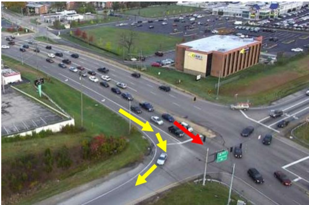
Figure 34: UAV image of signalized interchange along I-75 in Miamiisburg, OH area
