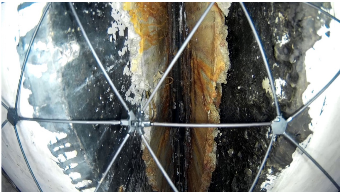
Figure 145: Bridge expansion joint and Elios close-up view
