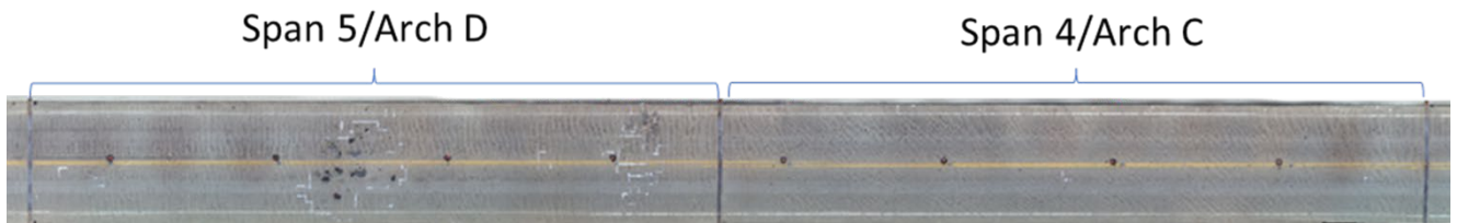
Figure 123: Visual 2D Orthomosaic of Fosters Bridge Deck
