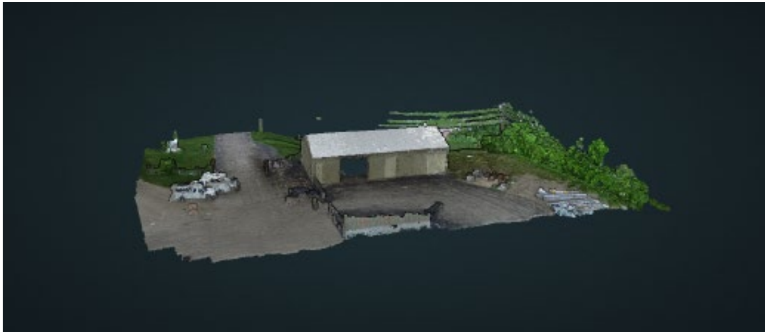
Figure 159: 3D point cloud of storage shed at ODOT District 8 Headquarters, Lebanon, OH
