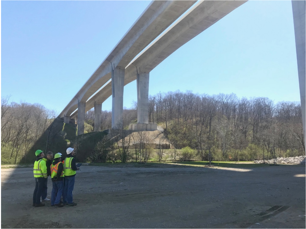
Figure 128: Bridge Inspectors during UAS Inspection
