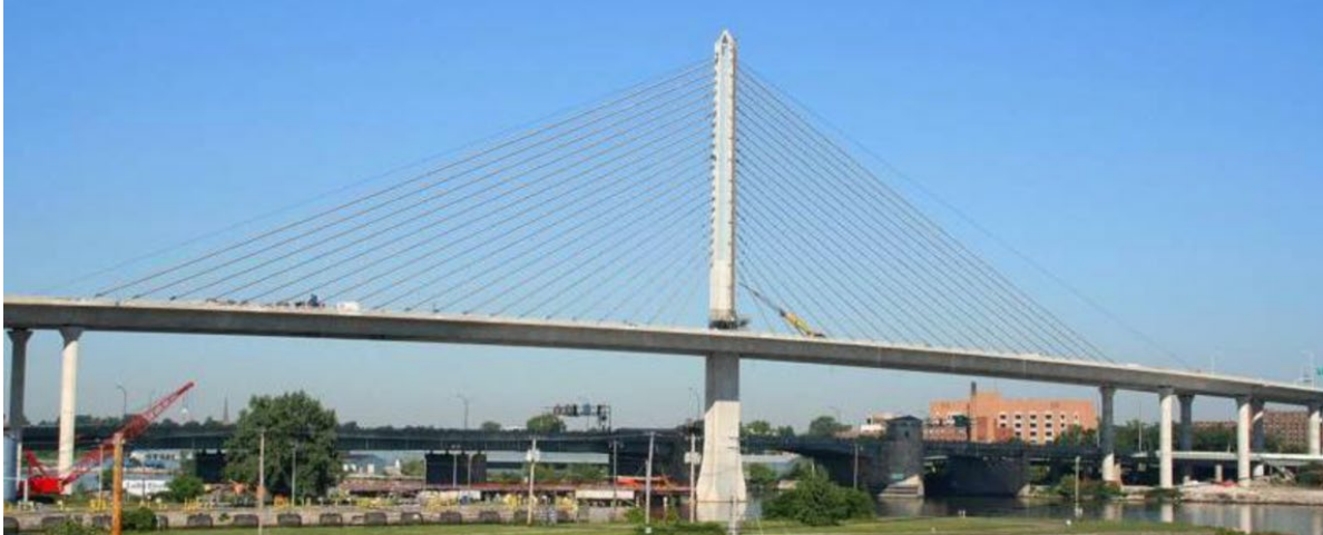
Figure 111: The VGCS Bridge in Toledo, OH
