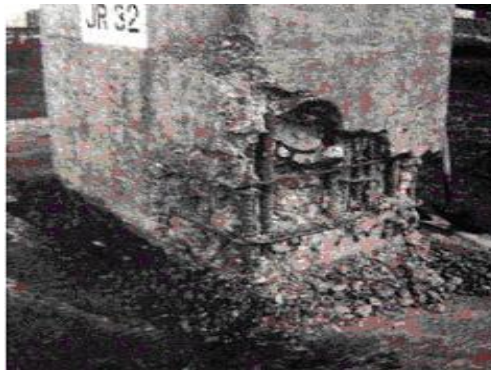
Figure 1-4. Lap splice failure at column base in the 1989 Loma Prieta earthquake (Priestley et al. 1996)
