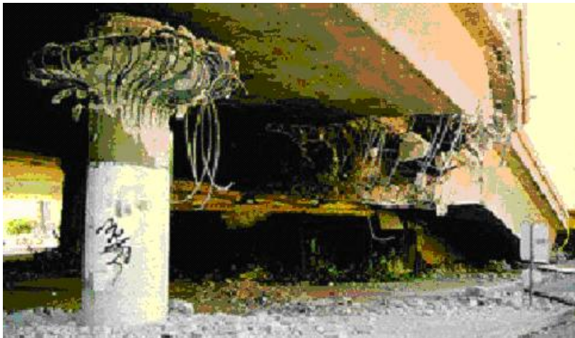
Figure 1-2. Example of damage to an existing bridge structure due to Northridge earthquake
