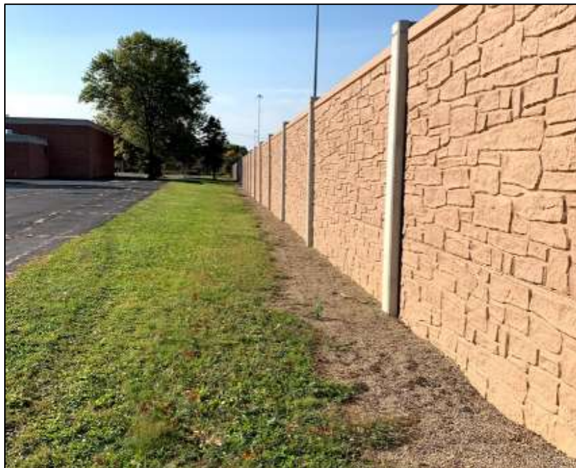
[b] General View, YMS Site, After Barrier Construction
