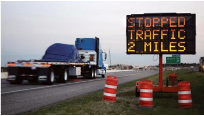
Advance warning signs and queue warning systems are useful in alerting traffic to downstream conditions during rolling roadblock operations. (Source: TTI)
