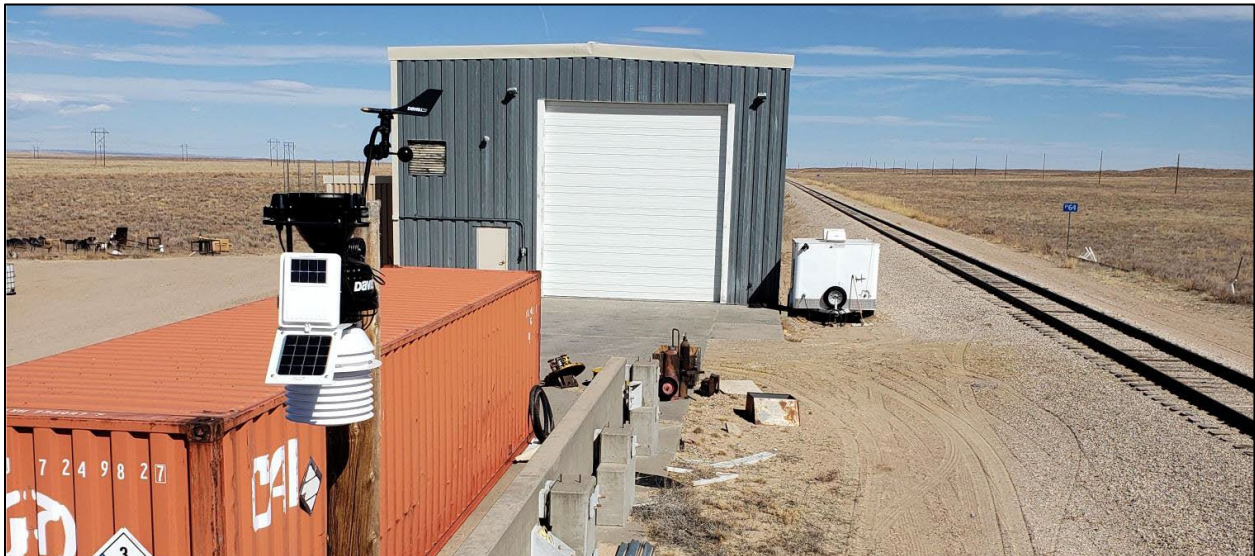
Figure 8. Weather Station and Trailer that Holds Desktop Node Equipment at Post P64 of the PTT
