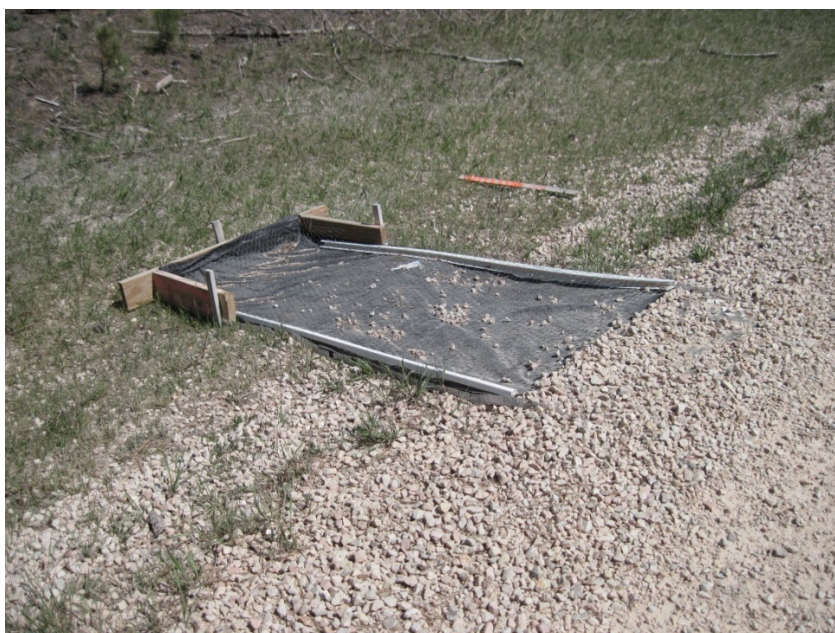
Figure 10: Cast-off collection box located in Custer County.
