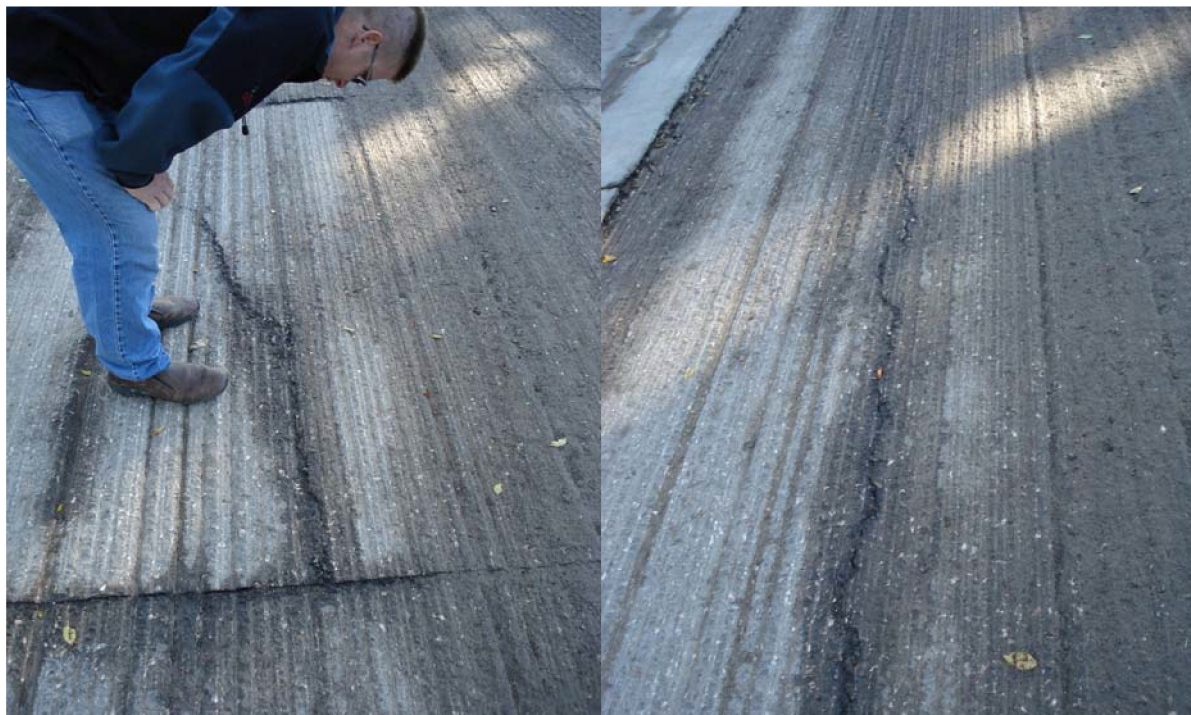
Figure 2-4: Conducting the distress survey with typical crack.
