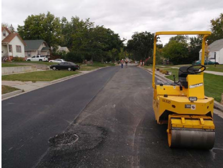
Figure 2-7: Compaction of fiber reinforced HMA with conventional paving equipment.
