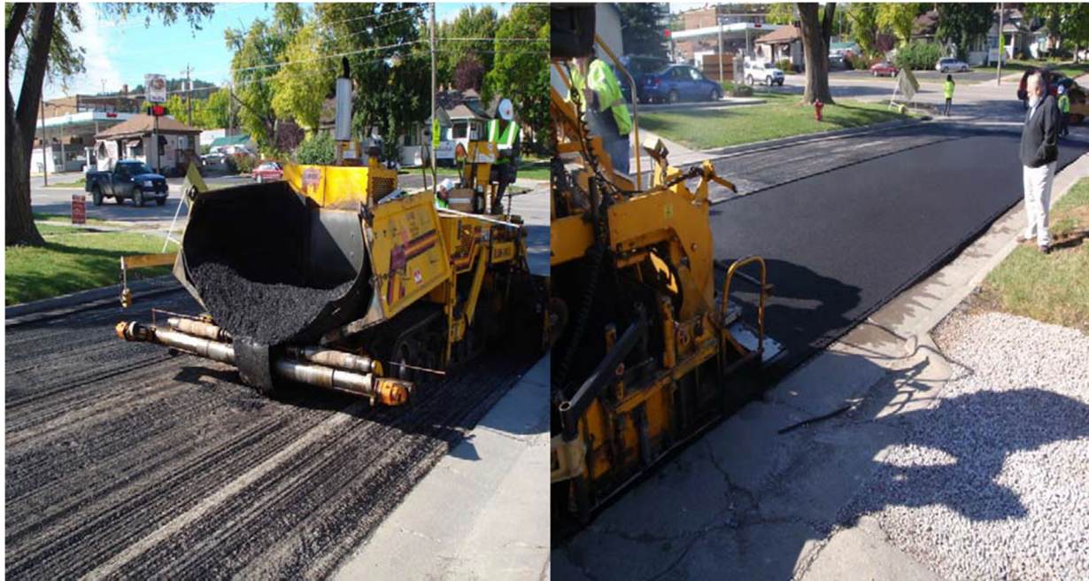
Figure 2-6: Placement of fiber reinforced HMA with conventional paving equipment.
