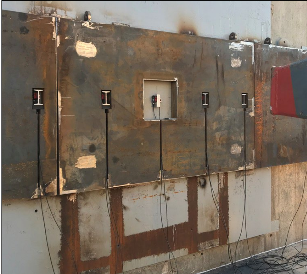
Figure 19. Lasers Displacement Transducers on Crash Wall
