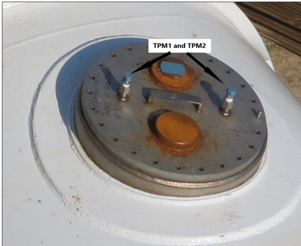
Figure 16. Tank Car Pressure/Temperature Transducer Locations (manway)
