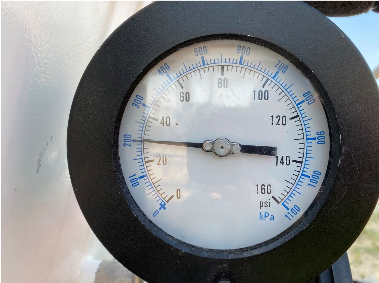
Figure 40. Mechanical Pressure Gauge Prior to Test
