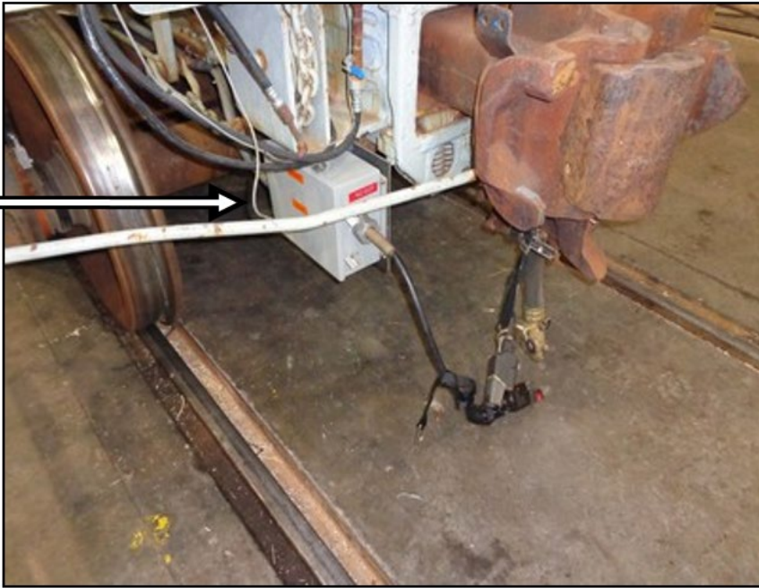
Figure 13 – EPSS junction box on the B-end of the hopper car
