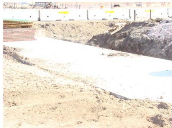
(b) Backfill around the Structure
