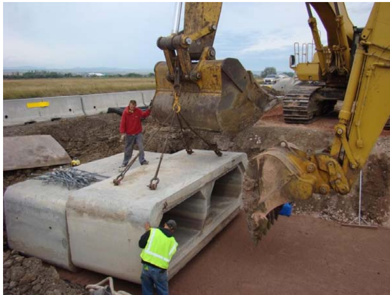
Figure 8.5: Assembly of the Precast Units of Structure #52-485-337
