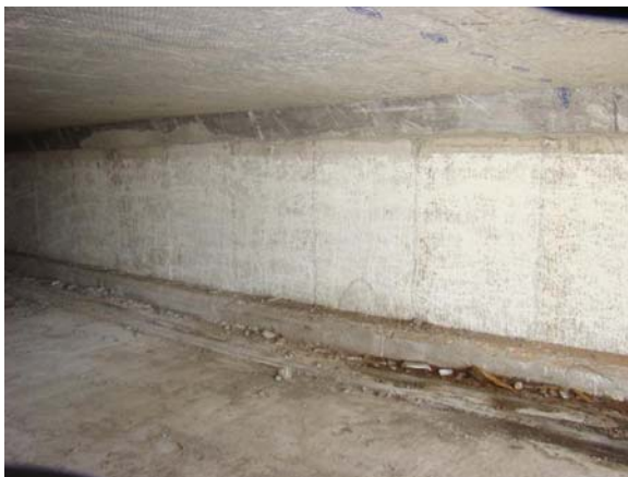
(a) Finished Wall Interior Surface
