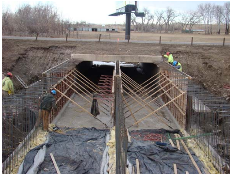
Figure 8.6: The Extension of Structure #52-489-339 under Construction
