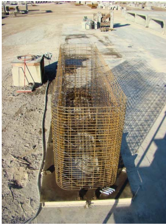
Figure 8.1: Reinforcement Cage of an SCC Box Culvert Unit
