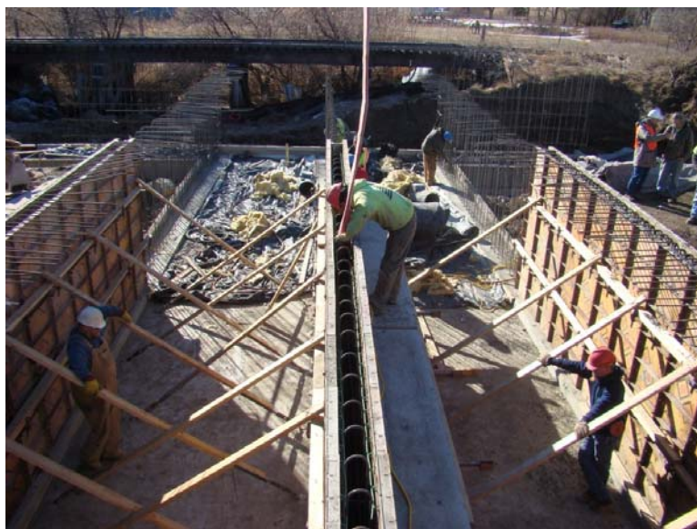
Figure 8.8: Casting of the SCC Mix in Structure #52-489-339
