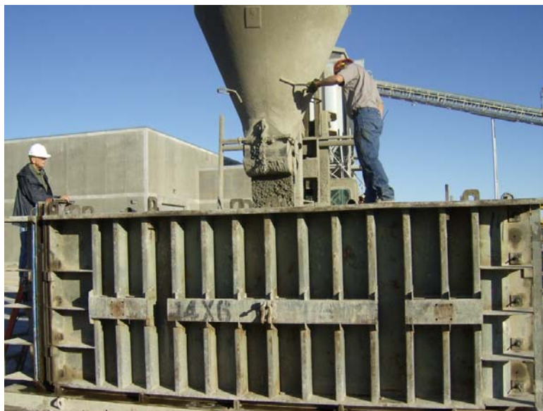
Figure 8.2: Casting of an SCC Box Culvert Unit
