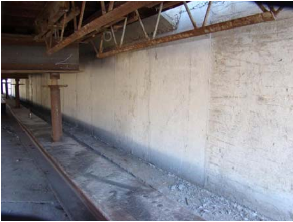
(a) Finished Wall Interior Surface
