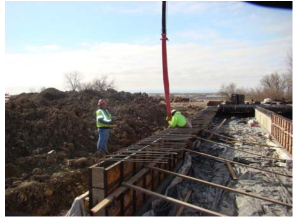
(b) Concrete Placement
