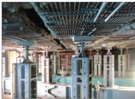
(a) Soffit before Repairing
