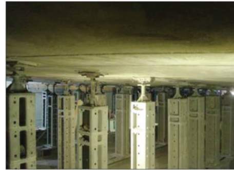
(b) Soffit after Repairing
