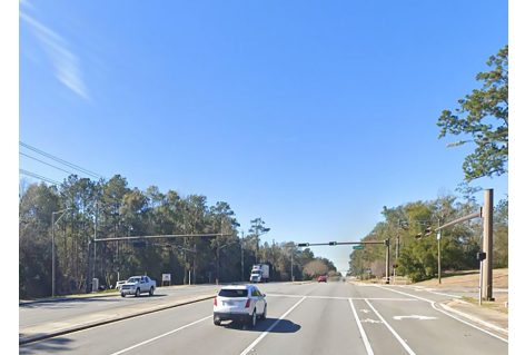
One of the 22 intersections on US-90 (Mahan Drive) which were part of the project.
