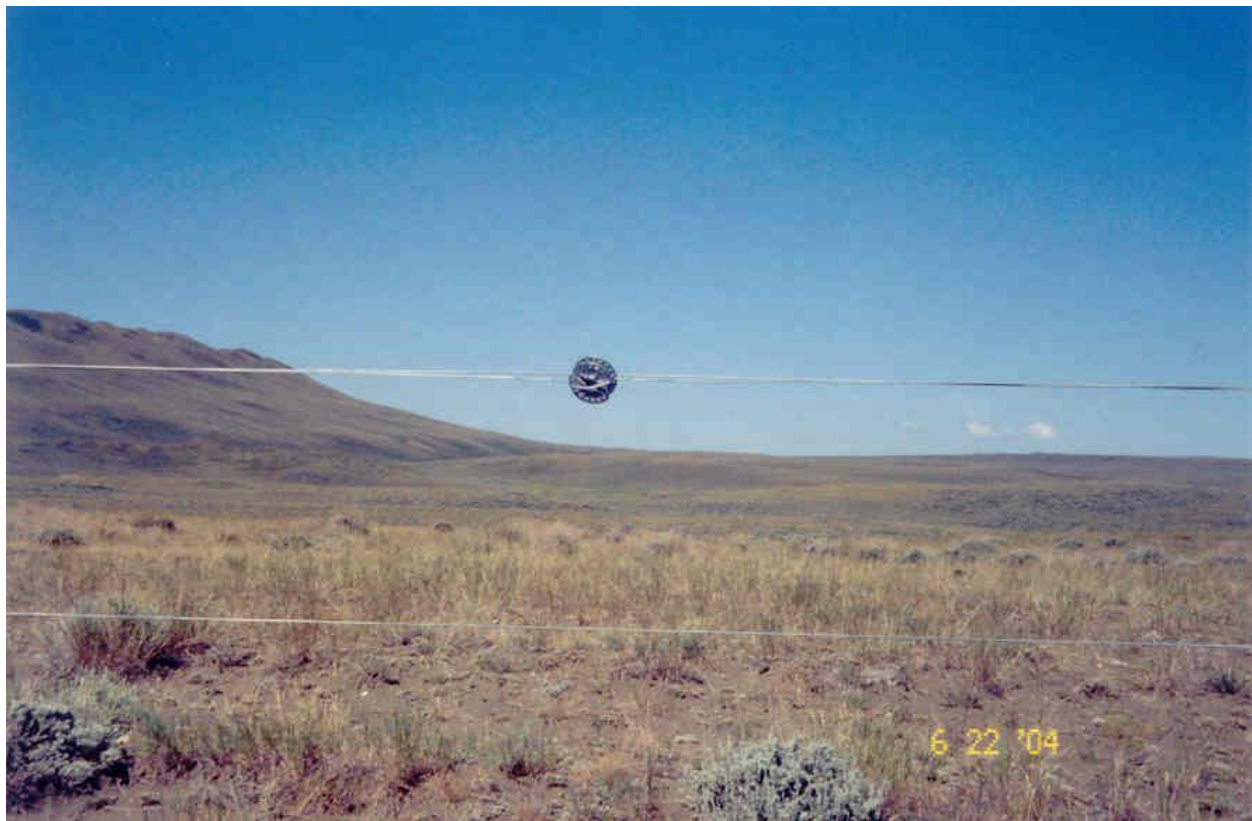
Figure 5. Two wires caught around a wire tightener causing a short.
