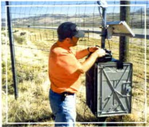
Matt Johnson installs the controller and transmitter for the Geophone scopes on the north side of the crossing zone.
