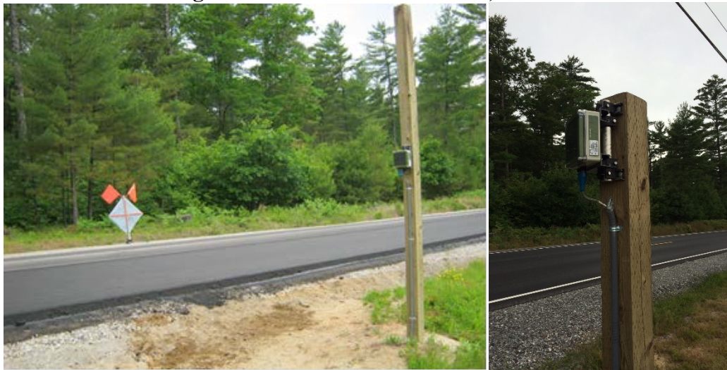
Figure 6. Waterford Instrumentation Site during PM RAP installation (left) and final (right)
