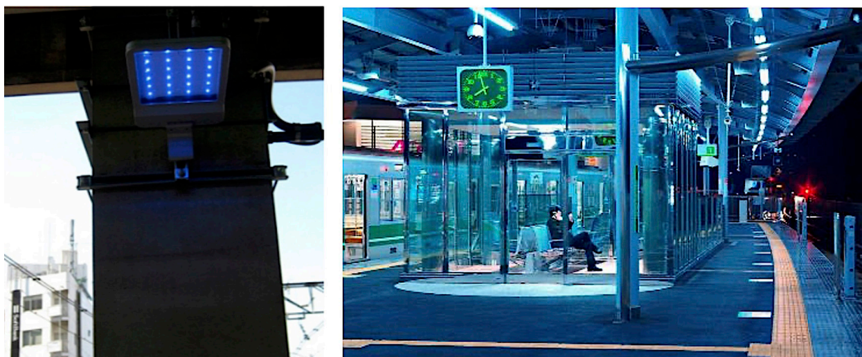
Figure 3-19 Suicide prevention – blue LED lights in Japan railroad station platforms
