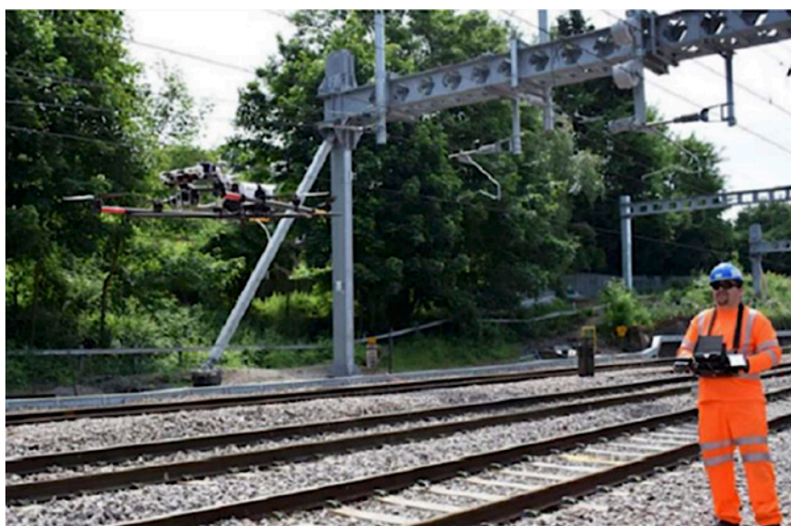
Figure 3-10 Trespasser detection – aerial drones
