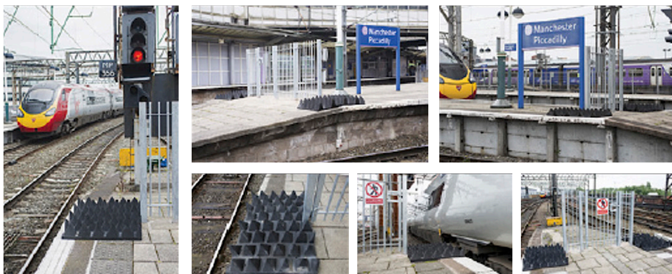
Figure 3-4 Trespasser detection – anti-trespass grids
