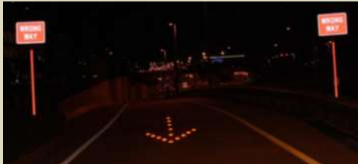
Red Reflective Tape on Sign Posts, Signs on Both Sides of Ramp (Source: Ouyang, 2013)
