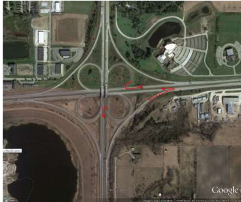
Wrong-Way Movements Observed at Interchange Entrance Ramps (Source: Iowa DOT)
