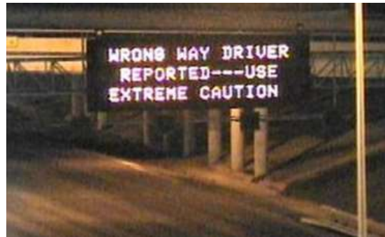
Current Message Posted to Oncoming Right-Way Traffic (Source: TxDOT)
