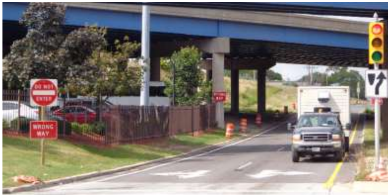
Additional WW and DNE Signs & Signs Mounted on Same Post (Source: Wisconsin DOT)
