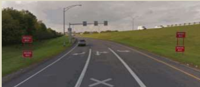
Signs on Both Sides of Ramp; Two Signs on the Same Post (Source: Provided by Ohio DOT)
