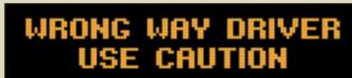
DMS Message to Alert Oncoming Right-Way Traffic
