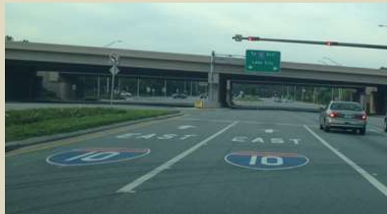
Route Designation Shield with Straight Arrow (Source: Provided by FDOT)
