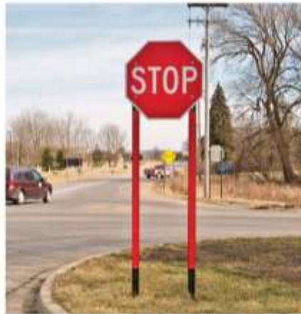
Red Reflective Sheeting on Sign Posts (Source: Morena and Leix, 2012)
