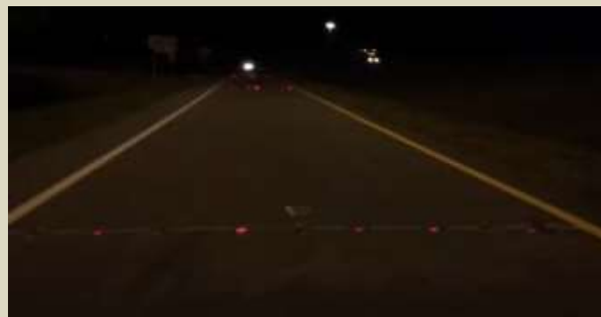
Internally Illuminated Raised Pavement Markers Create Illusion of Stop Bar (Source: Provided by Florida DOT)
