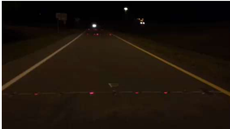
Internally Illuminated Raised Pavement Markers Create Illusion of Stop Bar (Source: Florida DOT )
