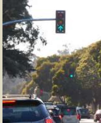
Straight Arrow Indication near Exit Ramp (Source: Provided by Rhode Island DOT)
