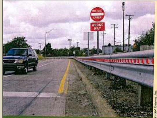
Red Delineators on Guardrail along Exit Ramp
