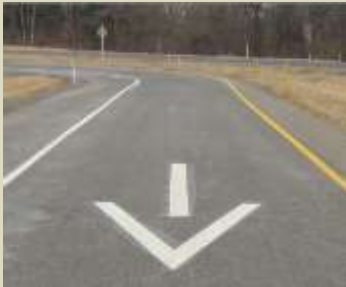
Wrong-Way Arrows at Exit Ramp (Source: Tobias, 2015)
