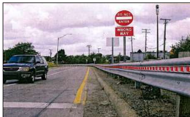
Red Delineators on Guardrail along Exit Ramp (Source: Morena and Leix, 2012)
