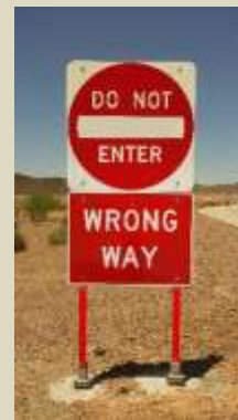
Oversized Signs, DNE and WW Sign on Same Post (Source: Provided by Arizona DOT)
