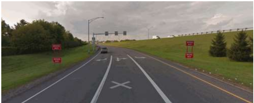
Two WW Signs on Same Post, Both Sides of Ramp, Red Reflective Tape on Posts (Source: Ohio DOT)
