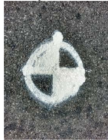
Figure 4-8 Painted Target with PK Nail in center
