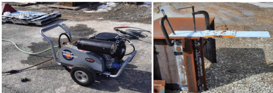
Figure 4.18 Pressure washer and pack rust removal set up.
