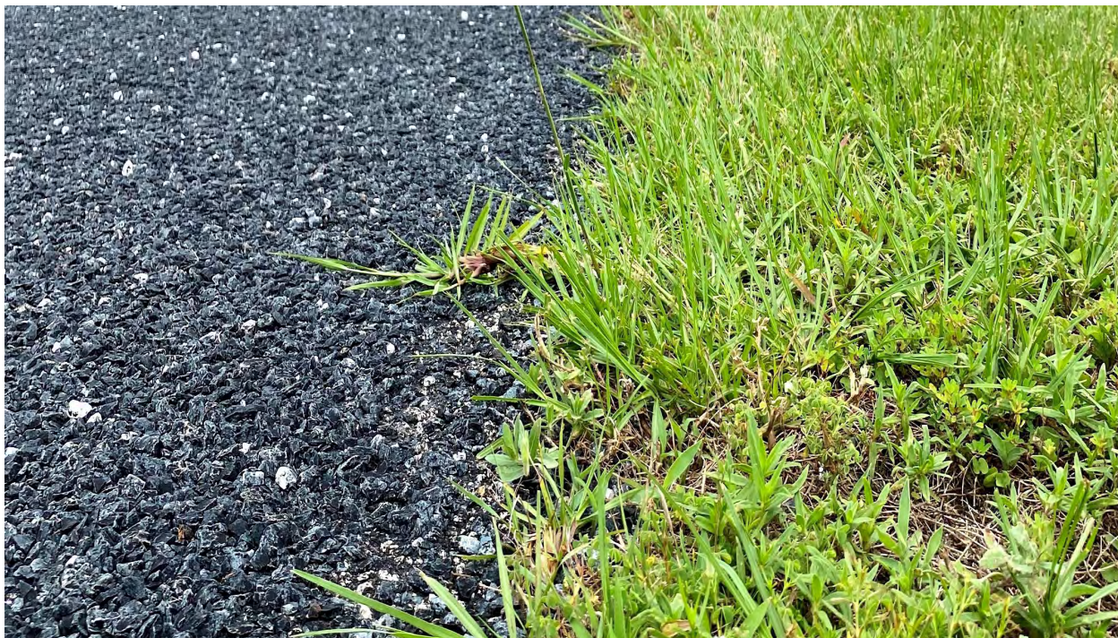
Figure 36: Weeds Sticking Out into Roadway, Which Caused Shuttle Disengagements
