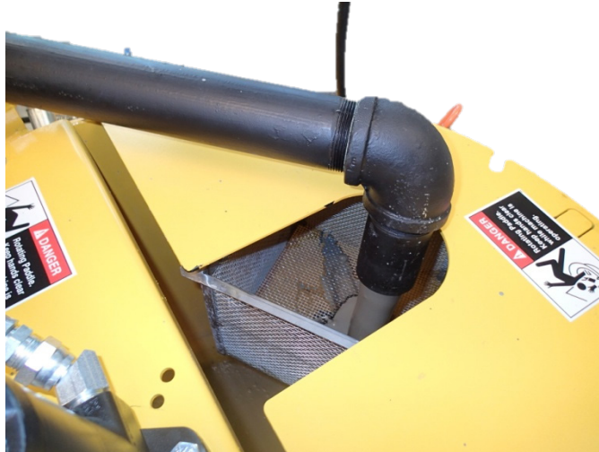
Figure I-4 Transfer the grout to the agitation tank
