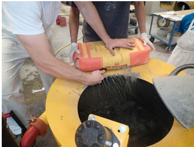
Figure I-3 Add one bag of grout at a time
