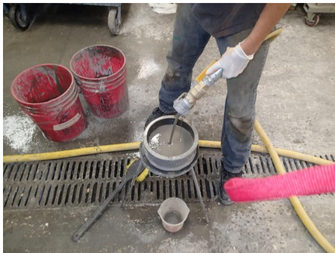
Figure I-5 Pump grout to target.
