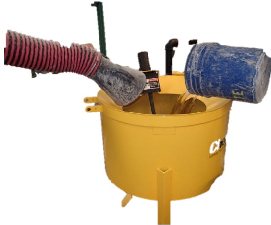
Figure I-2 Add water to mixing basin.
