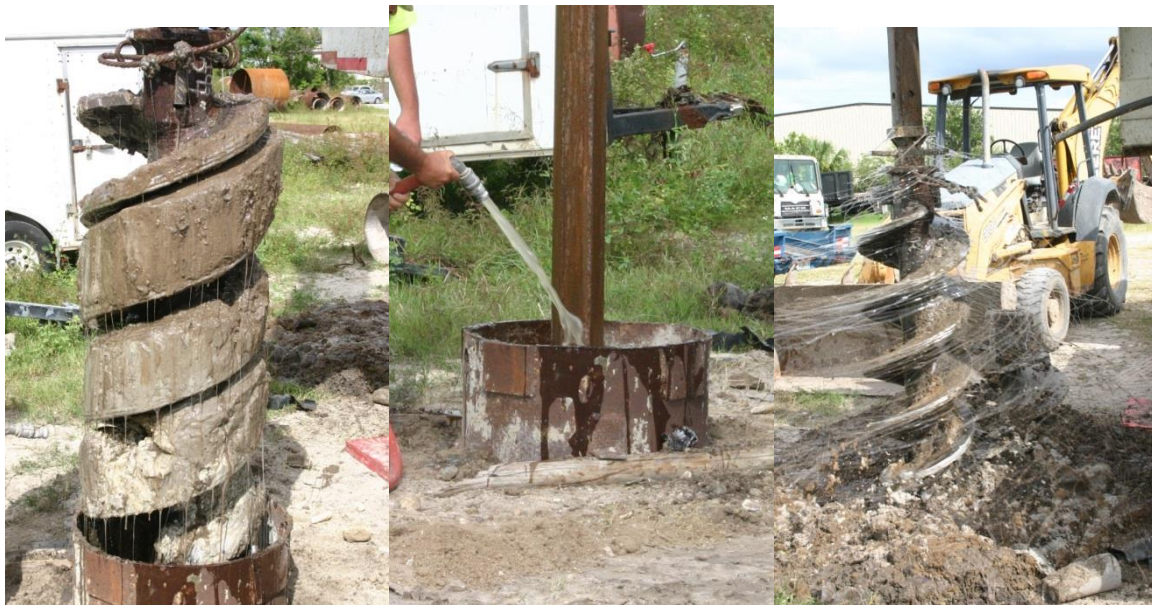
Figure 4.14 Auger extraction (left), slurry replacement (center), and polymer strings during auger spin off (right) of Shaft P0-100.
