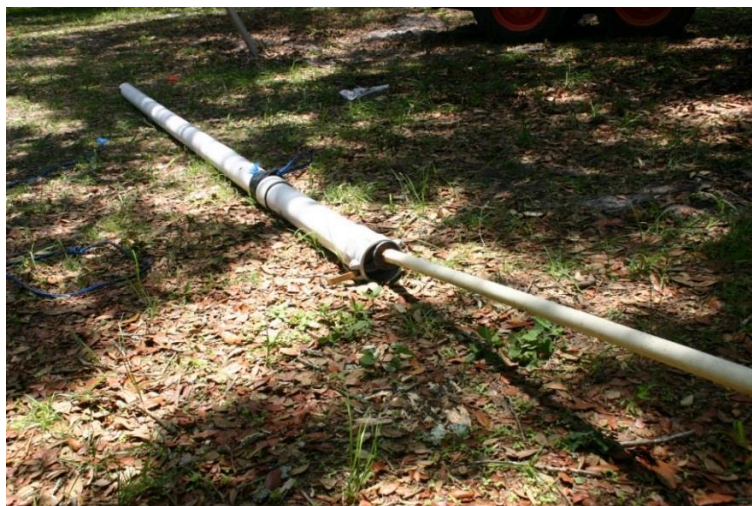
Figure 3.46 Sheathed all-thread inserted into the tremie.
