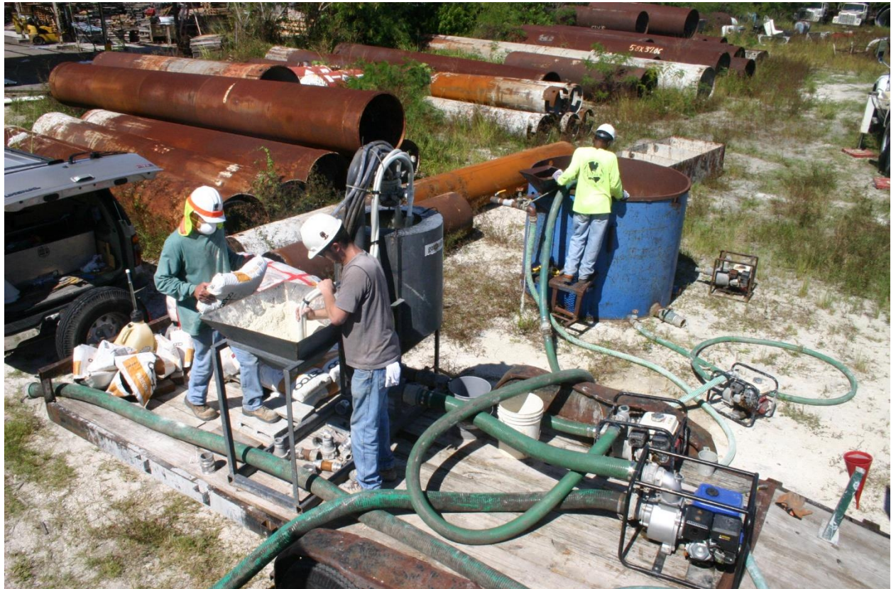
Figure 4.8 Multi-educator mixing system used to prepare slurry.
