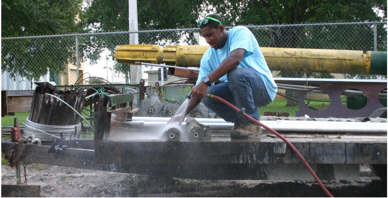
Figure 3.58 Filter cake removal of shaft quarters.
