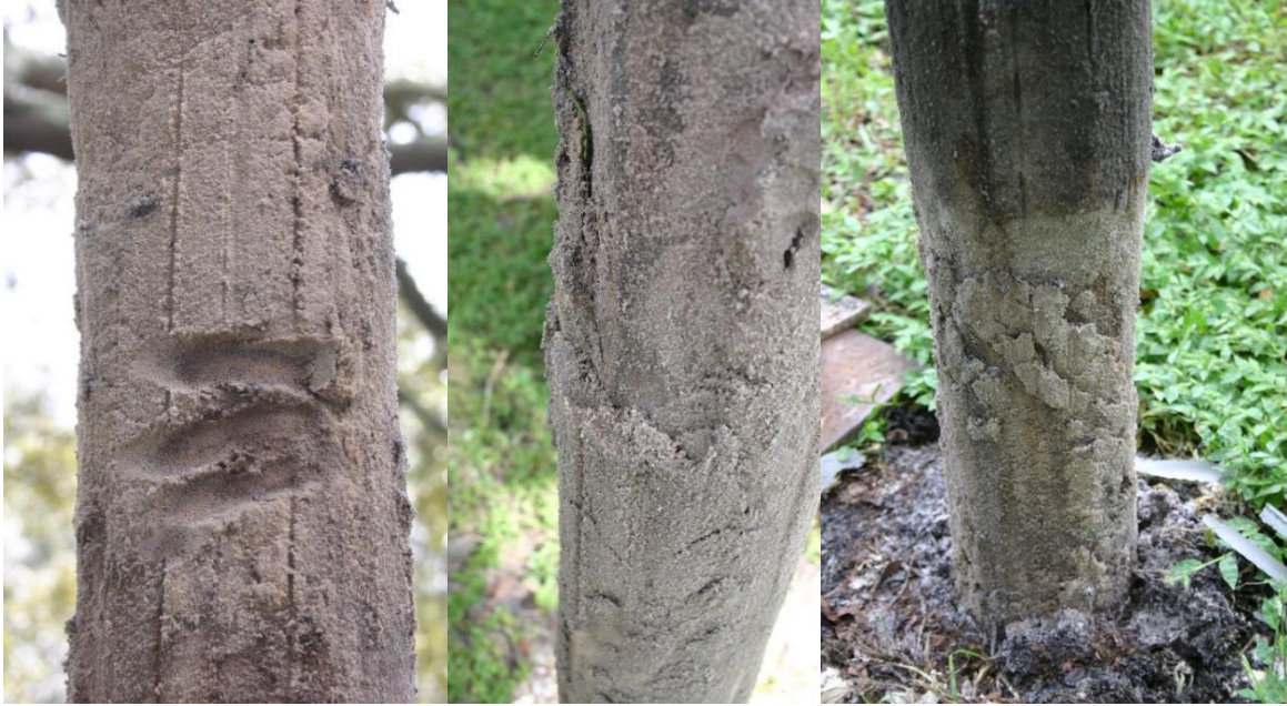
Figure 3.89 Layer of soil on perimeter of cetco polymer shafts.
