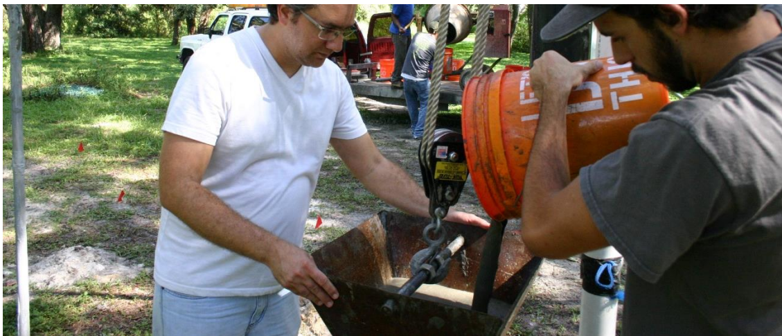
Figure 3.87 Bucket of mortar transferred to hopper.
