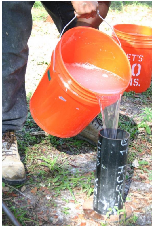
Figure 3.61 Introduction of KB International Enhanced CDP polymer into borehole.
