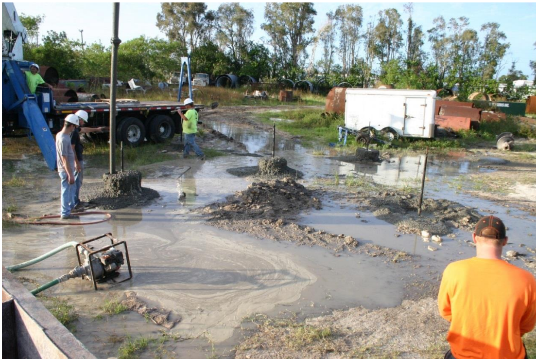
Figure 4.22 Concreting of final shaft.
