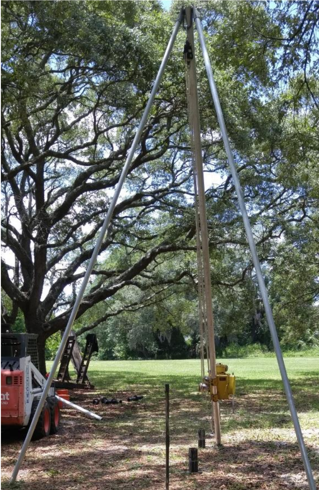
Figure 3.20 Tripod and hoisting system.
