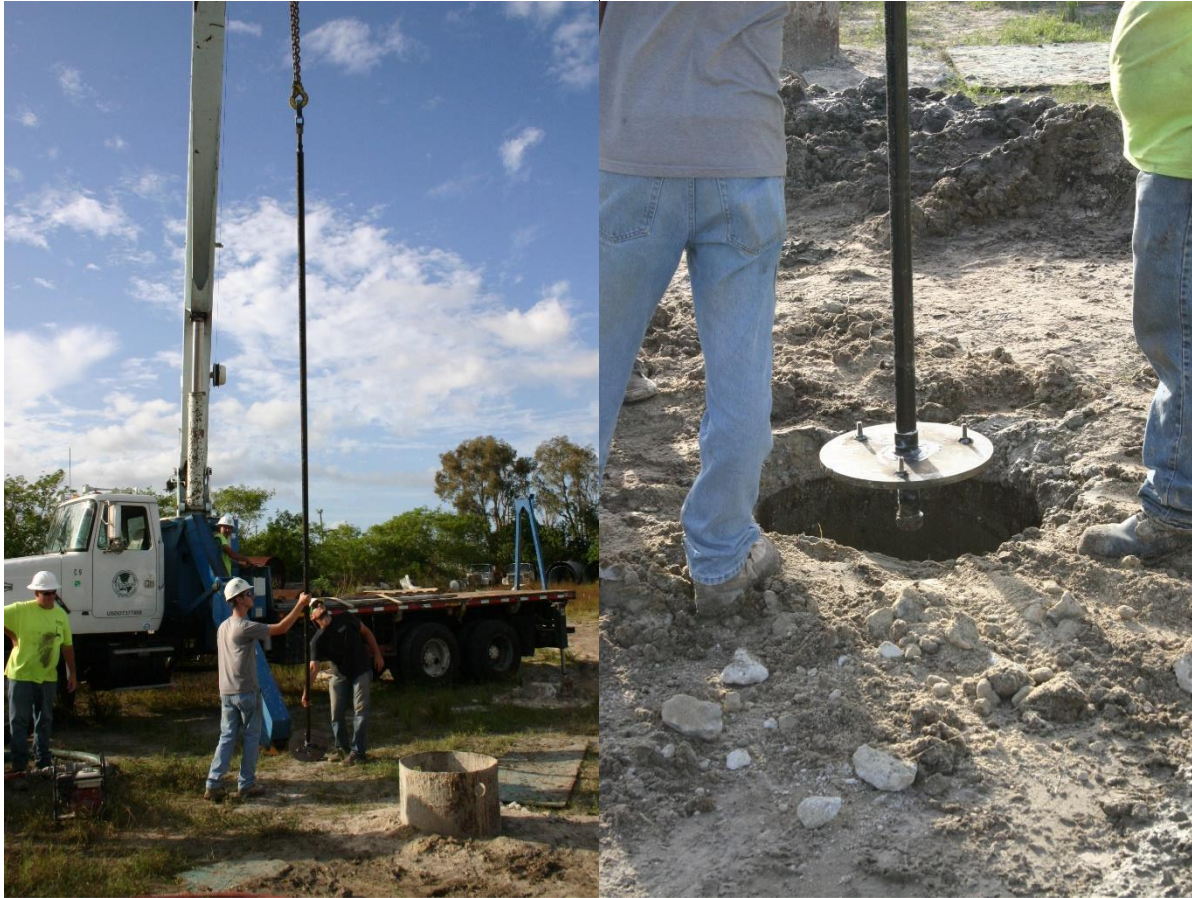
Figure 4.20 Anchor rod installation.
