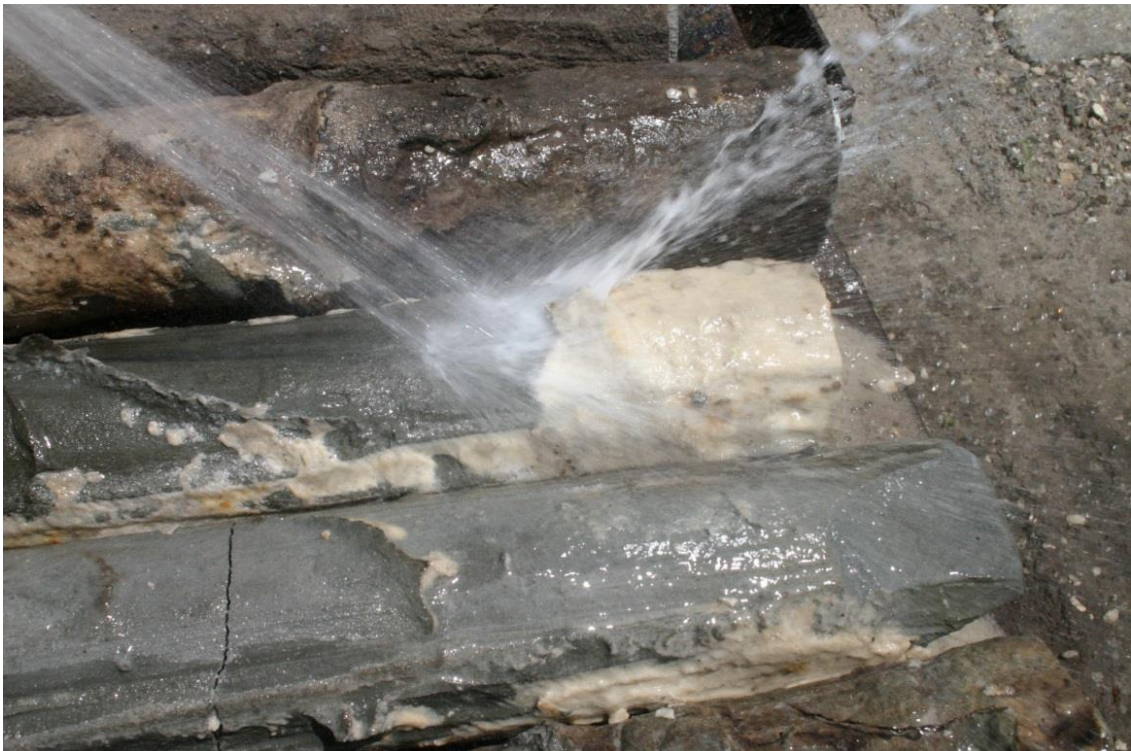
Figure 3.73 Removal of soil in lower portion of KB polymer shafts.
