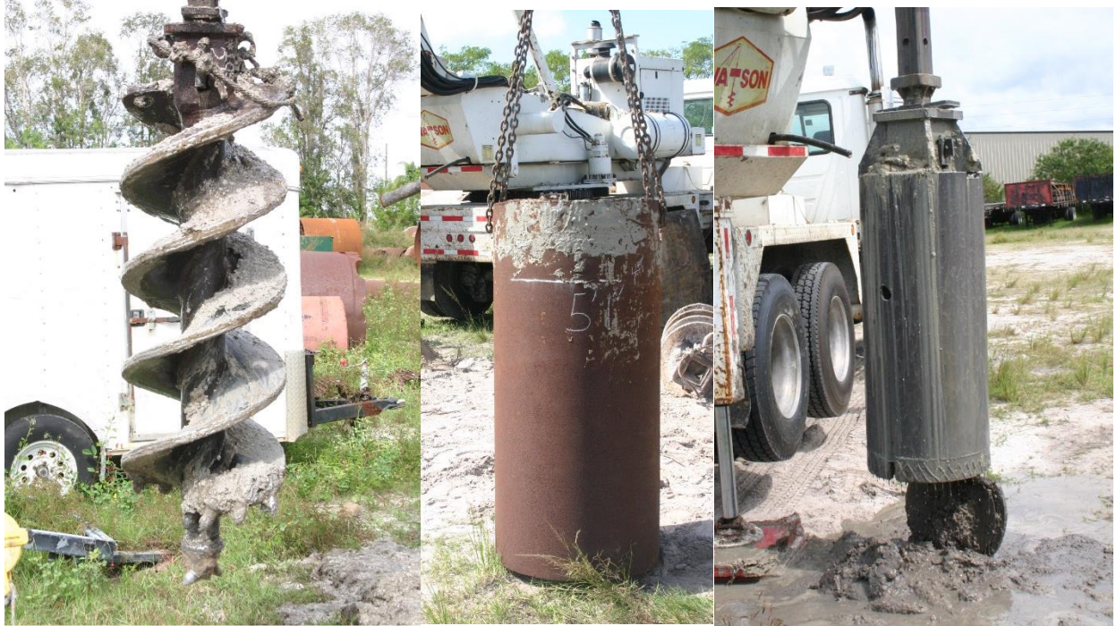
Figure 4.12 Excavation tools – auger (left), surface casing (center), and clean-out bucket (right).
