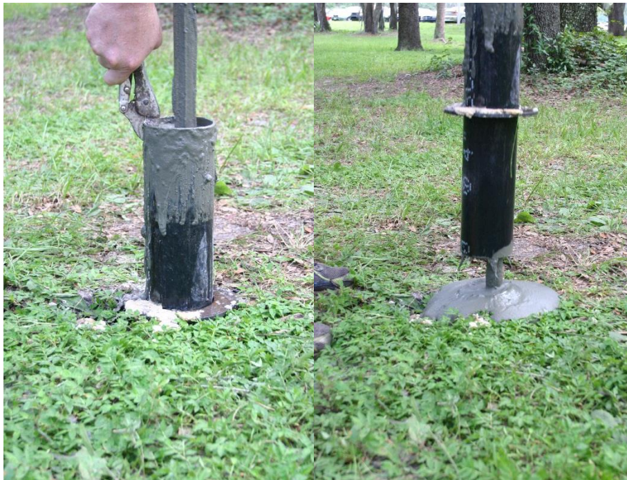
Figure 3.49 Removal of temporary surface casing.
