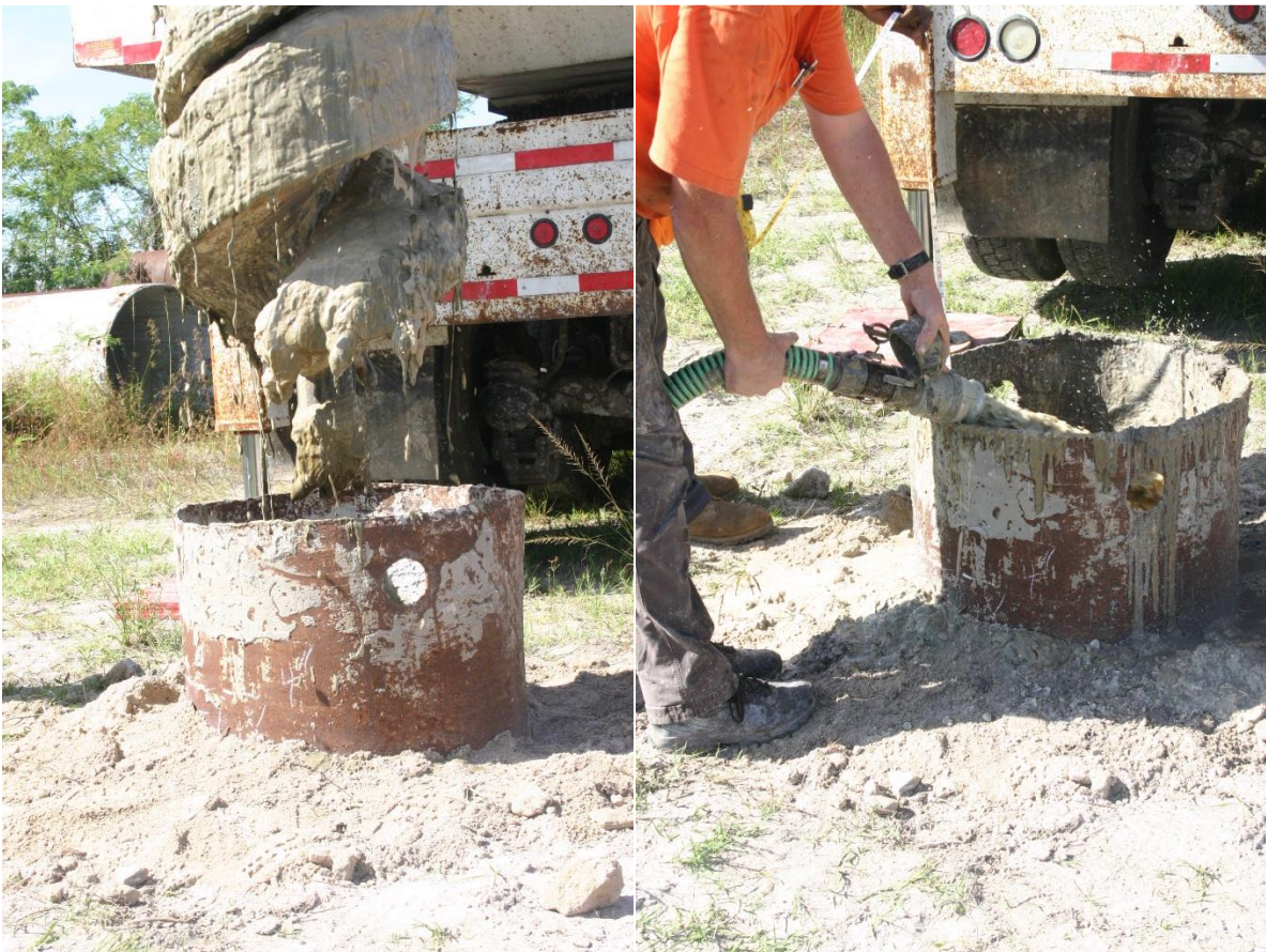
Figure 4.13 Auger extraction (left) and slurry replacement (right) during construction of Shaft B48-40.
