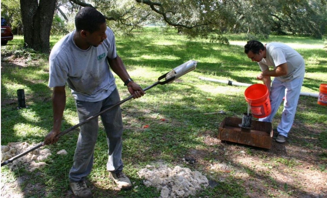
Figure 3.84 Emptying of auger bucket and simultaneous slurry addition to borehole.
