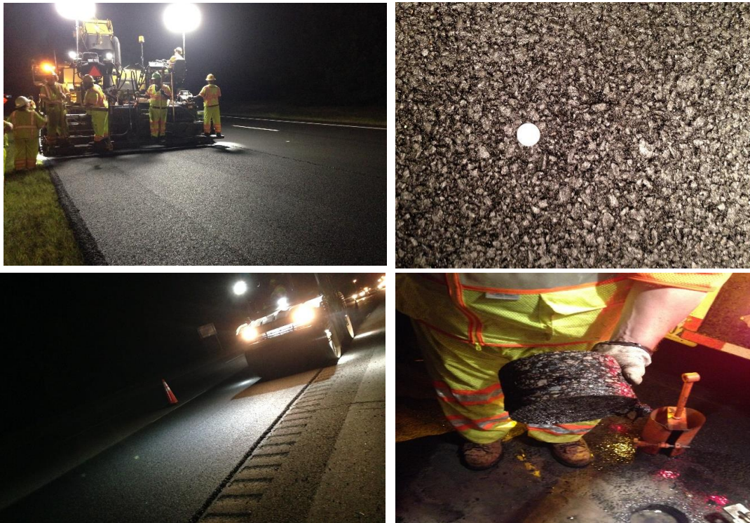
Figure 8. Placement of AR-GGM Mixture
