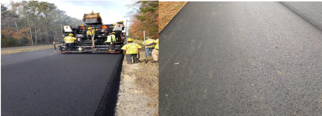
Figure 6. Placement of SM 12.5 (GTR) Mixture. GTR = ground tire rubber.
