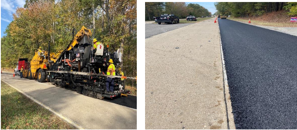
Figure 5. Placement of THMACO Layer. THMACO = thin hot mix asphalt concrete overlay.
