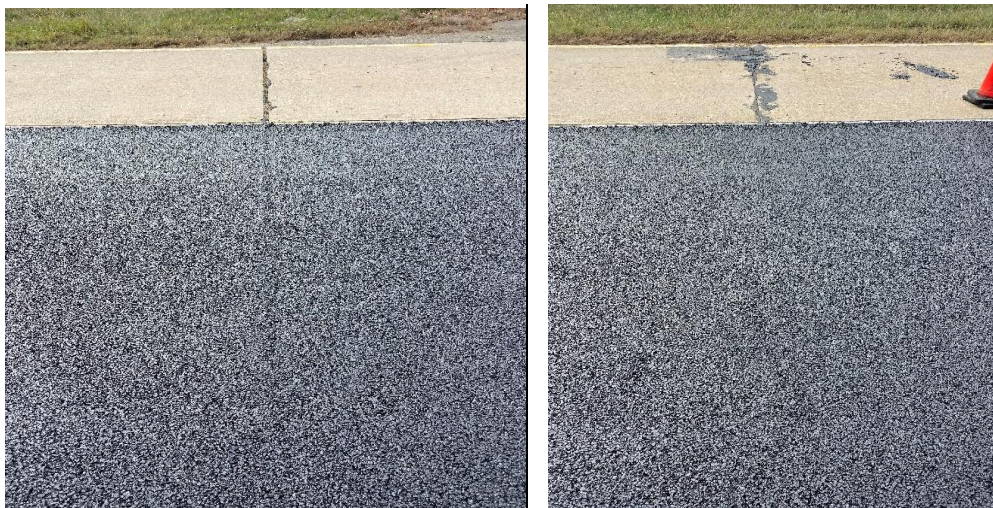
Figure 11. THMACO Layer Showing Shadow of Concrete Pavement Joint. THMACO = thin hot mix asphalt concrete overlay.
