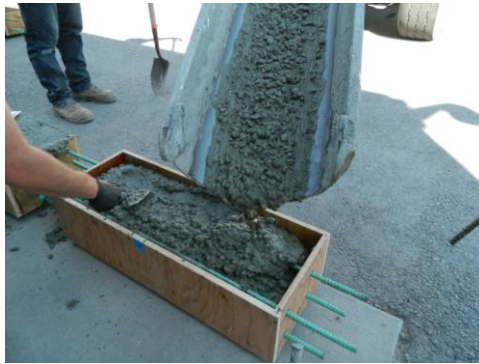
(a) Pouring large beam precast segments
