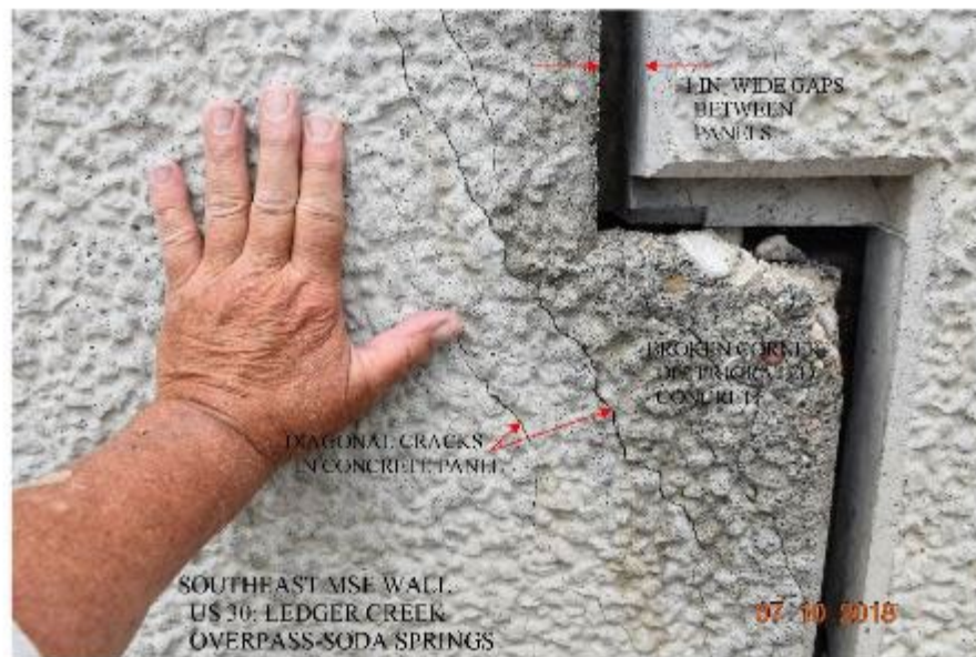
Figure 27. Concrete Deterioration and Diagonal Cracks in MSE Wall at Ledger Creek Bridge
