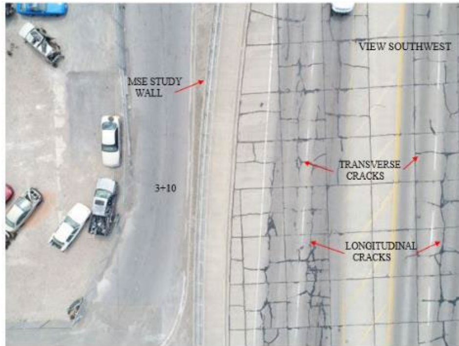
Figure 53. sUAV Photo of Pavement Cracks, Gould Street Overpass, Wall 4
