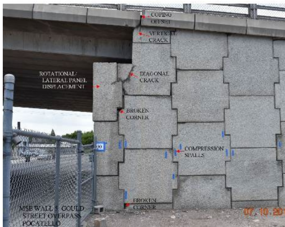
Figure 23. Severe Damage in MSE Wall 5 Beneath West Abutment of E. Gould Street Overpass
