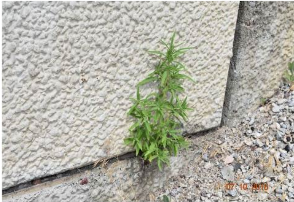
Figure 70. Vegetation Growth, STA 0+41.7, S. Wall, E. Abutment, Ledger Creek Bridge
