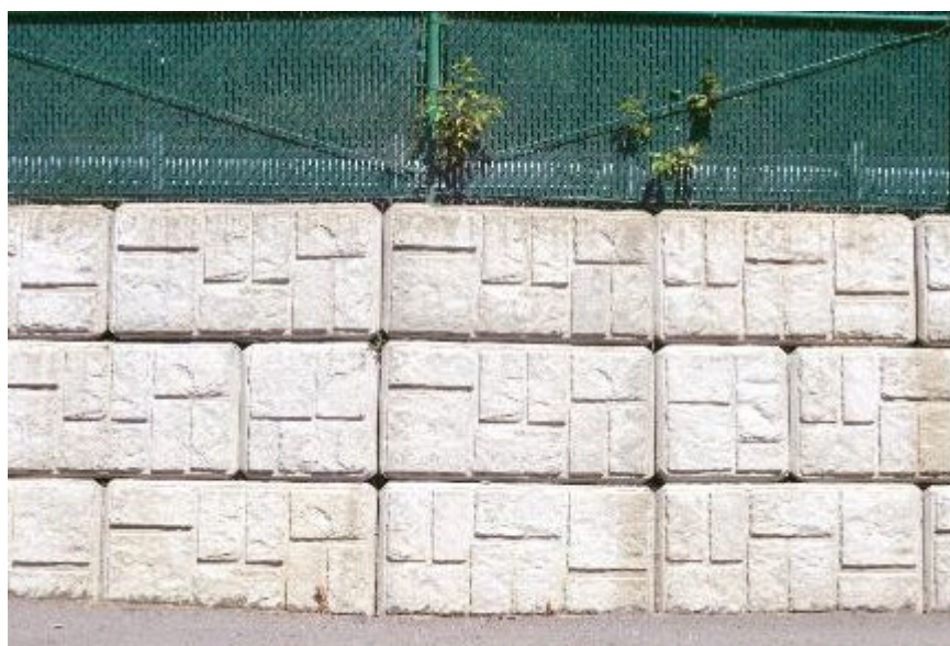
Figure 14. Concrete Block with “Cut-Stone” Finish used for Trestle Creek Wall
