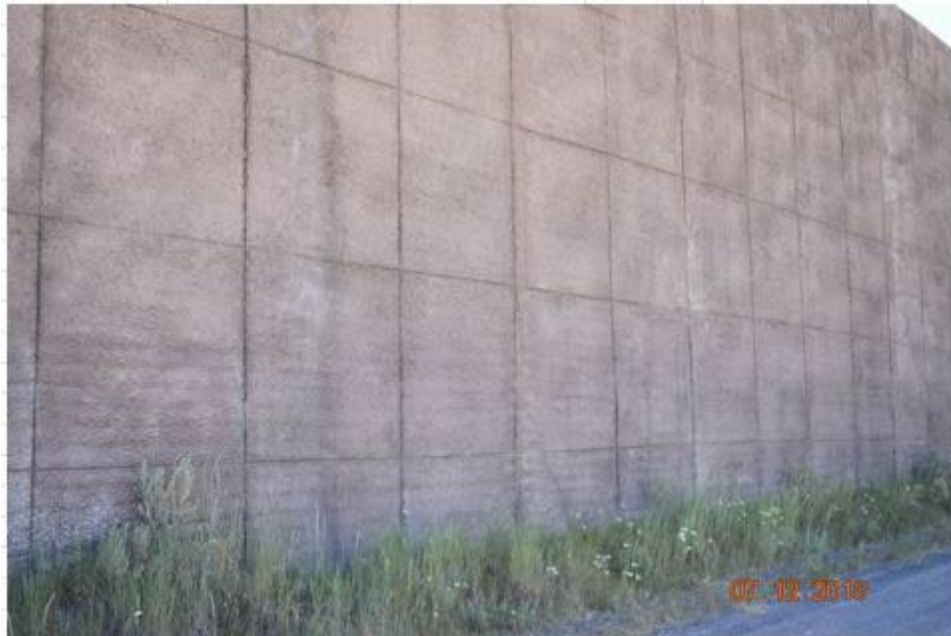
Figure 65. sUAV Photo of Fiber Shotcreted Geofoam Blocks, N. Wall, W. Abutment, Topaz Bridge
