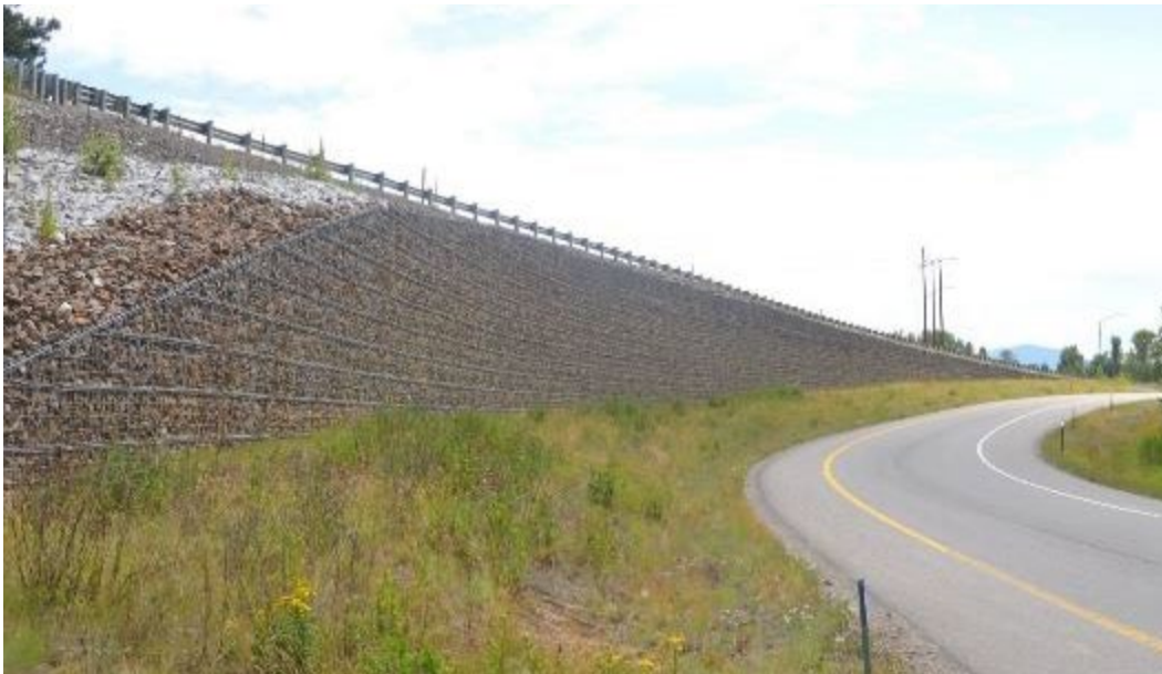
Figure 11. Wire-Gabion MSE Wall at MP 475, SB US-95 in Sandpoint
