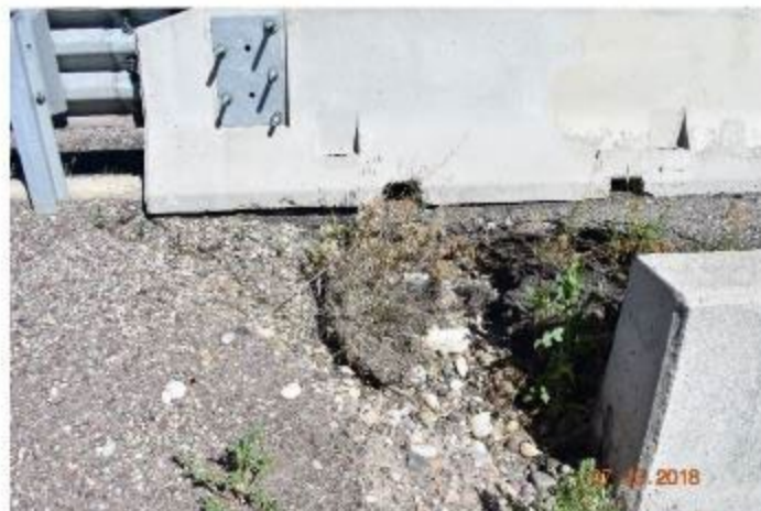
Figure 28. Erosion Along and Behind MSE Wall Coping and Concrete Barrier at US-20, St Leon Exit
