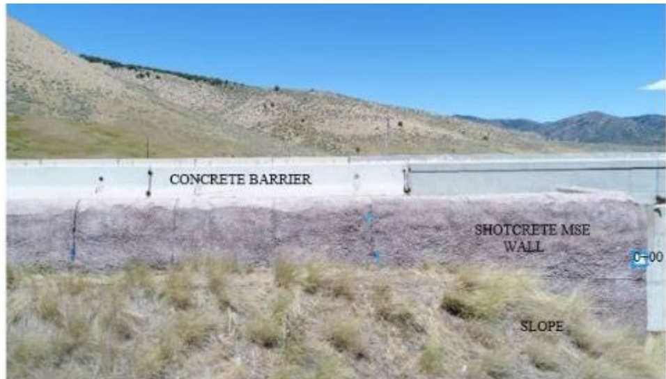
Figure 60. sUAV Photo of South MSE Wall, West Abutment, Topaz Bridge, looking North
