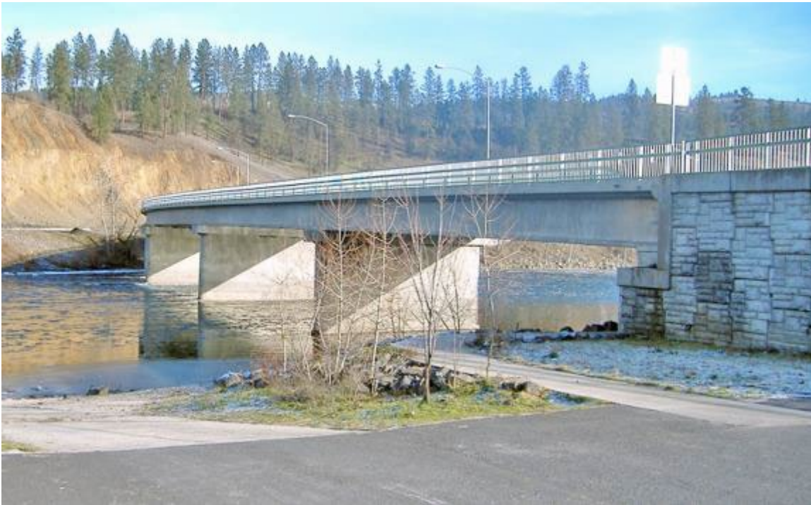
Figure 38. North MSE Wall at Eastern Abutment of Kamiah Bridge, MP 66.69, WB US-12
