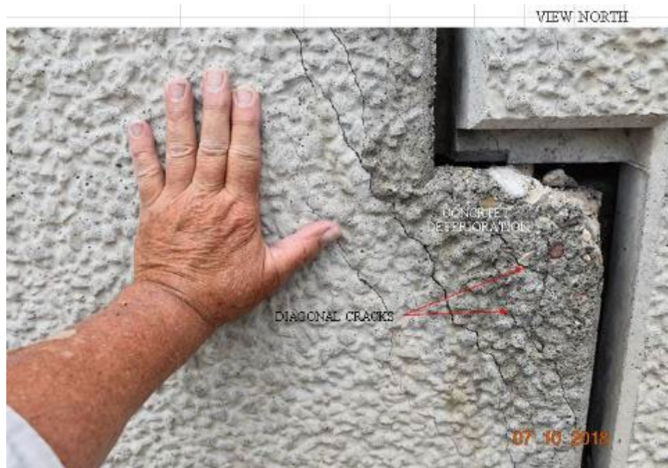
Figure 68. Diag. and Vert. Cracks (HL to 1/16 in) and Concrete Deterioration, Ledger Creek Bridge
