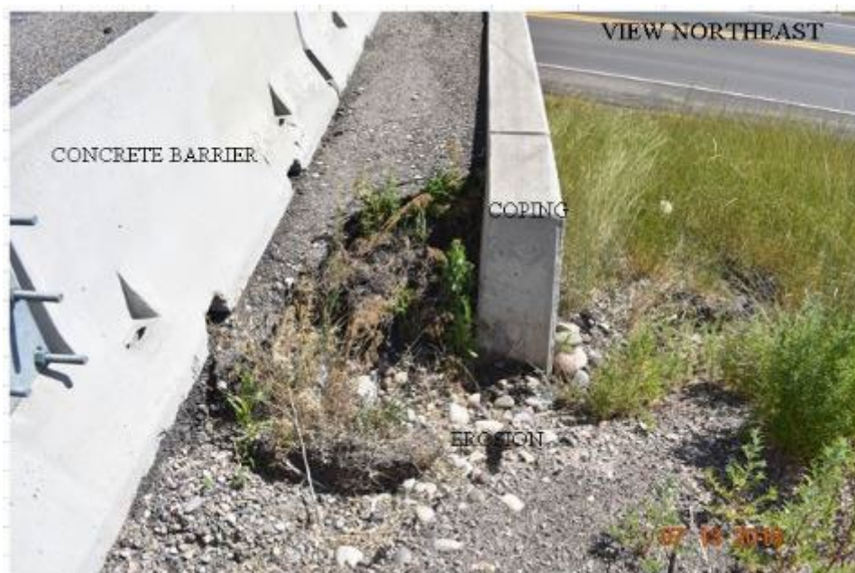
Figure 77. Erosion Channel at Edge of South Wall, West Abutment, US-20, St Leon Exit
