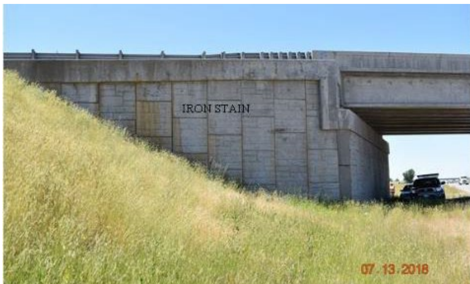
Figure 89. Iron Staining and Coping Cracks, N. MSE Wall, E. Abutment of SH-33 Exit at US-20
