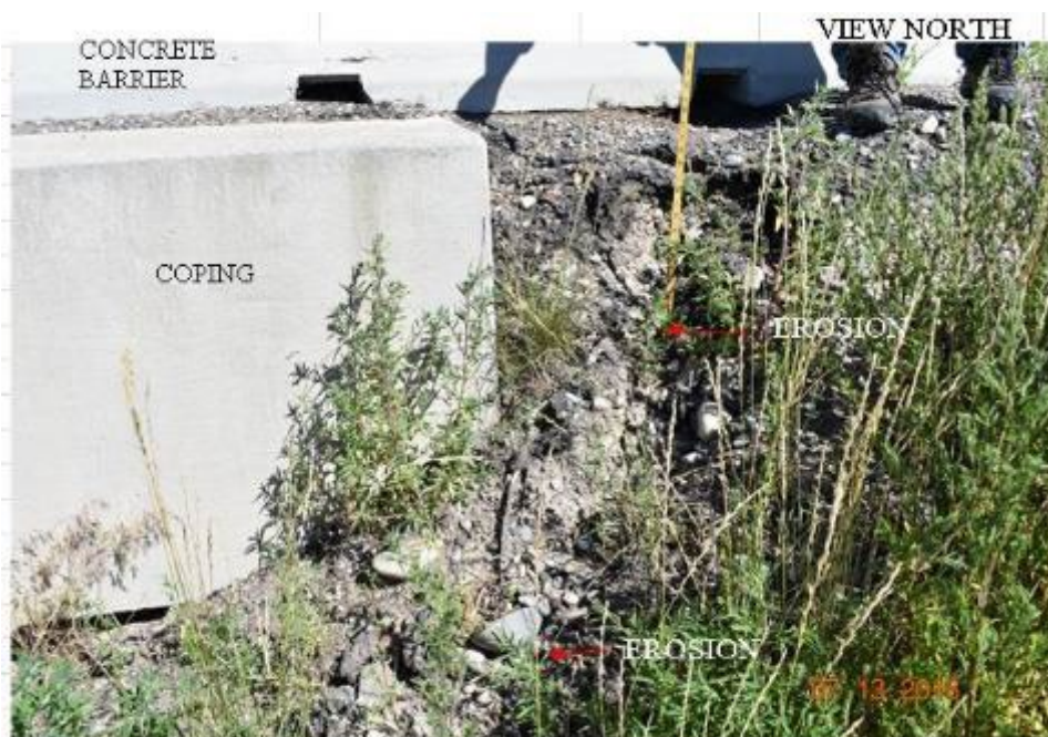
Figure 79. Erosion Channel at Edge of South Wall, West Abutment, US-20, St Leon Exit
