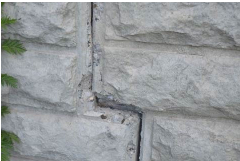
Figure 10. Crushed Panel at L = 40 feet
