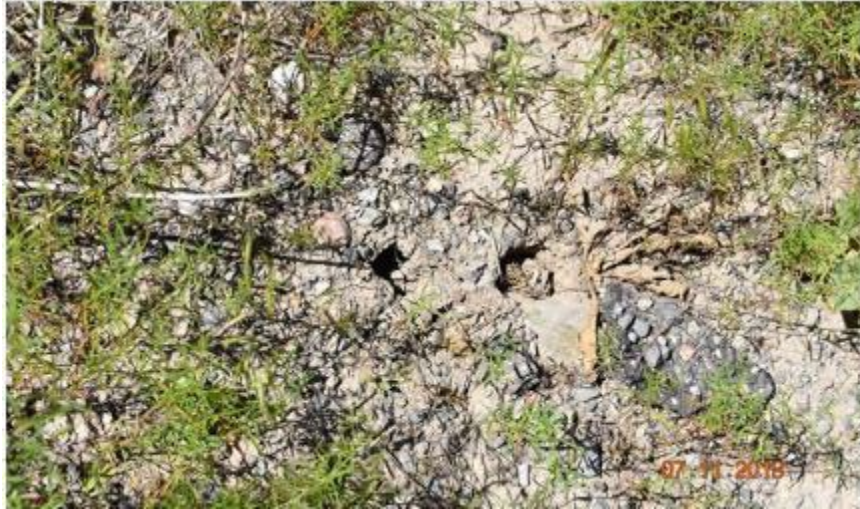
Figure 96. Animal Burrows at STA 2+77,1, South MSE Wall, Bitch Creek Bridge
