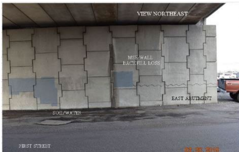
Figure 22. Soil/Water Flow (Piping) from MSE Wall 4 West Abutment Face, E. Gould Street Overpass
