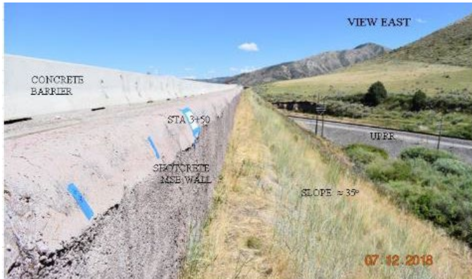
Figure 24. Steel-fiber Reinforced Shotcrete MSE Wall at Topaz Bridge, US-30
