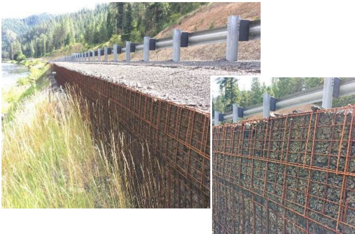
Figure 18. View of Eastern Wall and Corten-steel Gabions from Clearwater Riverbank
