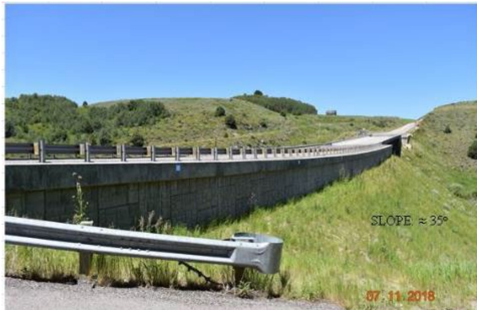
Figure 93. East MSE Wall, South Abutment, Bitch Creek Bridge, SH-32
