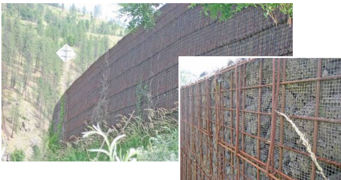
Figure 16. View of Western Wall and Corten-steel Gabions from Clearwater Riverbank
