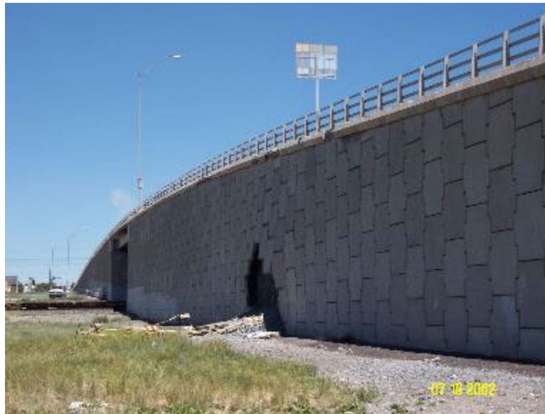
Figure 2. MSE Wall Failure on SH-34, Soda Springs, ID, in July 2002 (3)
