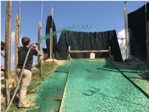
(a) Bottom install
