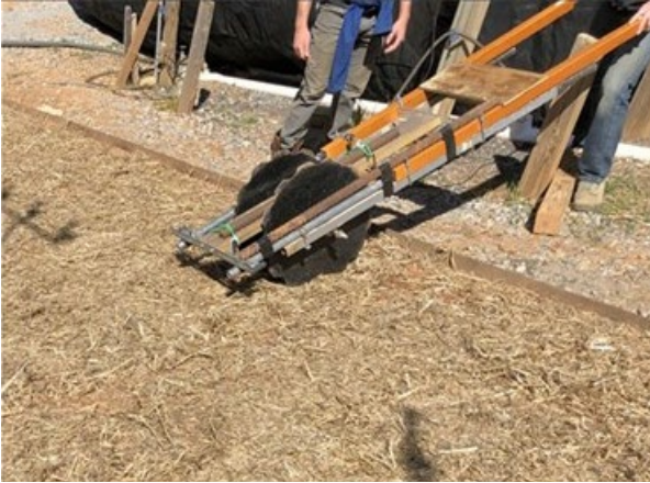
(a) Crimping perpendicular to slope
