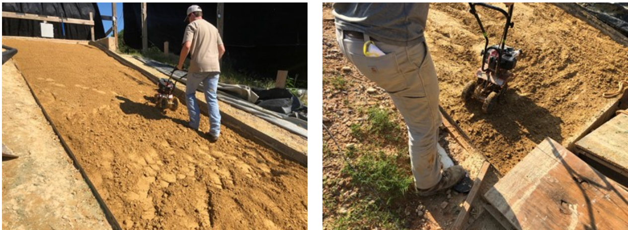
FIGURE 3.6: Tilling Test Slope
