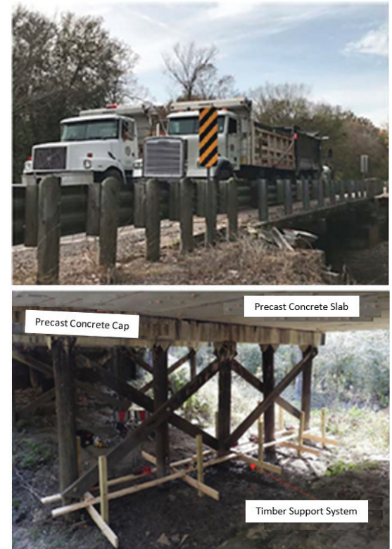
Top: Proof load testing of a bridge foundation; Bottom: Instrumented piles at a Louisiana bridge
