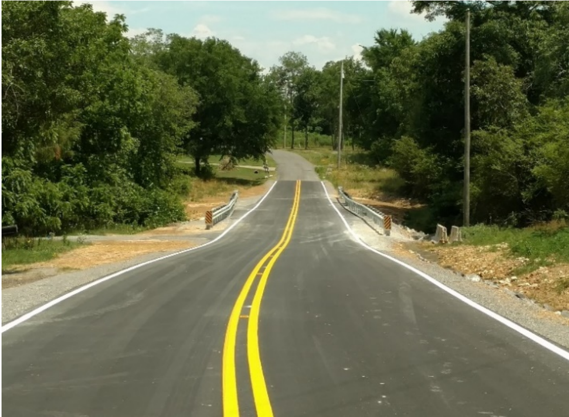
Figure 22 The completed GRS-IBS over Turkey Creek in Marshall County, AL.
