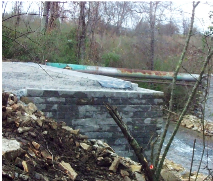
Figure 19 The finished GRS abutment prior to placement of the bridge beams.
