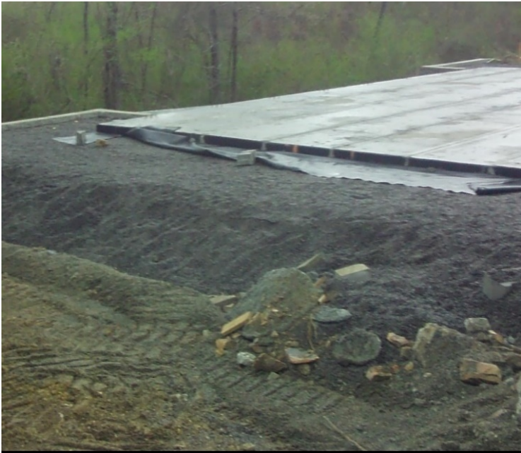
Figure 21 Placed bridge beams and the integrated approach.
