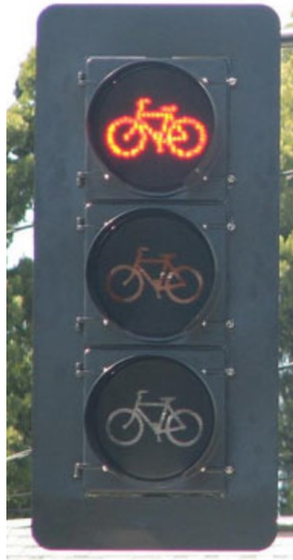
Figure 2.4: Example of a bicycle signal with bicycle symbol in signal face (NACTO, 2014)
