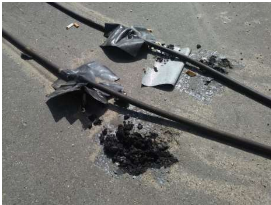
Figure 3 Pneumatic tube dislocation in asphalt, Tulane Avenue, June 2017
