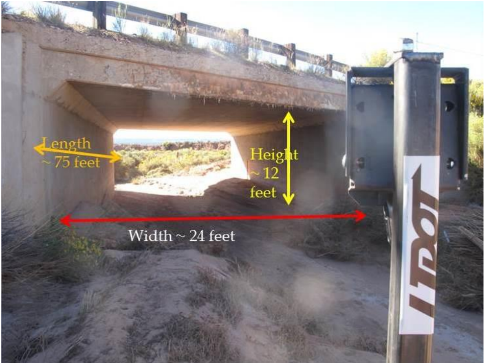
US 89 MP 48.2 Seaman Wash Existing Concrete Box Culvert.
