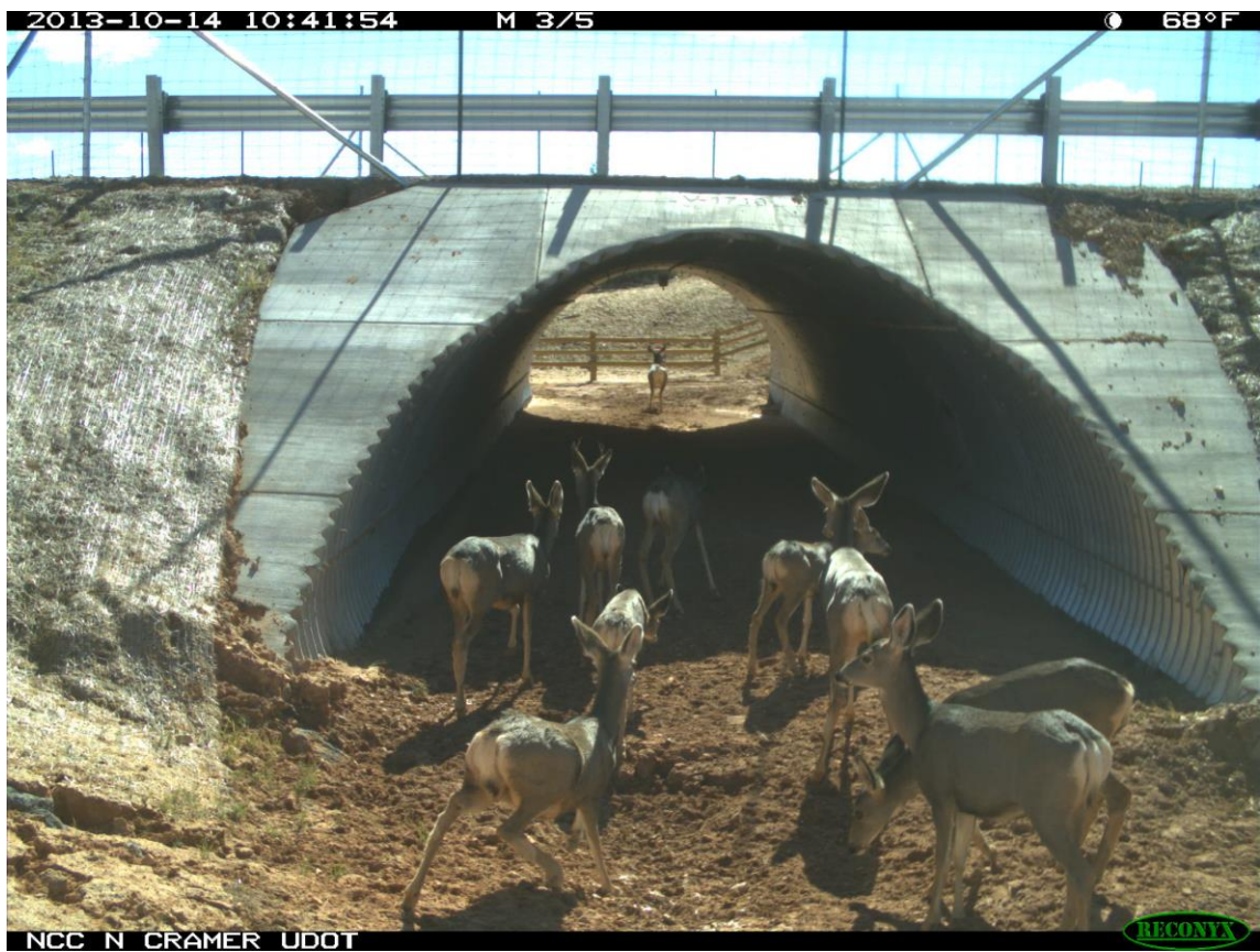
Mule Deer Used the Center New Culvert During the First Fall Migration, 2013.
