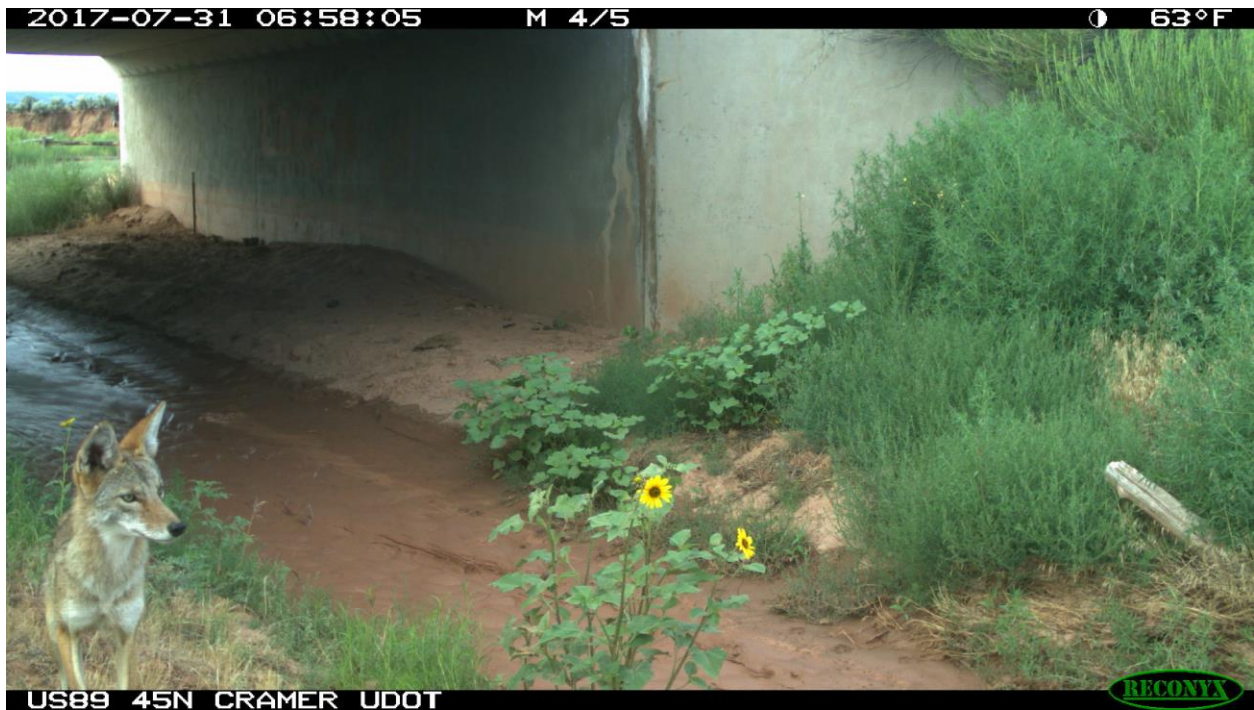
Coyote at Petrified Culvert, July 2017.
