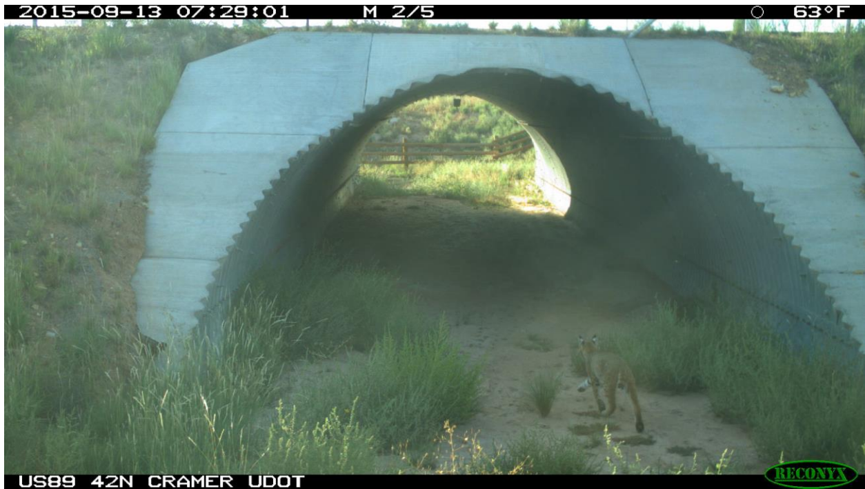
Bobcat Used Center New Culvert MP 42.5 From North.
