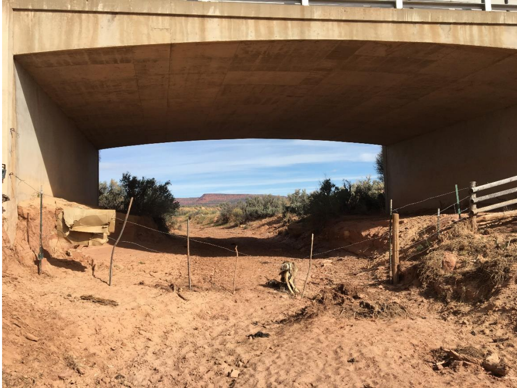
Figure 27. Wire Fence for Domestic Cattle Attached to the South End of the Buckskin Structure in 2018 with Mule Deer Carcass Tangled In Barbed Wire.
