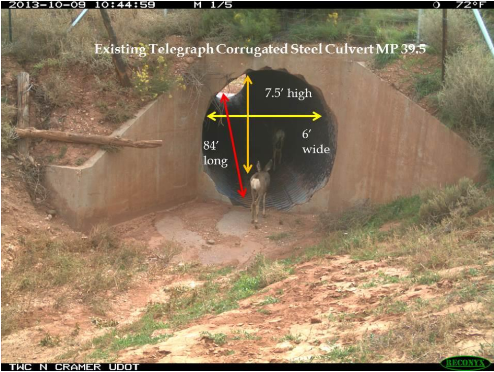
US 89 MP 39.5 Telegraph Wash Existing Corrugated Steel Culvert.
