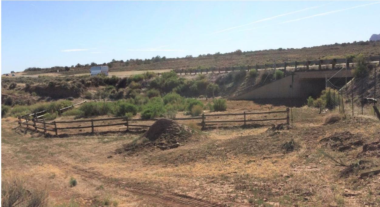
Figure 28. Wildlife Friendly Fence Installed by UDWR Wildlife Biologists on South Side of Petrified Culvert.
