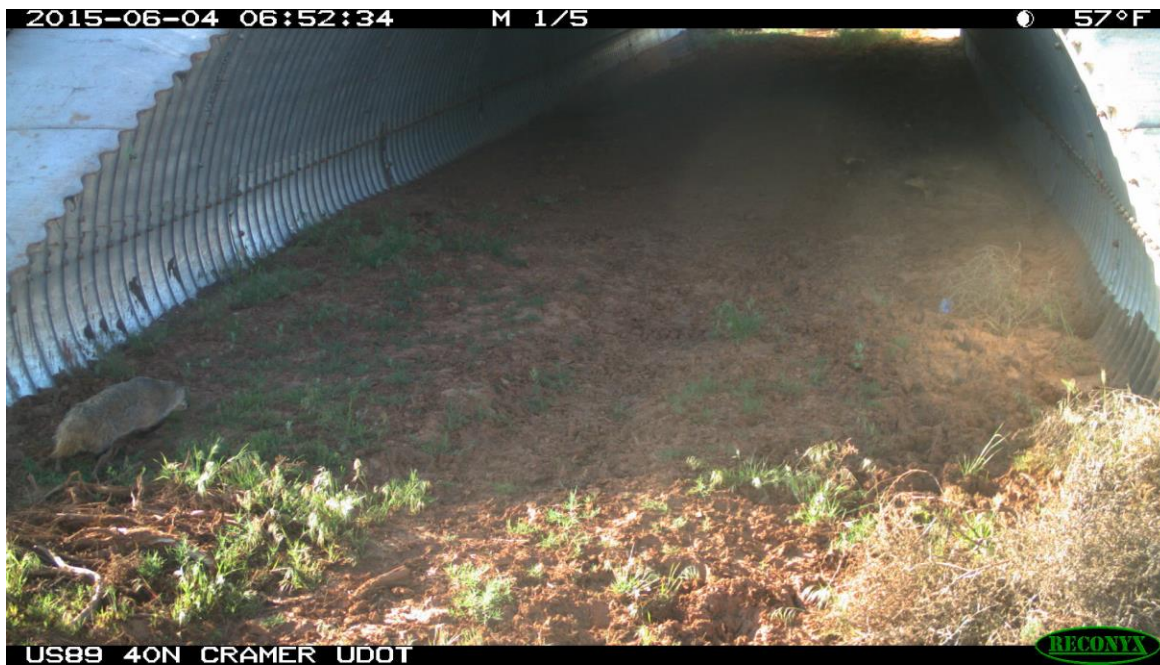
East New Culvert MP 40.5 Badger Used Culvert from North.
