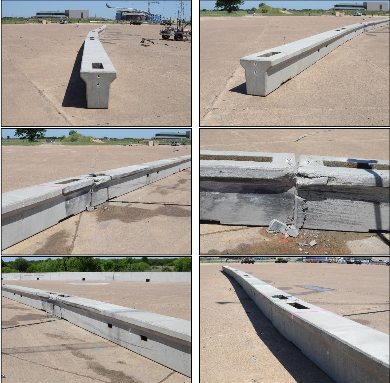
Figure 7.3. TL-3 Low-Profile Barrier after Test No. 469688-1-2.
