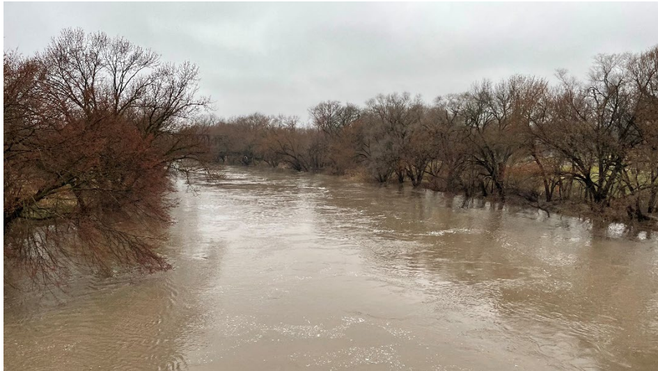
Figure 3.10: Railroad bridge upstream of the Beatrice bridge.
