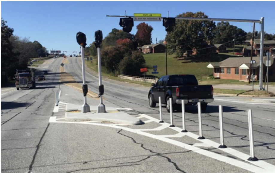
Figure 6. Construction of new Pedestrian Hybrid Beacon in Macon-Bibb County. 24
