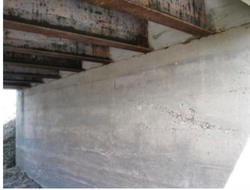
Figure 0.1 Representative steel girder bridge
